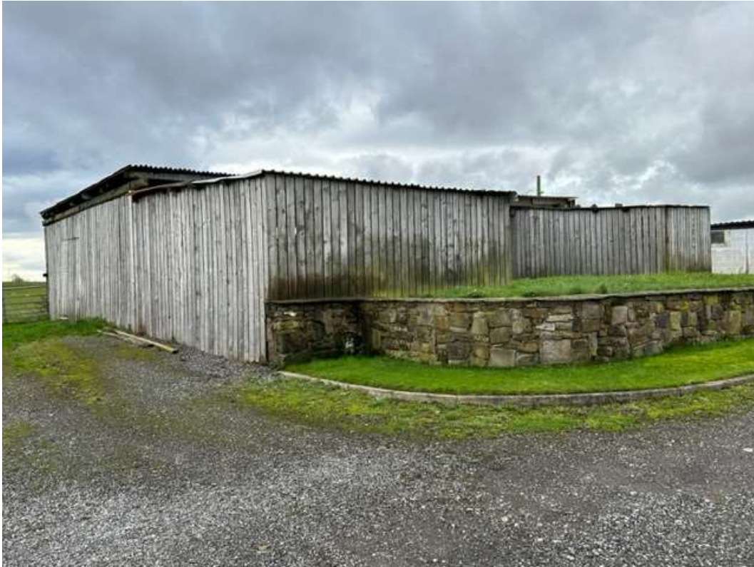
Image 3 – Existing agricultural building
