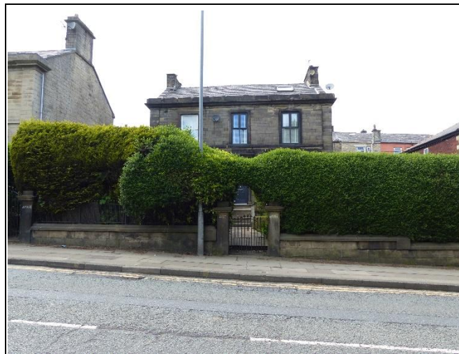
Hest Bank, Bolton Street
