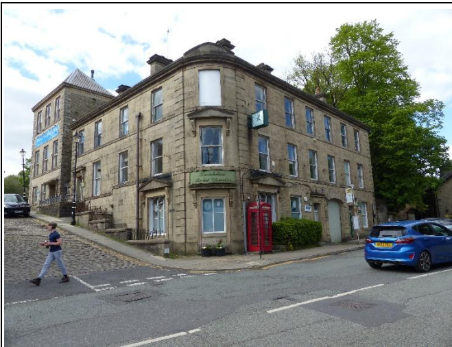
Council Chambers and K6 Kiosk, Ramsbottom Lane
