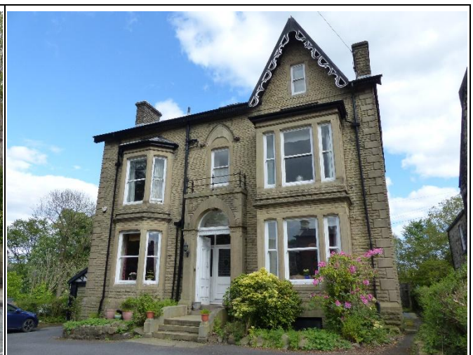
Hope House, Bolton Street
