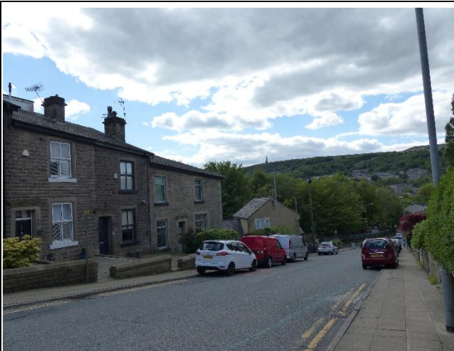
Looking West Towards Peel Monument from Peel Brow
