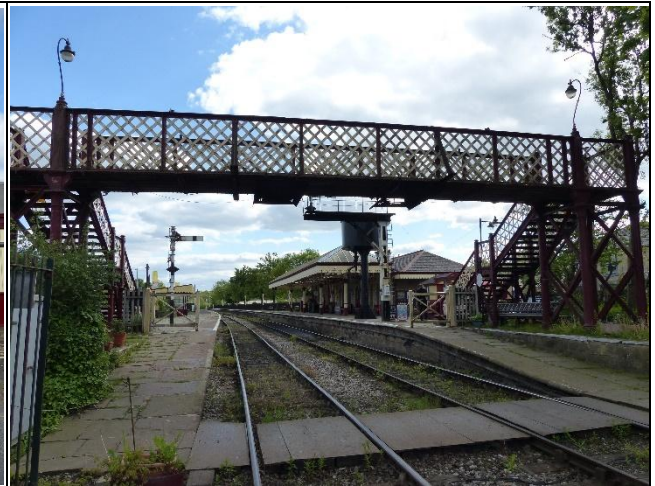
Cast Iron Footbridge Over the Railway
