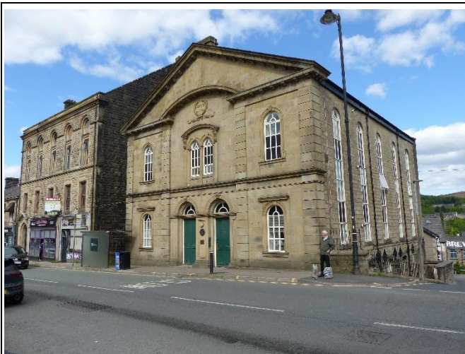
Ramsbottom Co-operative Hall and Adjacent 55 Bolton Street
