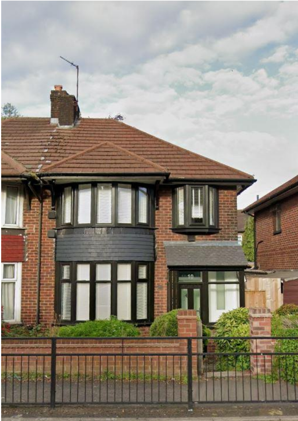
Fig 1. Front Elevation, (Google Street View, Accessed March 2026)
