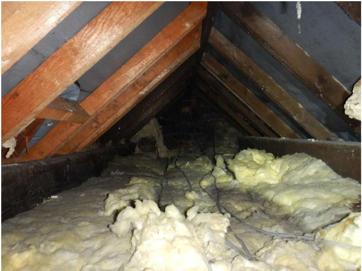
Photo 19. North facing in western roof space
