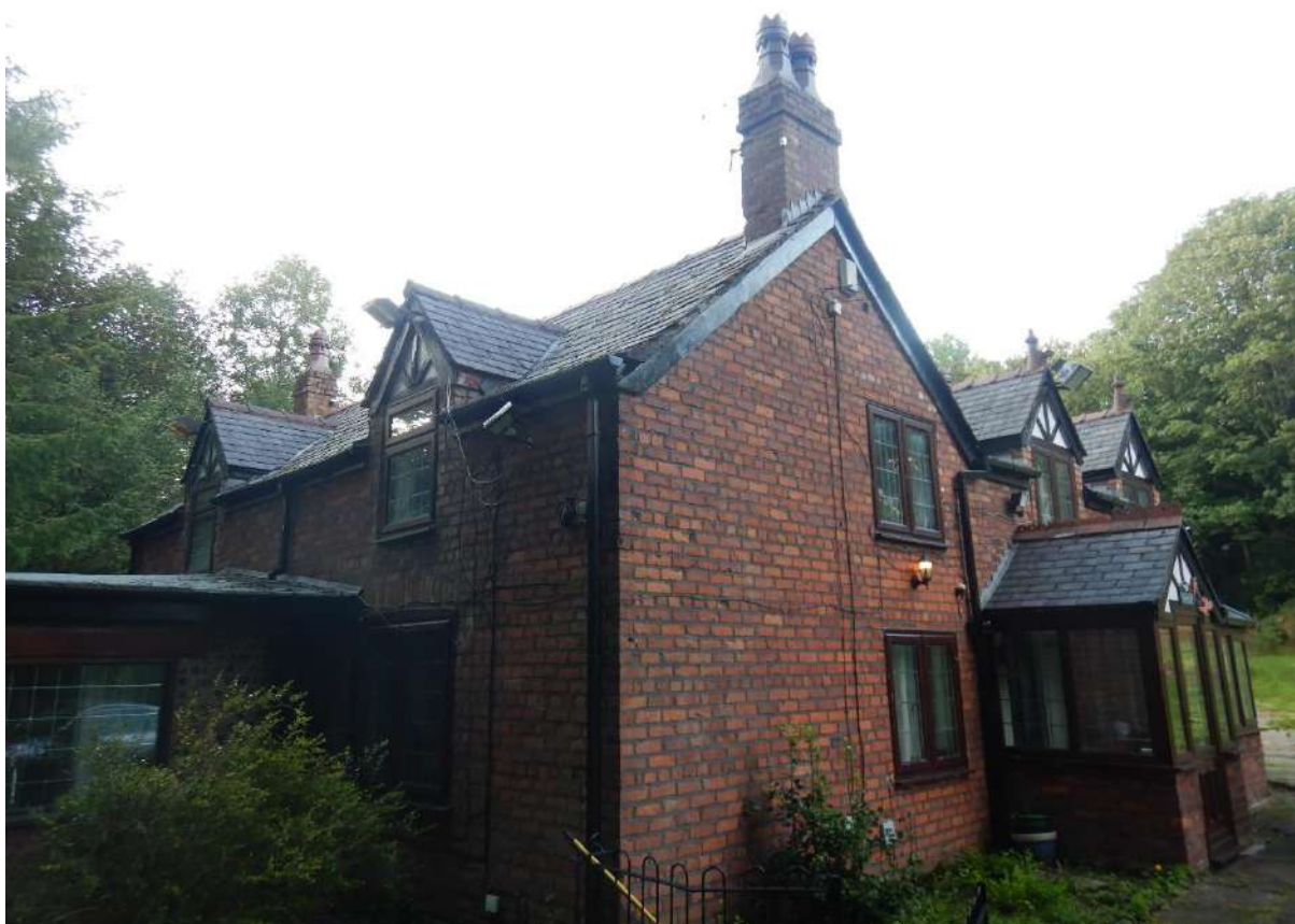
Photo 6. Southwest aspect (left) and southeast front aspect (right)
