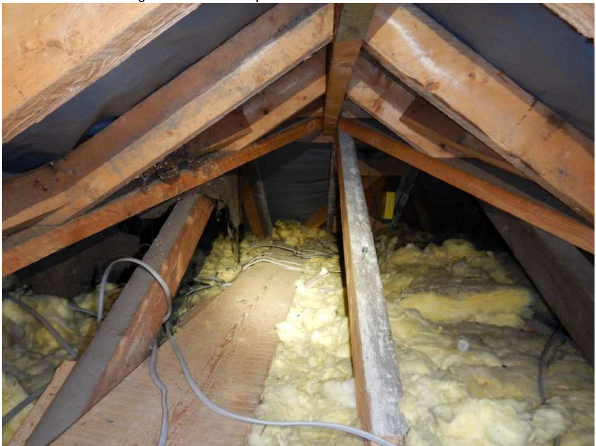
Photo 20. Showing eastern loft space. Note plastic lining.
