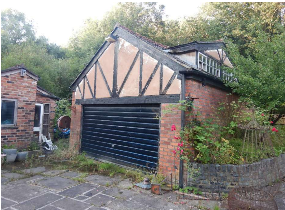
Photo 12. Garage outbuilding showing southwest facing gable end.
