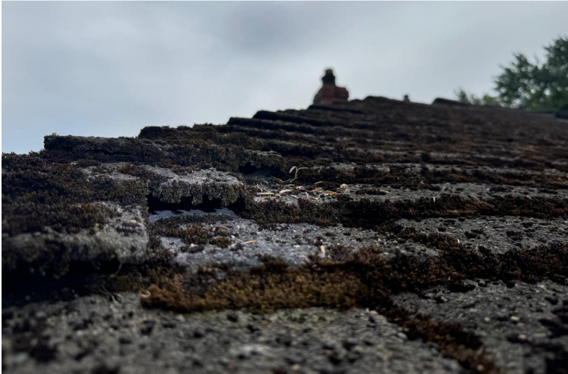
4. No gaps or missing roof tiles
