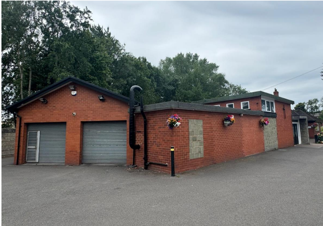
1. Front of building
