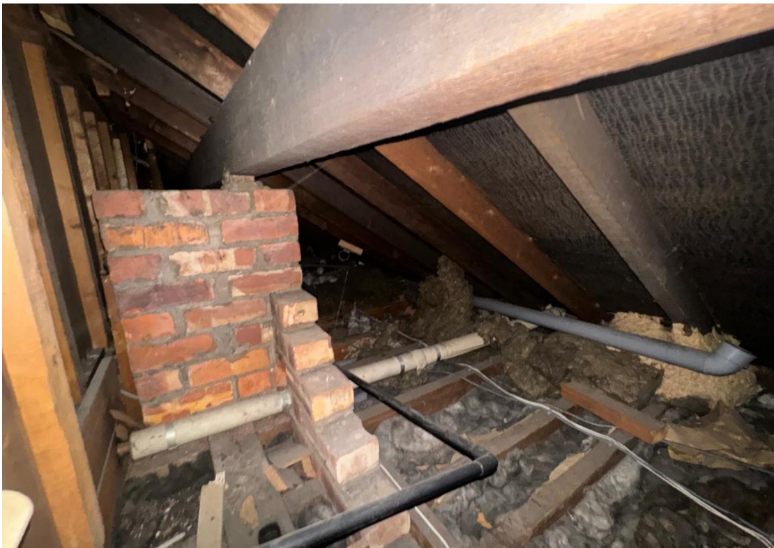
5. Exposed rafters lined with bitumen roofing felt
