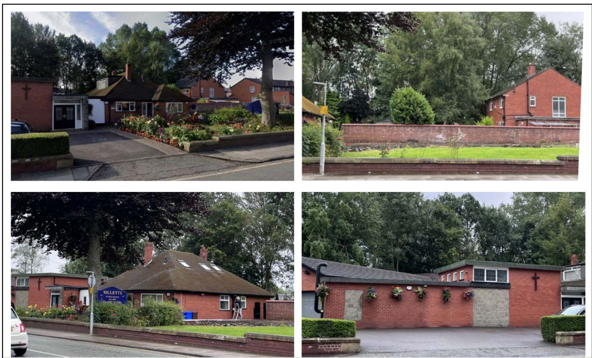
Images of the existing buildings (Workshop Design Studio Ltd Design & Access Statement)
