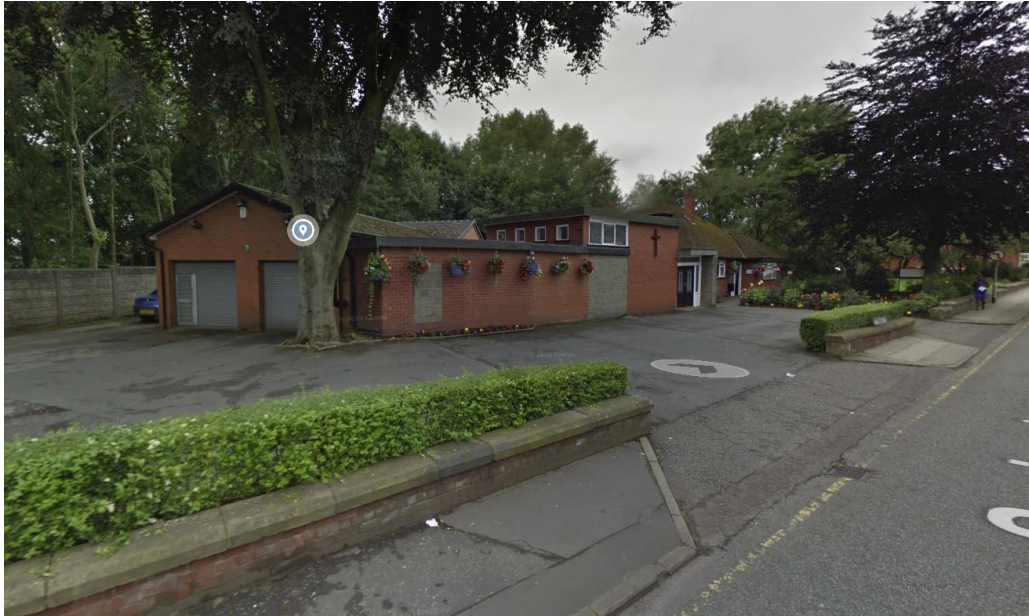
Photo 1 – Existing Buildings and Accesses
