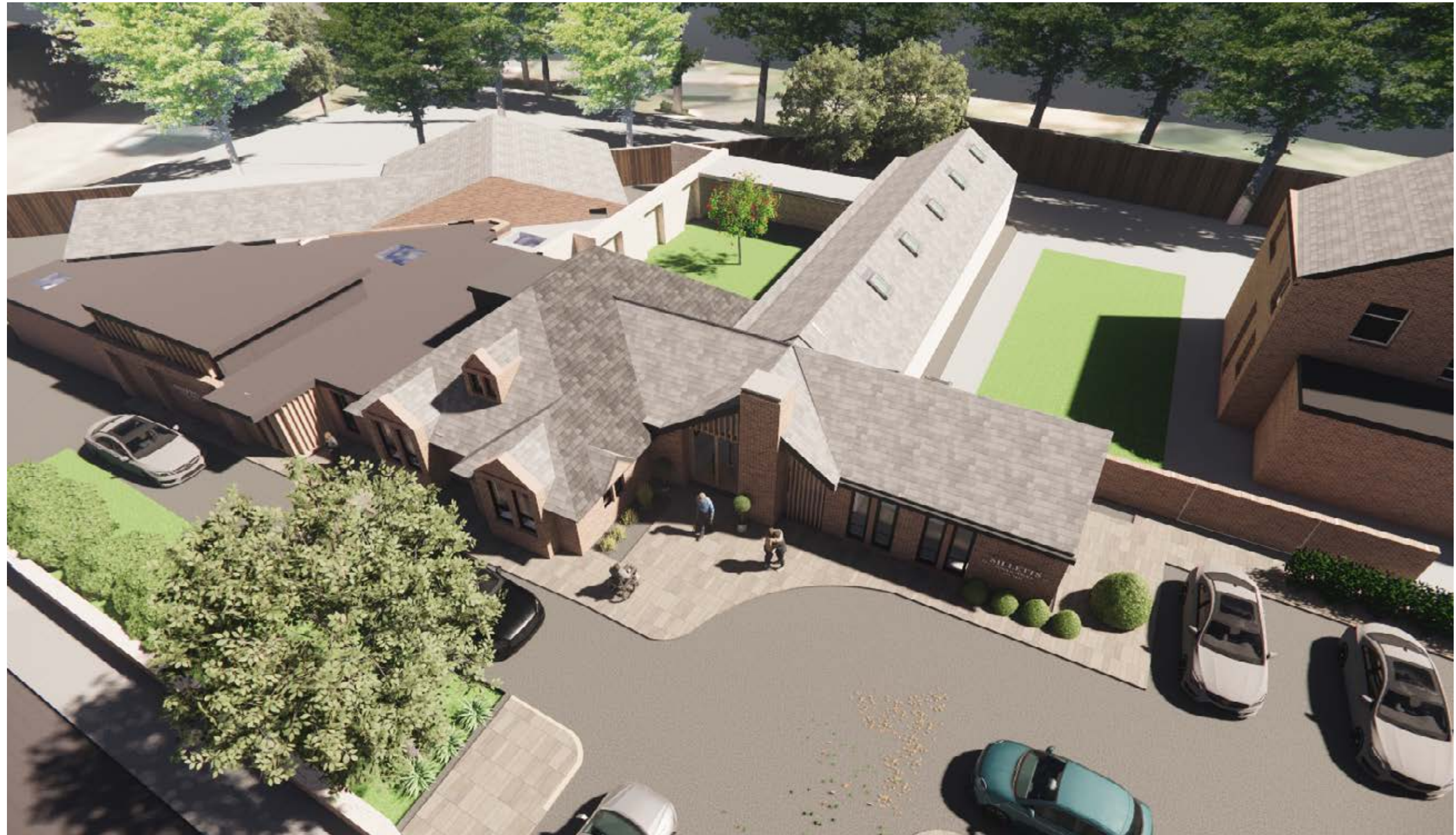
6.5 Front elevation - Aerial view
