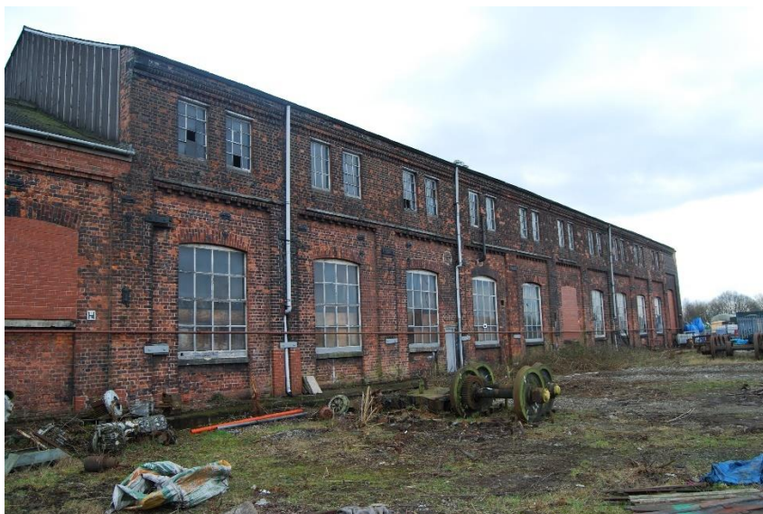
The original 1850s brickwork façade to the west side of the building is largely intact with large numbers of C19th window frames insitu.
