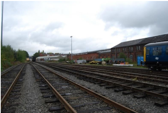
West side of historic 1857 locomotive works/carriage shed building – view north towards Baron Street with 1988 ELR carriage & waggon shed in the background.
