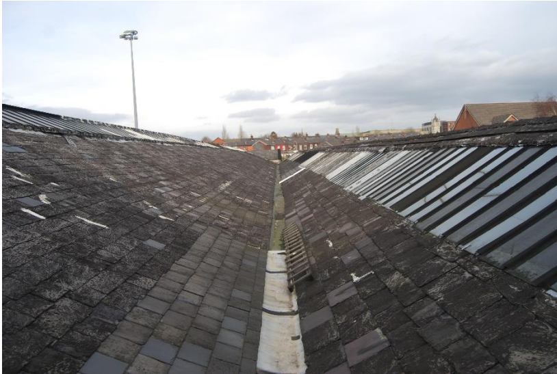
General condition of roof, valley gutter and roof lights.
