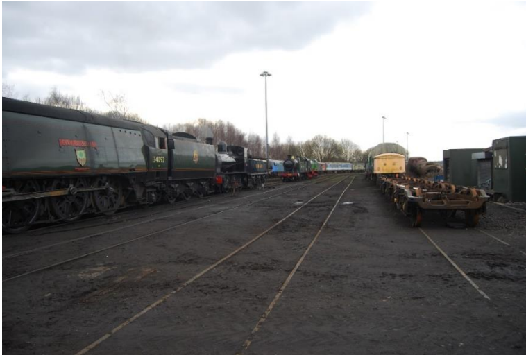
View south from end of the 1855/57 locomotive works/carriage shed building
