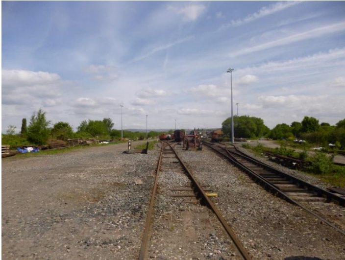
View north from southern end of the site – site for proposed carriage shed building
