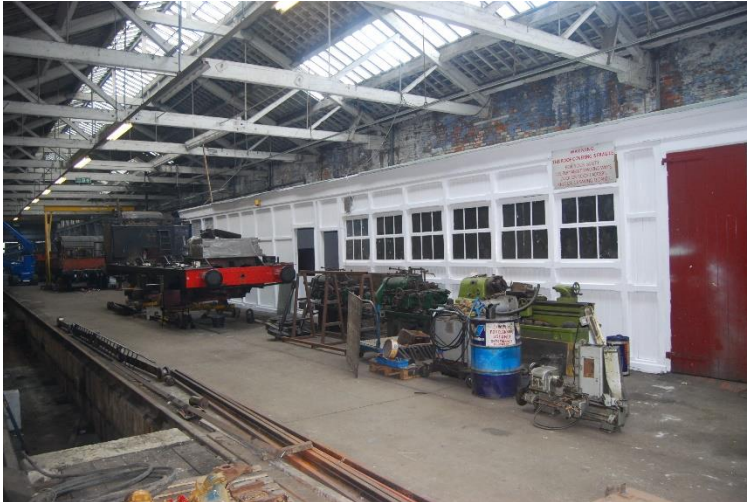
L&YR timber 'platform' buildings though to have been installed in 1915 as part of the conversion of the building into an electric car shop in 1915.
