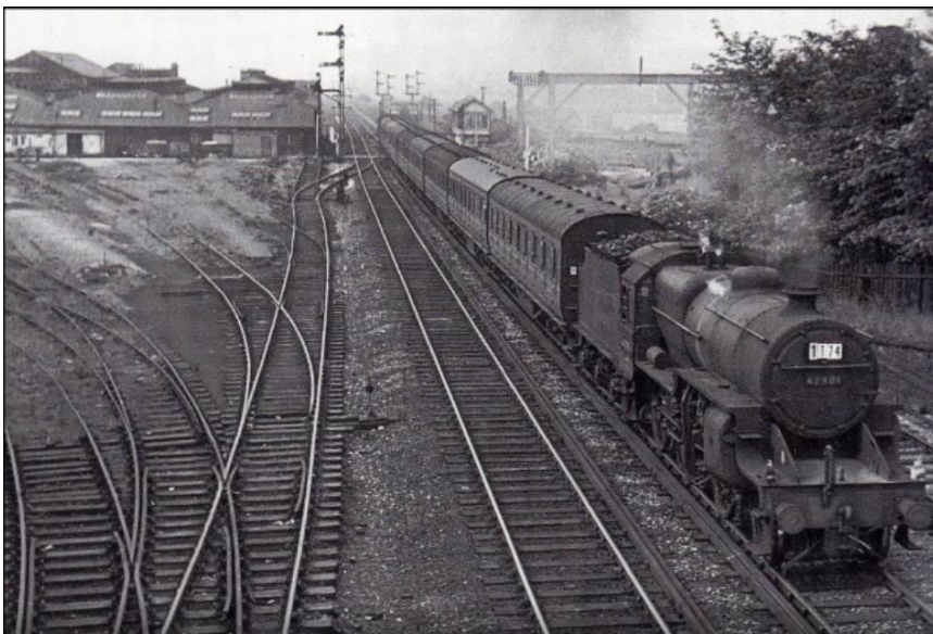
1960s view looking south towards the Buckley Wells depot.
