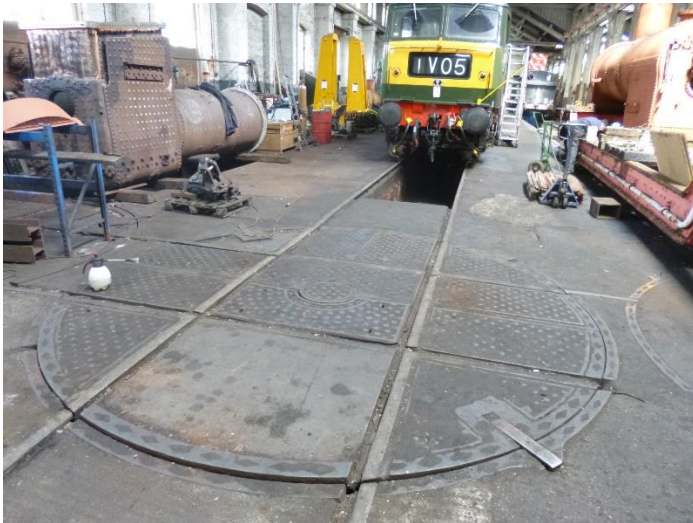
Internal wagon turntable thought to date from the 1850s.
