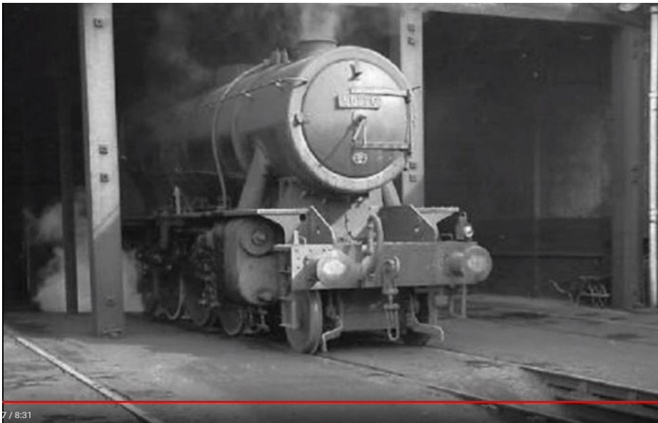
Close up view of the open-end of the engine shed with details of the timber frame – timber columns and lintel.
