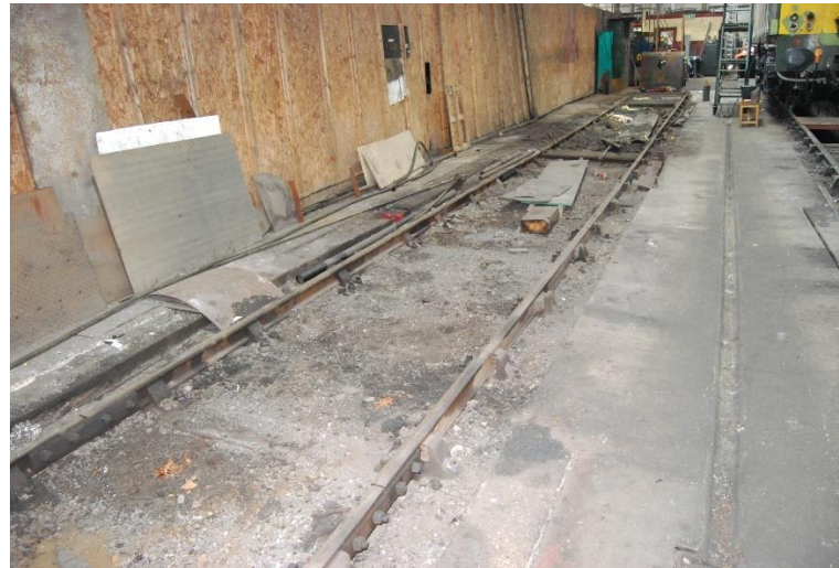
Surviving sections of C19th L&YR cast iron rails
