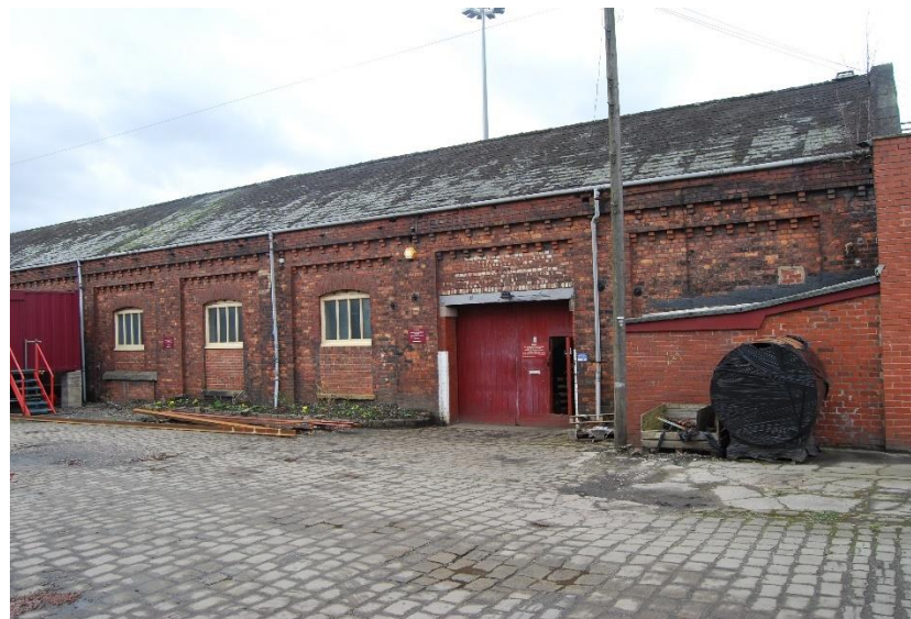
The original 1870s brickwork façade to the east side of the building is also largely intact but, also showing clear evidence of C20th interventions.
