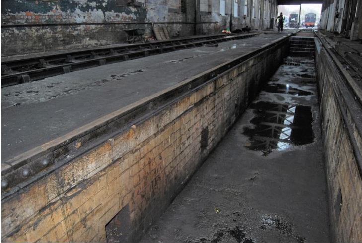
C19th inspection pit(s) at southern end of the building
