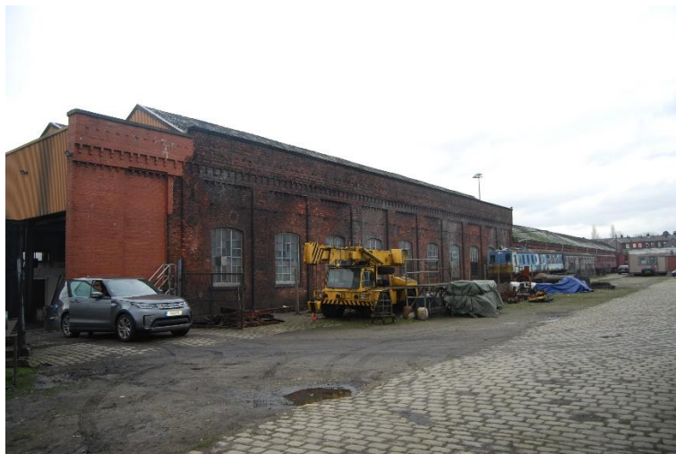
East side of historic 1857 locomotive works/carriage shed building (the façade dating from the 1870's) – view north towards Baron Street with temporary building in background.
