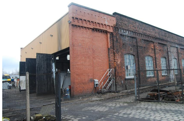
Reconstructed southern end of 1855/57 locomotive works/carriage shed building resulting from demolition of southern end of the building in 1974 – former internal inspection pits in foreground (photo on the left).
