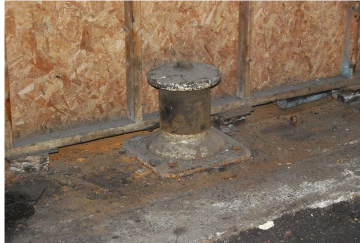
Electric capstan installed as part of the conversion of the building to an electric car shop in 1915.
