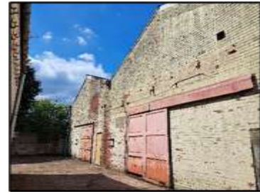
South elevation of unit 9 and 9c
