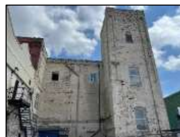
West elevation of unit 5 and tower
