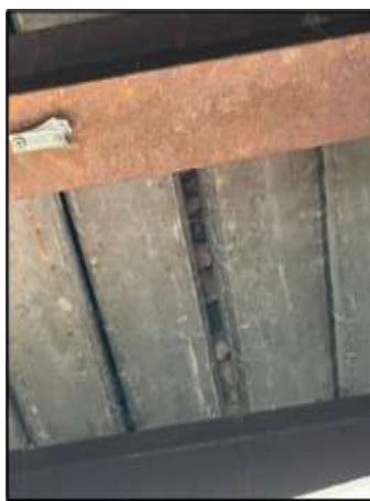
Interior roof void of the office block
