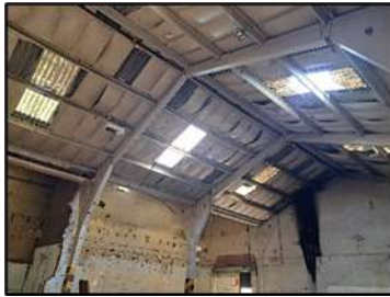
Roof of interior of unit 9
