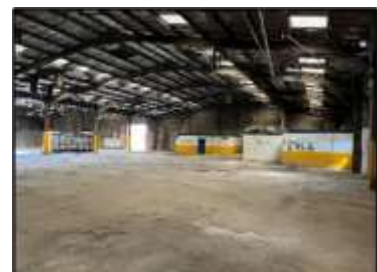
Interior of unit 10
