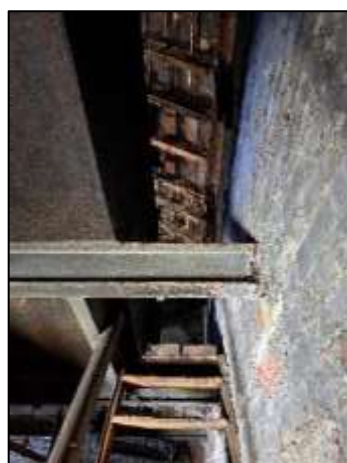
Interior roof void of the tower
