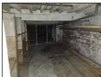
Interior of the cellar below units 4a-4b
