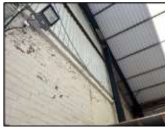
Interior of unit 11
