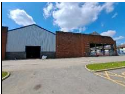
Units 1d and 1e east elevation
