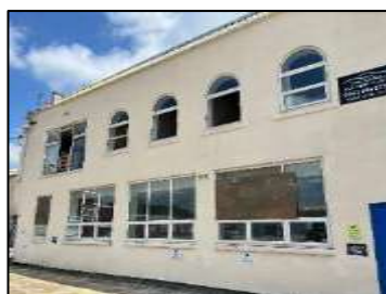
West elevation of unit 4c
