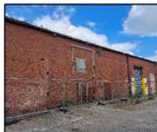
South elevation of unit 10
