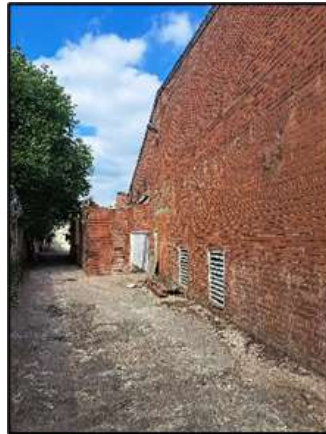
West elevation of unit 10
