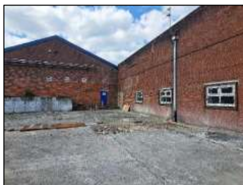
South elevation of unit 2a
