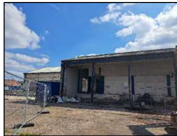
North elevation open extension of unit 8
