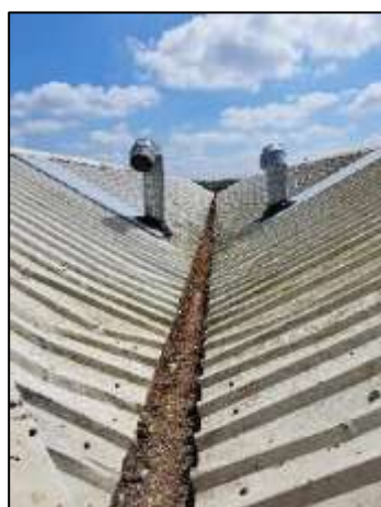
Exterior roof of unit 5
