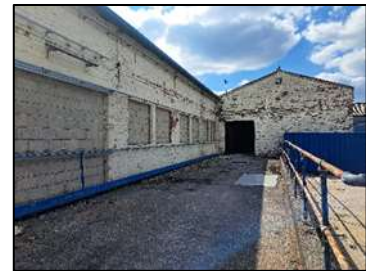
North elevation of unit 8
