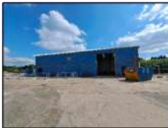
North elevation of unit 11
