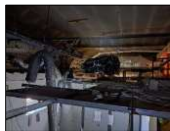
Interior roof void of unit 5
