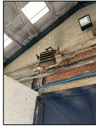
Interior of Unit 12
