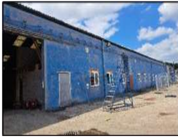
East elevation of unit 9
