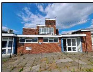
South elevation of office blocks
