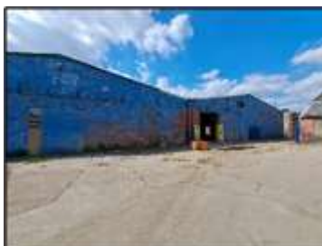
East elevation of unit 10
