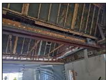
Interior roof void unit 4c
