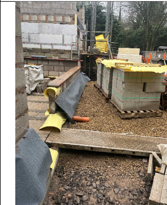
Photo 3. Front of Plots 1-3, facing north.
