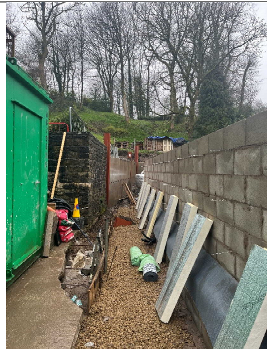
Photo 2. Southern site boundary showing old and new retaining wall, facing west.
