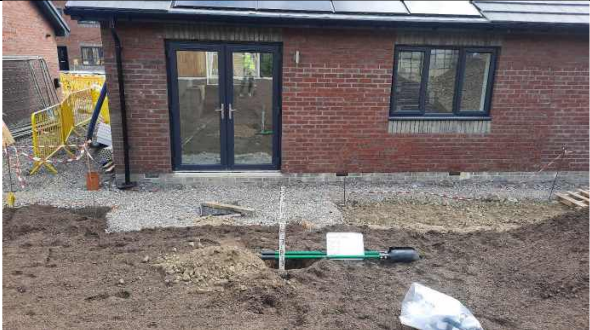
Photo 1 – Plot 2 depth validation to 0.6m.
