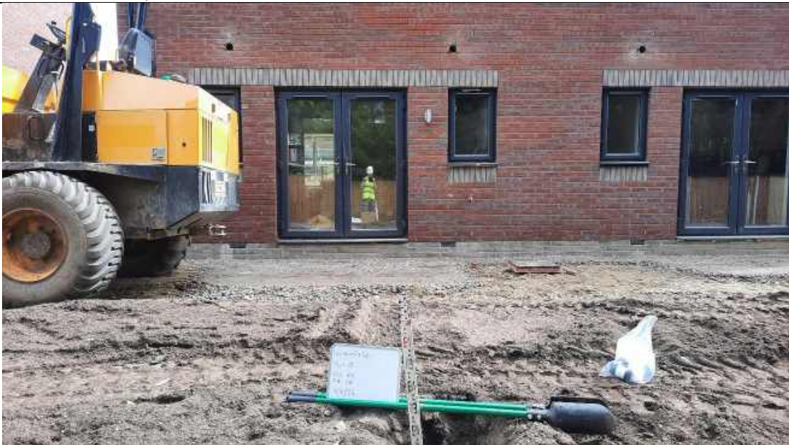
Photo 24 - Plot 10 depth validation to 0.6m.
