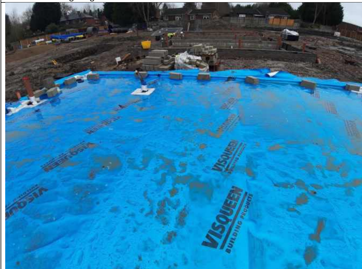
Plate 70: Showing the general condition of the membrane on Plots 21-22
