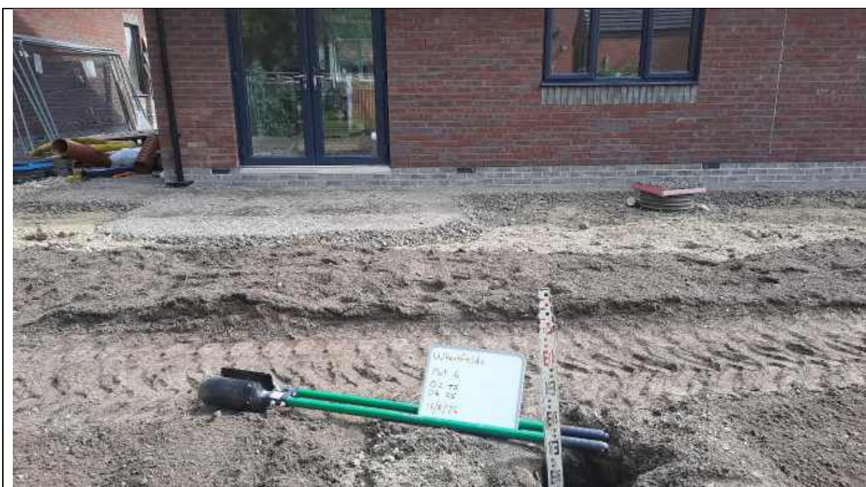
Photo 13 – Plot 6 depth validation to 0.6m.
