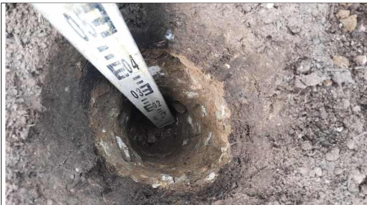
Photo 46 - Plot 22 depth validation to 0.6m.
