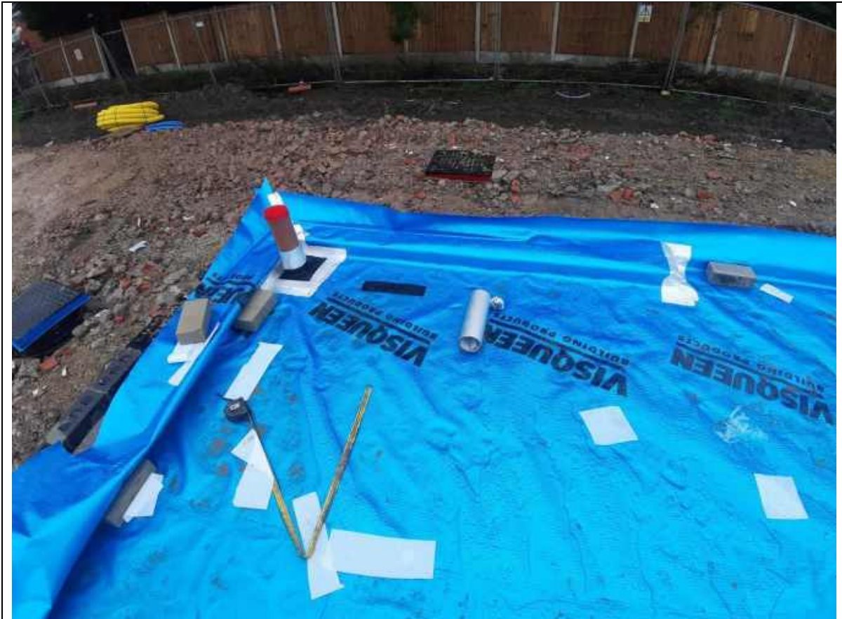
Plate 38: Showing the general condition of the membrane on Plots 11-12
