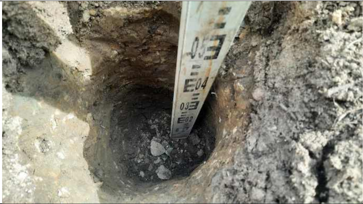
Photo 23 - Plot 9 depth validation to 0.6m.
