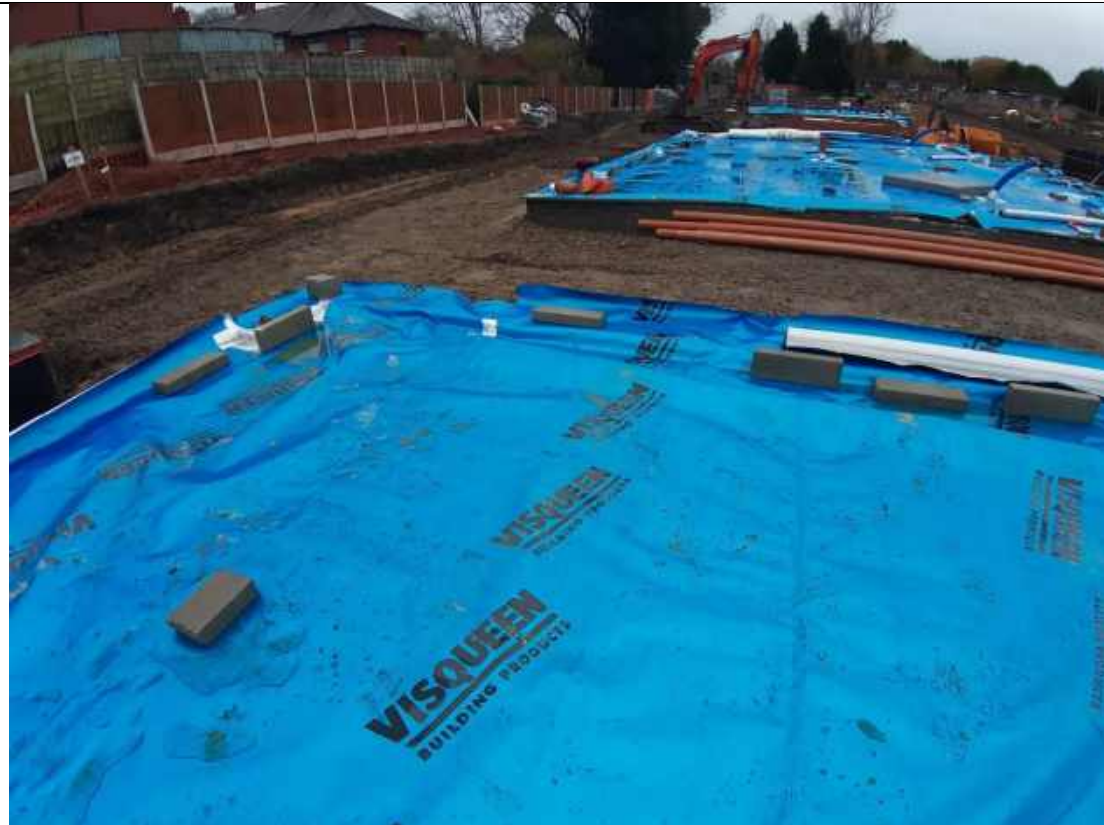
Plate 6: Showing the general condition of the membrane on plot 1-2
