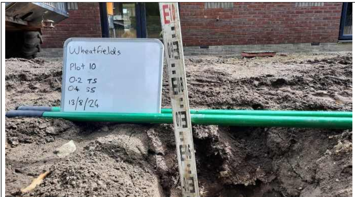
Photo 25 - Plot 10 depth validation to 0.6m.
