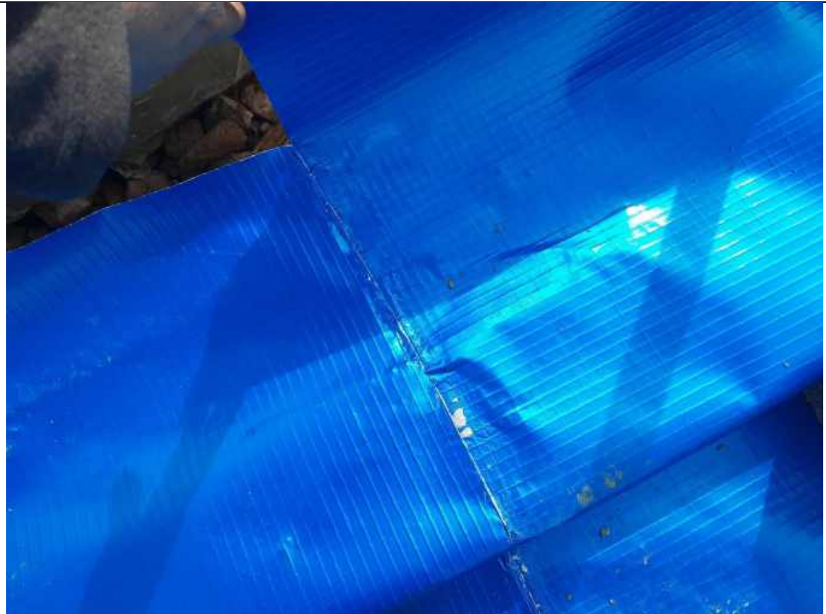
Plate 50: Showing a heat sealed membrane on Plot 16
