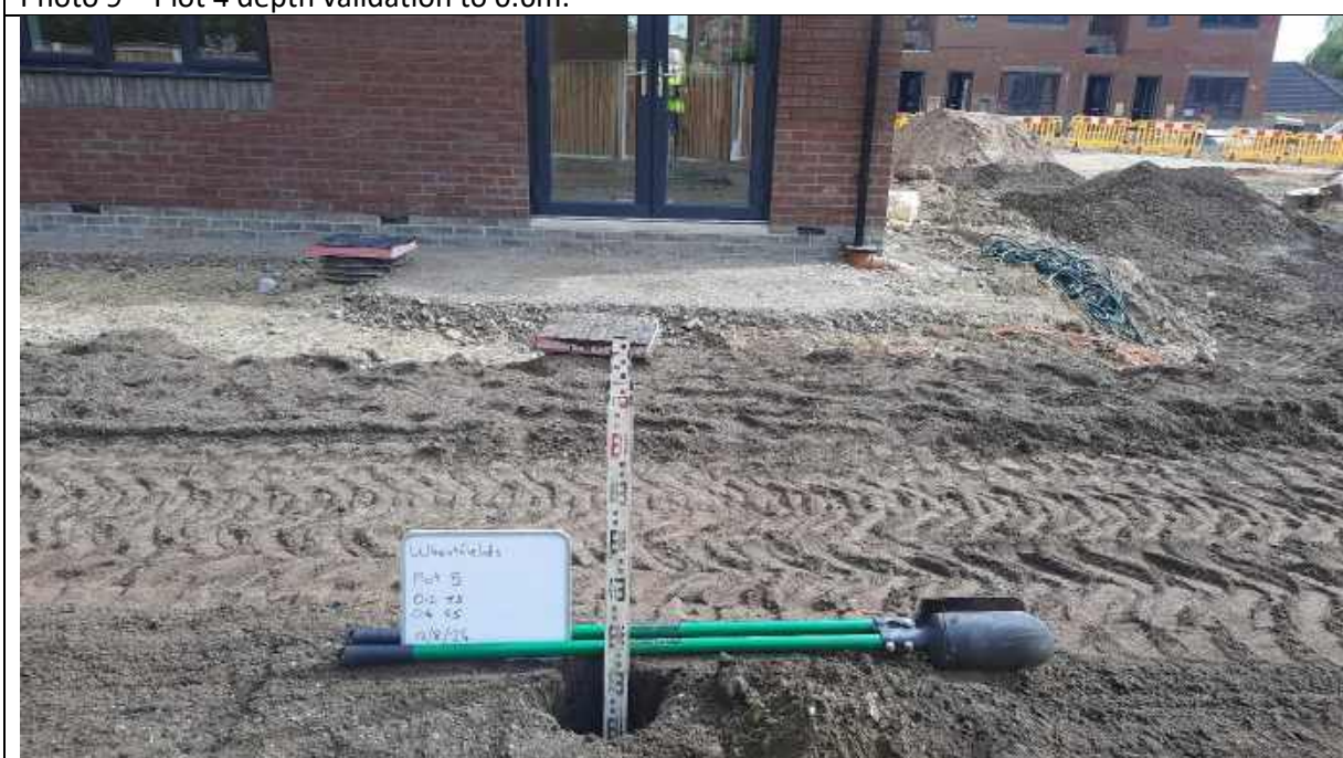
Photo 10 – Plot 5 depth validation to 0.6m.
