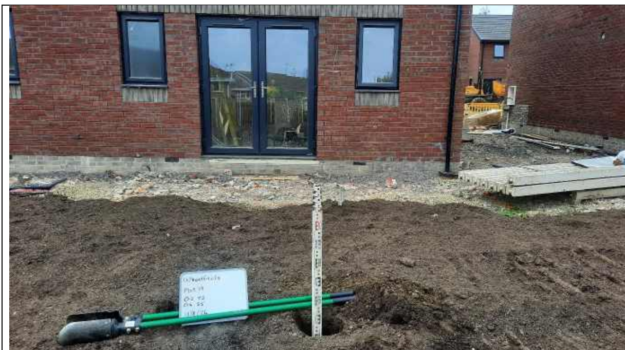
Photo 36 - Plot 19 depth validation to 0.6m.
