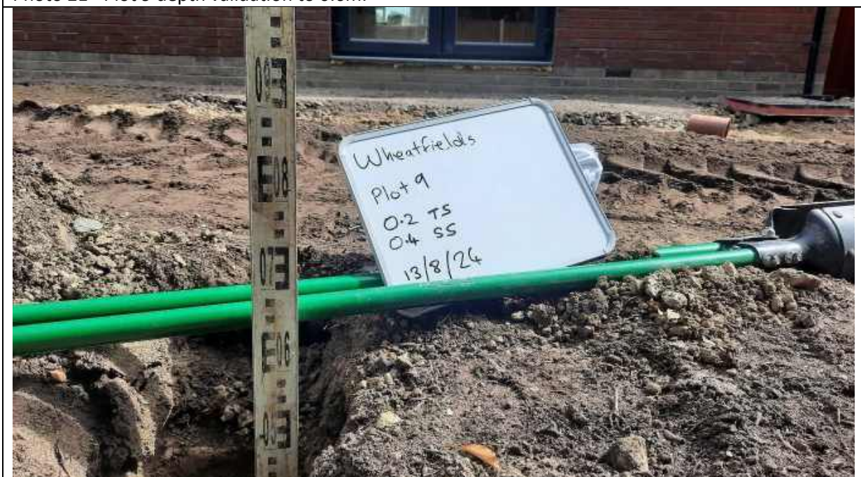
Photo 22 - Plot 9 depth validation to 0.6m.
