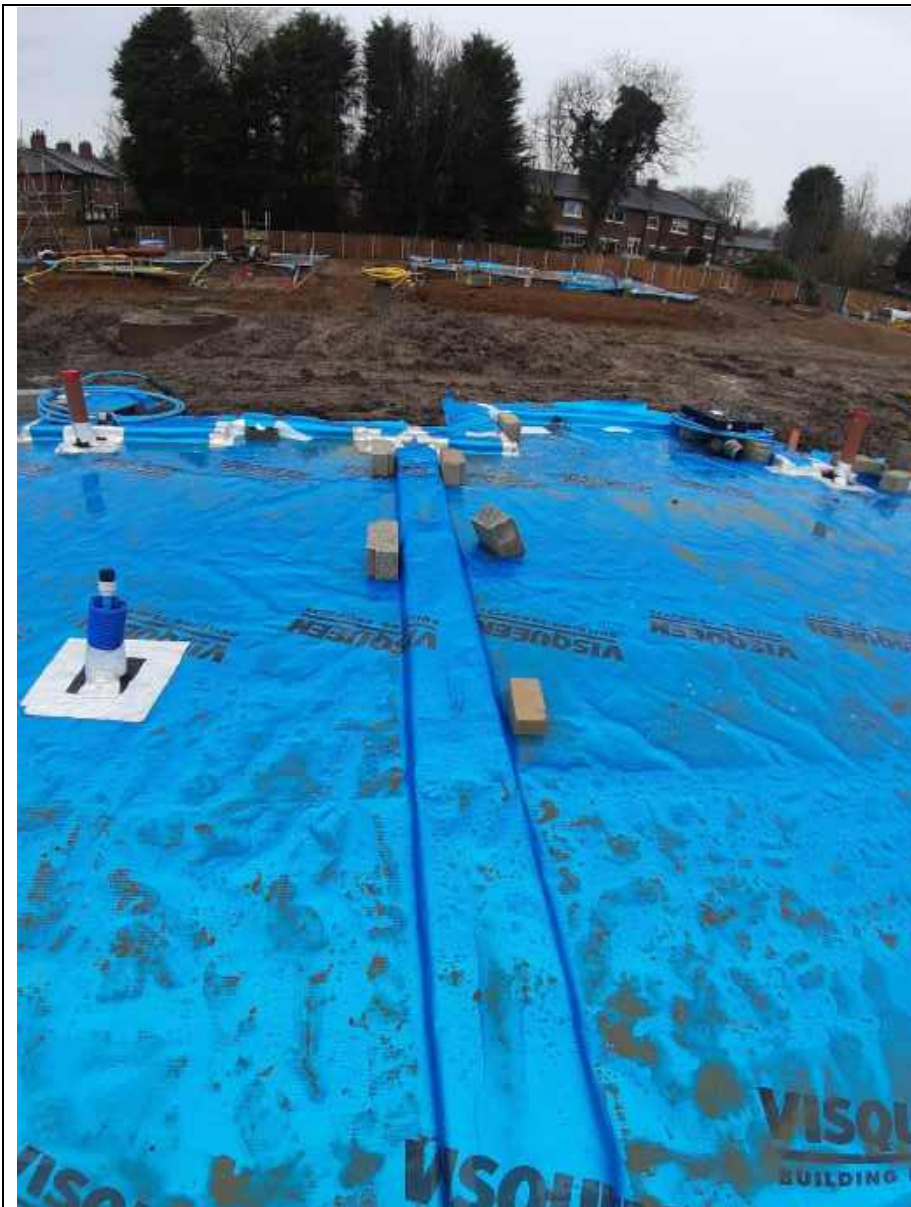
Plate 71: Showing the general condition of the membranes on Plots 21-22
