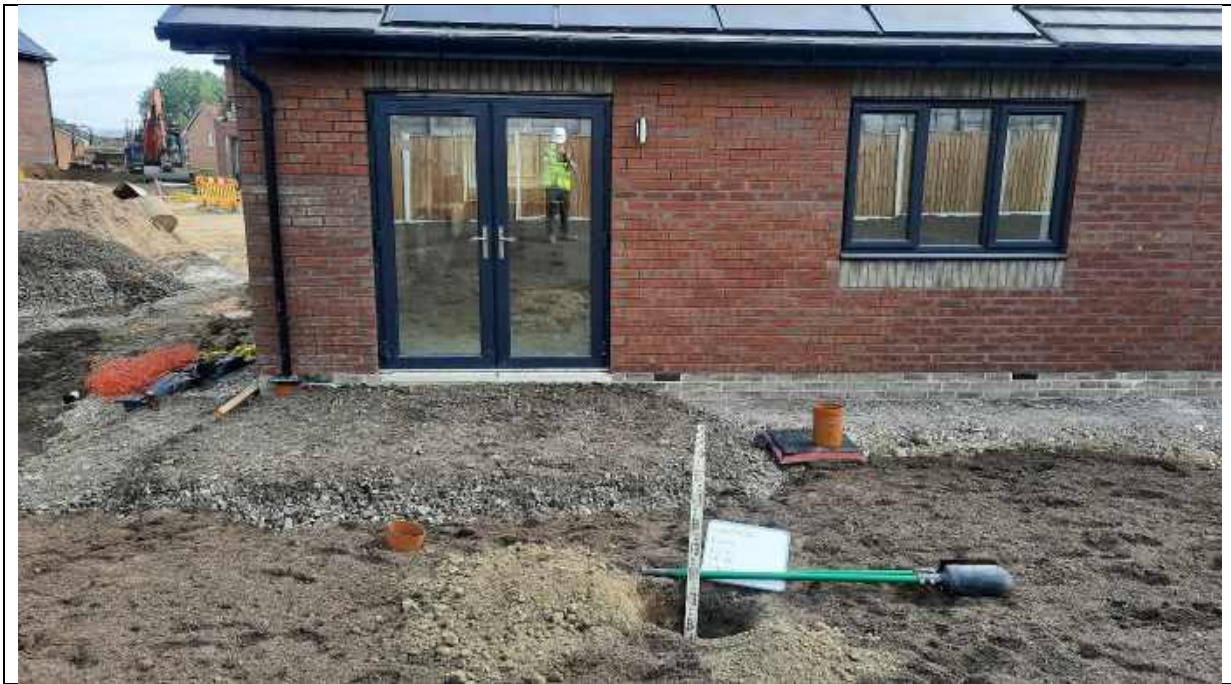
Photo 7 – Plot 4 depth validation to 0.6m.
