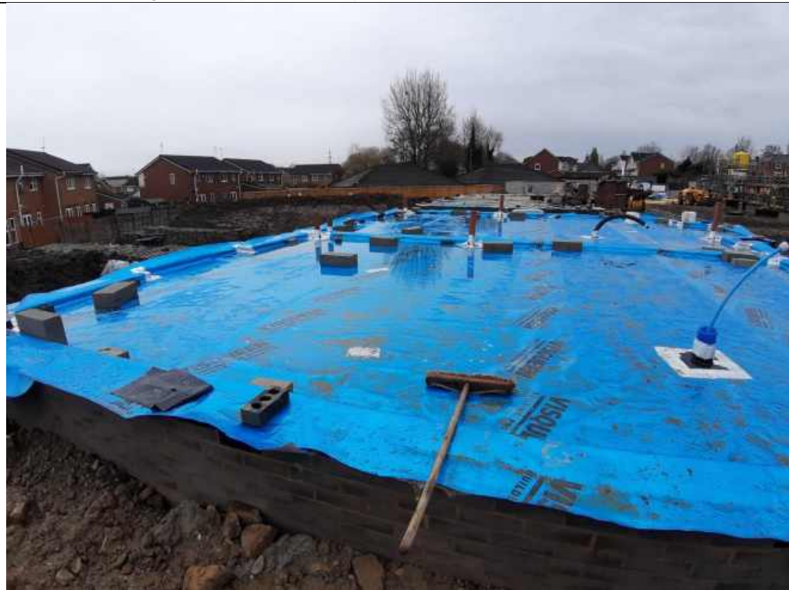
Plate 73: Showing the general condition of the membrane on Plots 23-24
