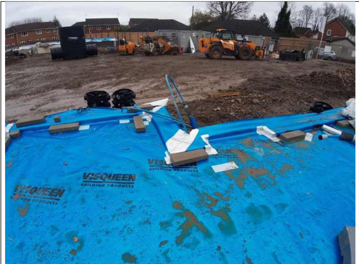
Plate 12: Showing the general condition of the membrane on plots 3-4
