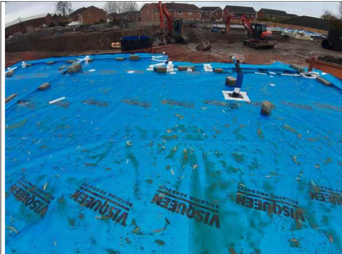
Plate 20: Showing the general condition of the membrane in plots 5-6
