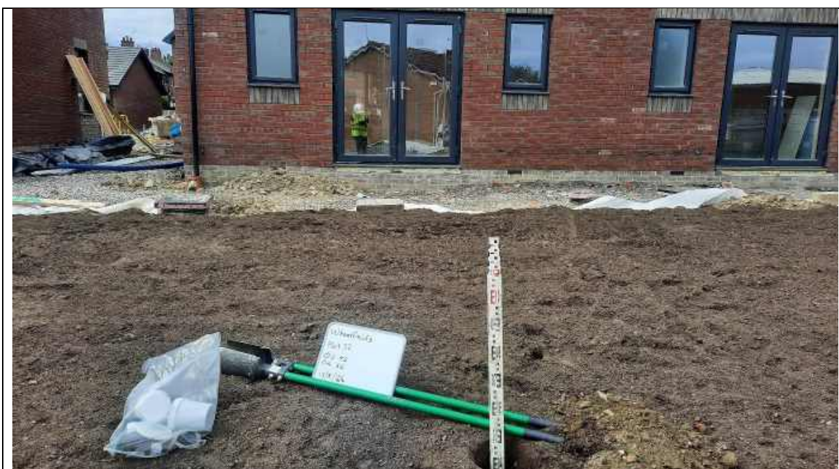
Photo 44 - Plot 22 depth validation to 0.6m.
