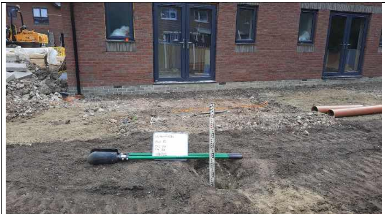
Photo 29 - Plot 11 depth validation to 0.6m.
