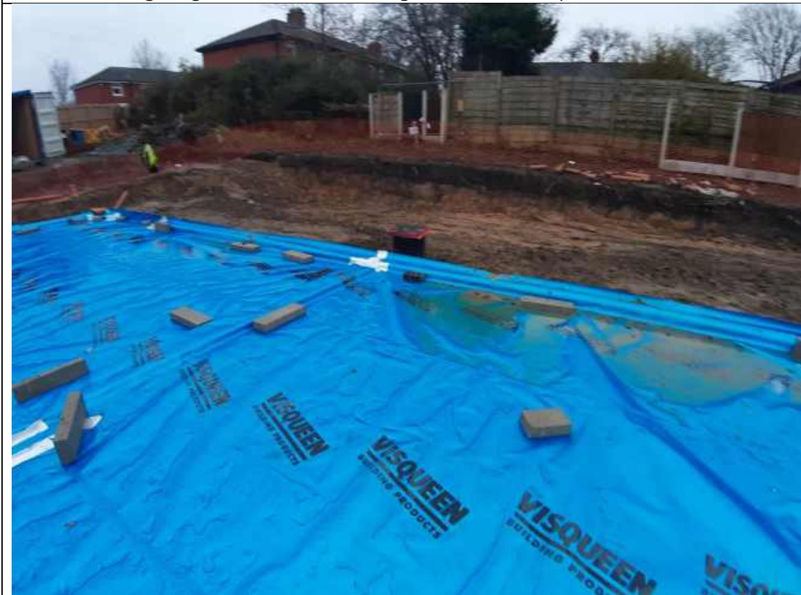
Plate 5: Showing the general condition of the membrane on plots 1-2
