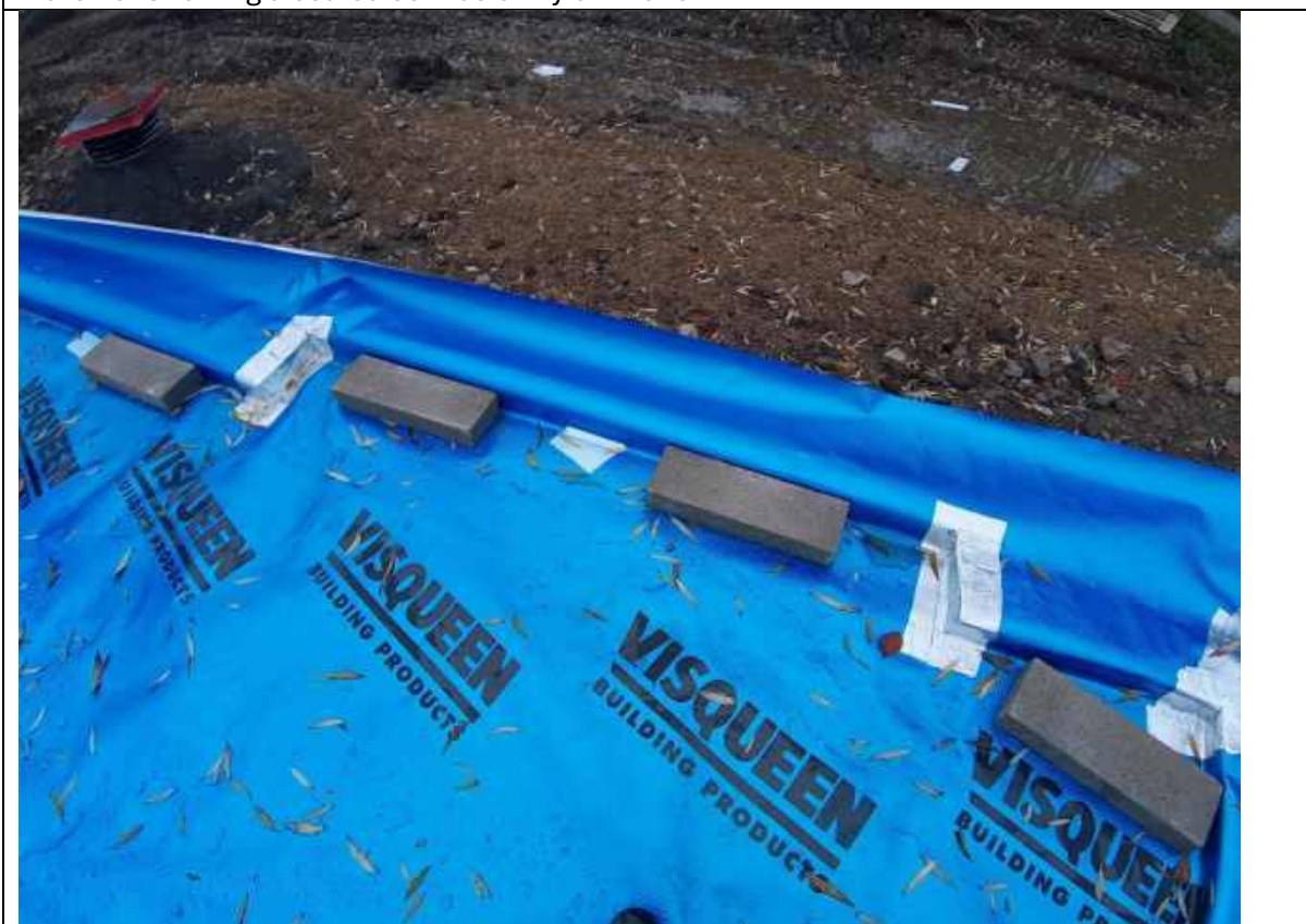
Plate 29: Showing the general condition of the membrane on Plot 8
