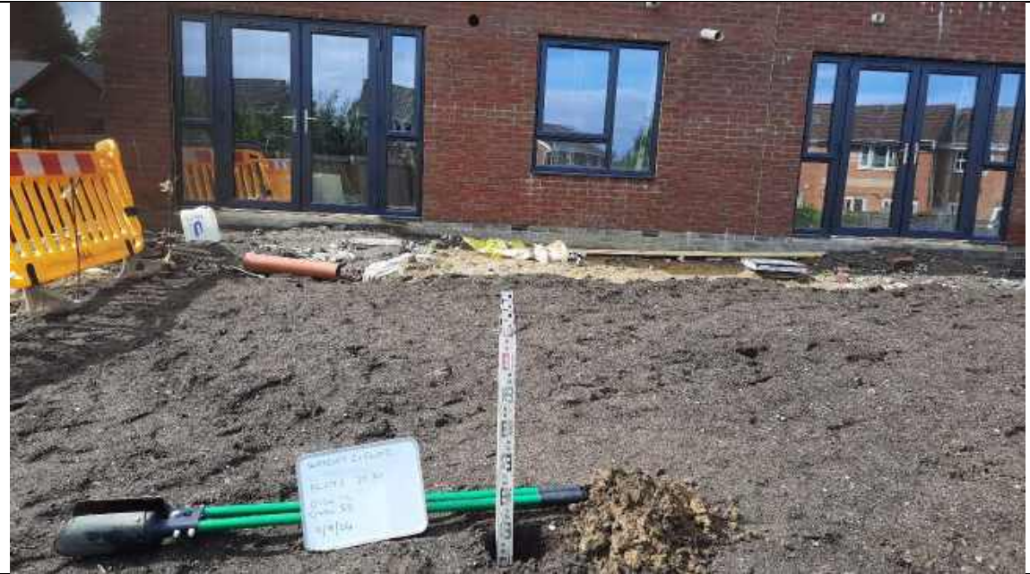
Photo 13 – Plots 29-30 apartments validation hole to 0.6m.
