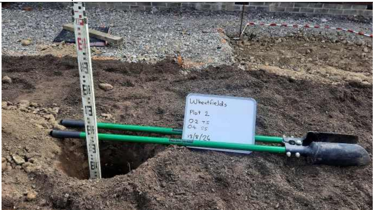
Photo 2 – Plot 2 depth validation to 0.6m.
