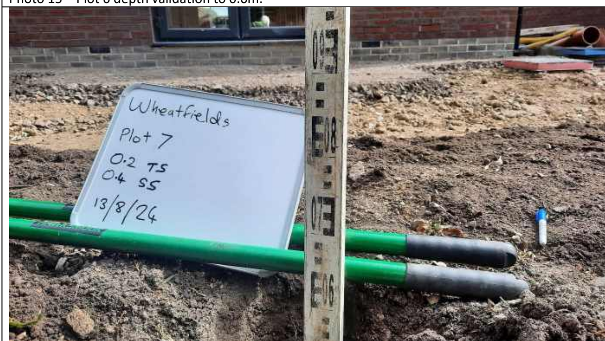
Photo 16 – Plot 7 depth validation to 0.6m.
