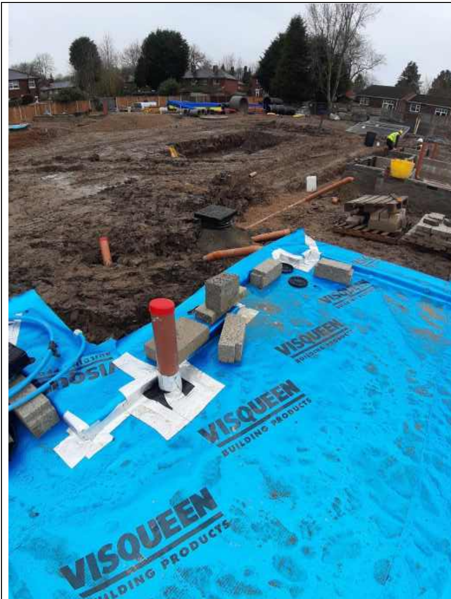
Plate 68: Showing the general condition of the membrane on Plots 21-22
