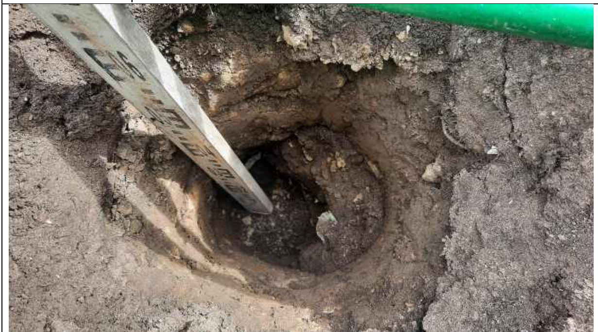
Photo 26 - Plot 10 depth validation to 0.6m.
