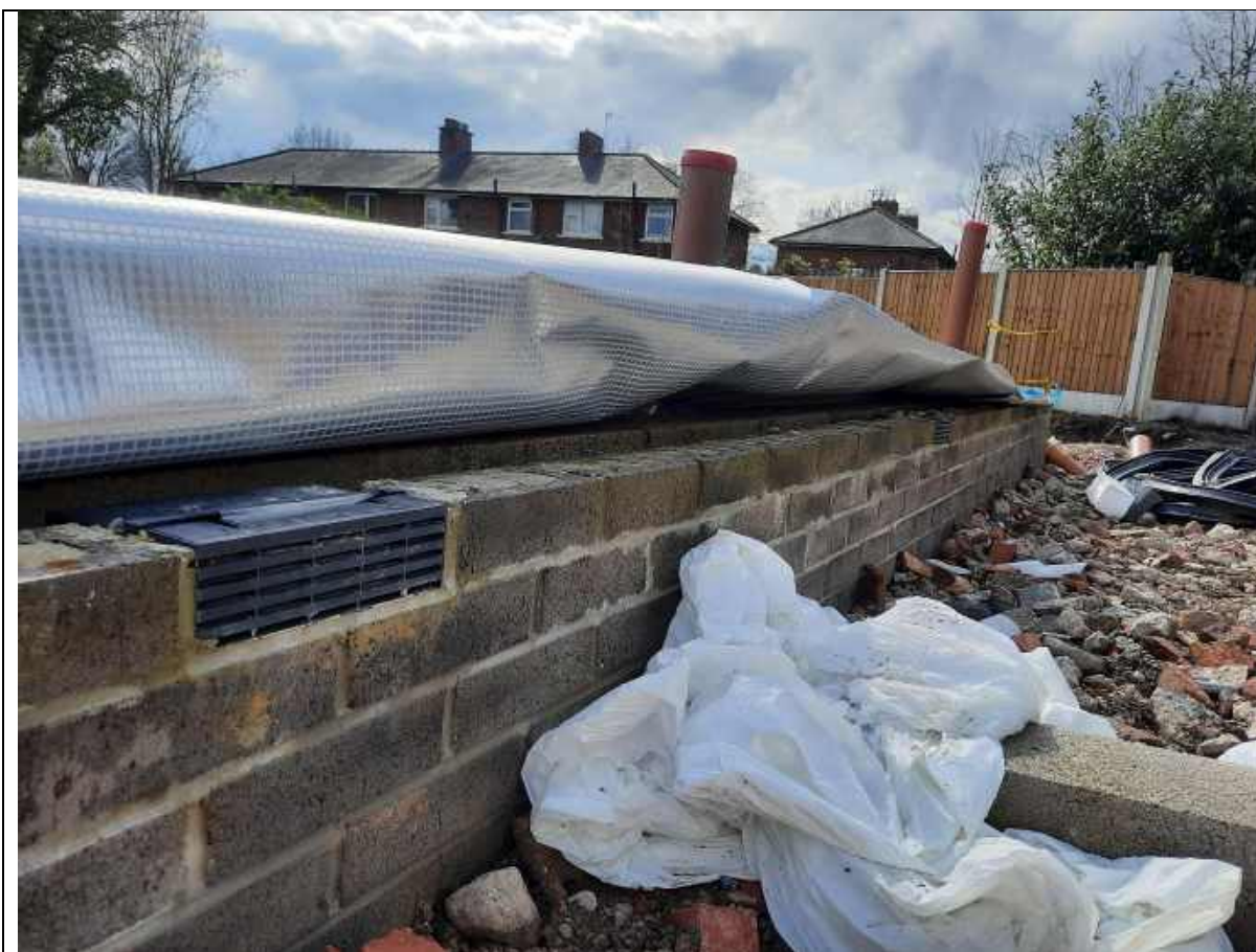
Plate 48: Showing the membrane covering the cavity wall on Plot 15
