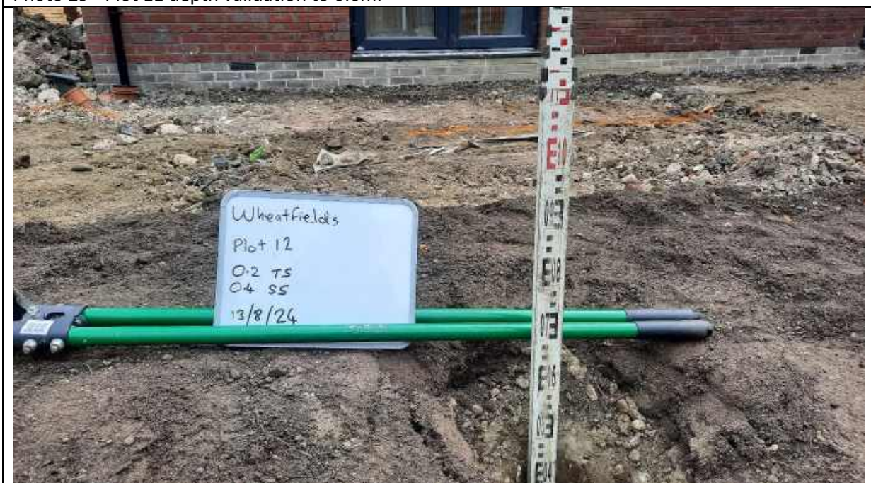
Photo 30 - Plot 12 depth validation to 0.6m.
