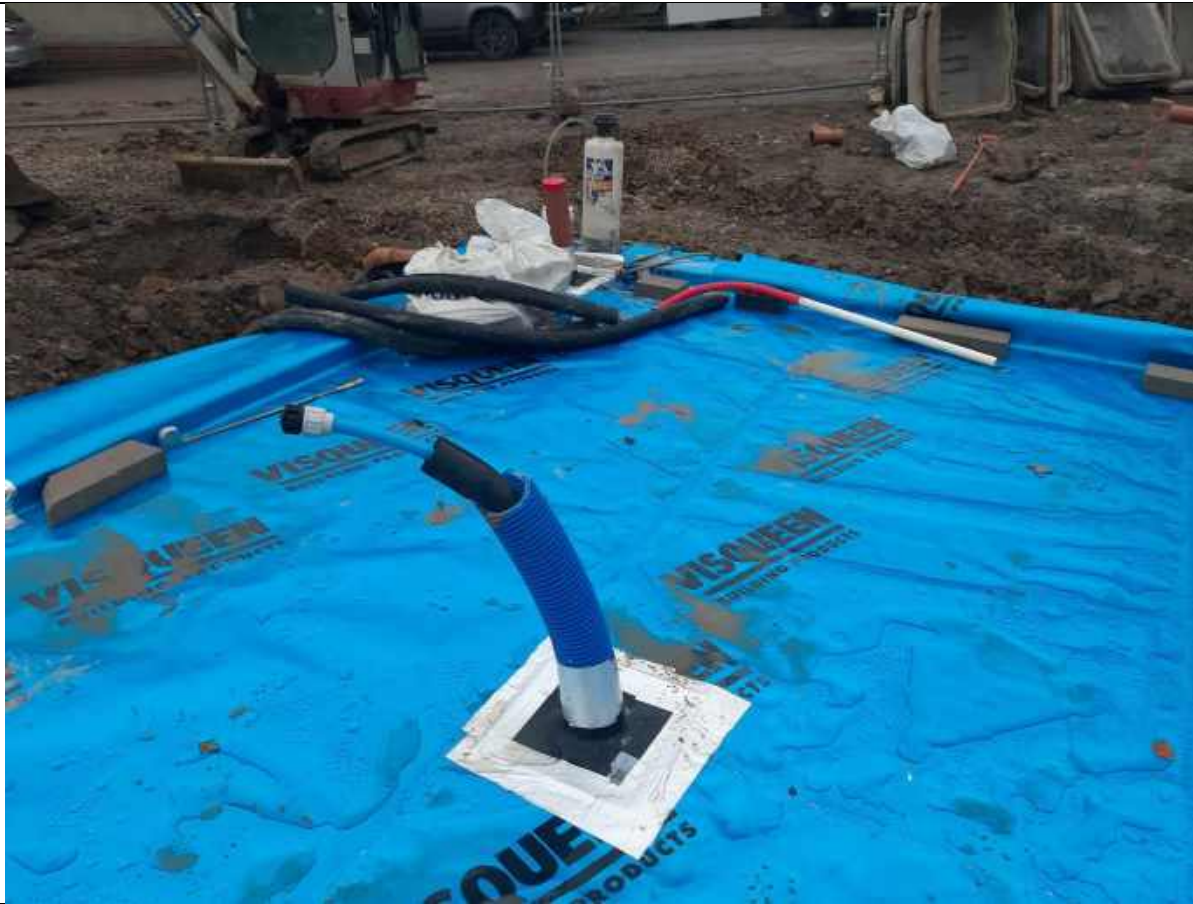
Plate 1: Showing a sealed service entry on plot 1 using Visqueen detailing strip
