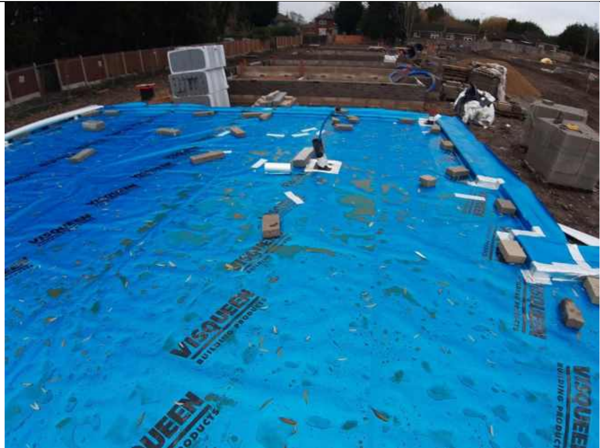
Plate 22: Showing the general condition of the membrane on plots 5&6
