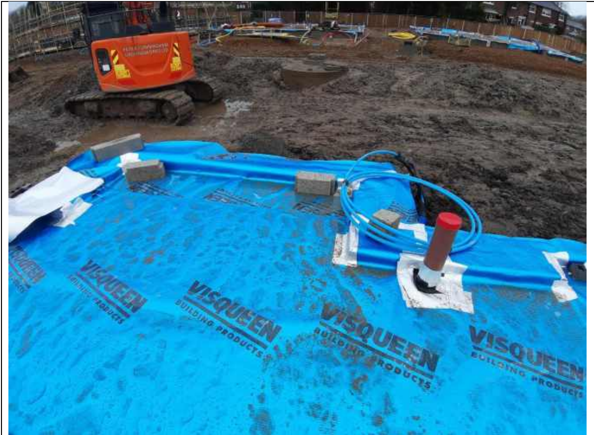
Plate 72: Showing a sealed preformed top hat on Plots 21-22
