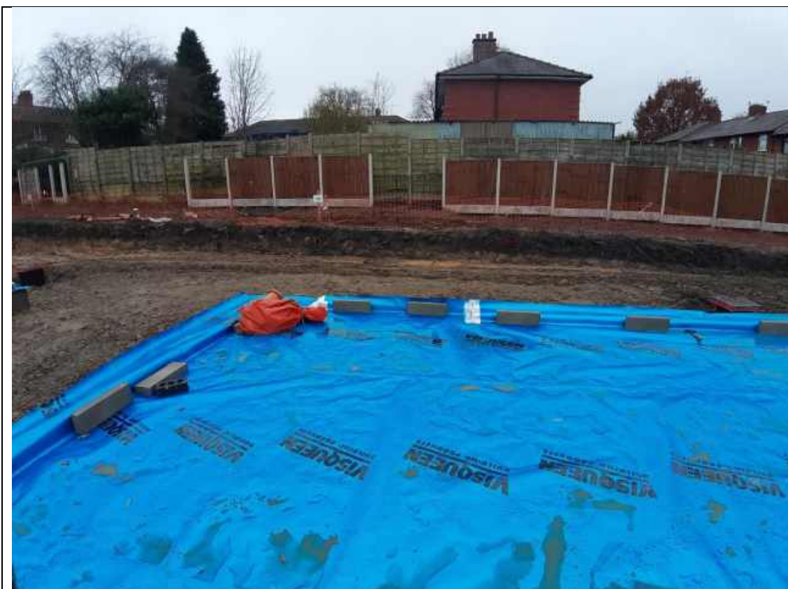
Plate 10: Showing the general condition of the membrane on plot 3-4
