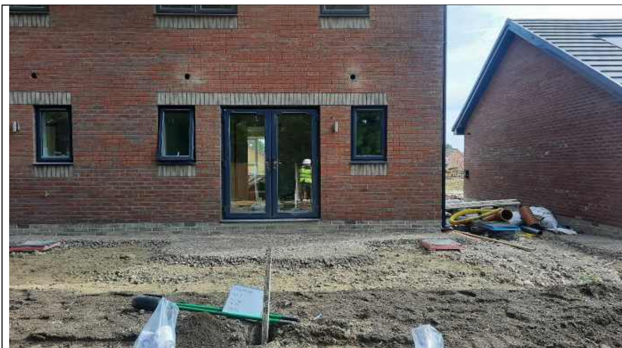
Photo 15 – Plot 6 depth validation to 0.6m.
