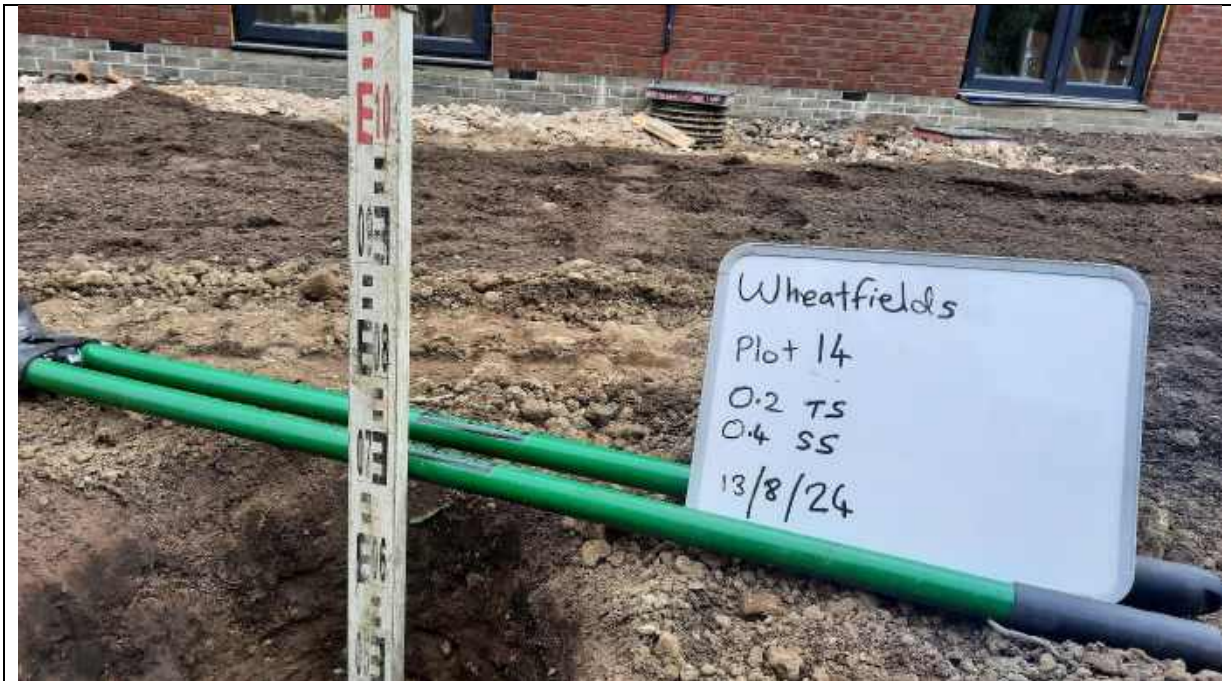
Photo 34 - Plot 14 depth validation to 0.6m.
