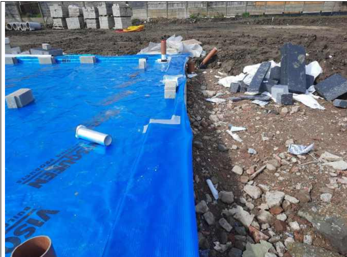
Plate 52: Showing a sealed service entry Plot 17
