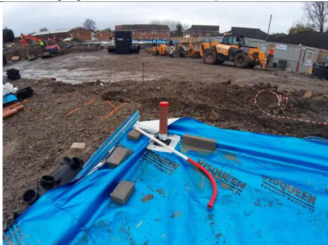
Plot 7: Showing a sealed preformed tophat on a service entry using Visqueen detailing tape on plot 3
