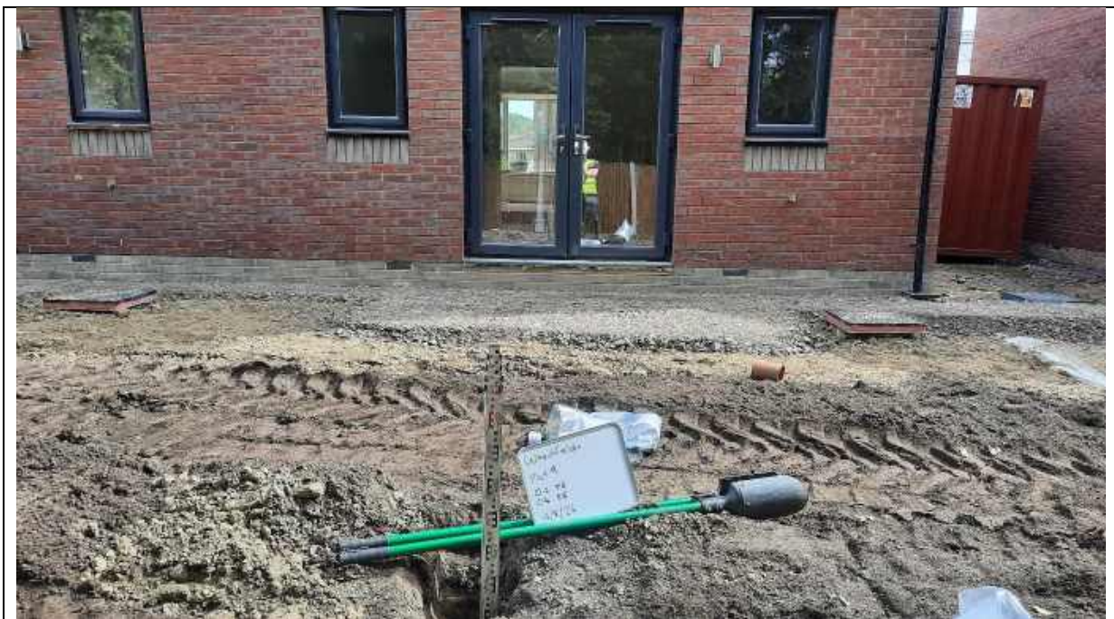
Photo 21 - Plot 9 depth validation to 0.6m.
