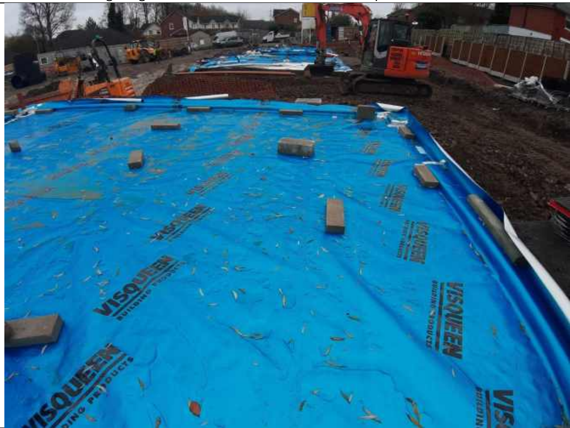
Plate 19: Showing the general condition of the membrane on plots 5-6
