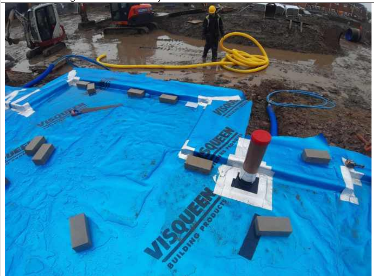
Plate 33: Showing a preformed top hat on Plots 9-10
