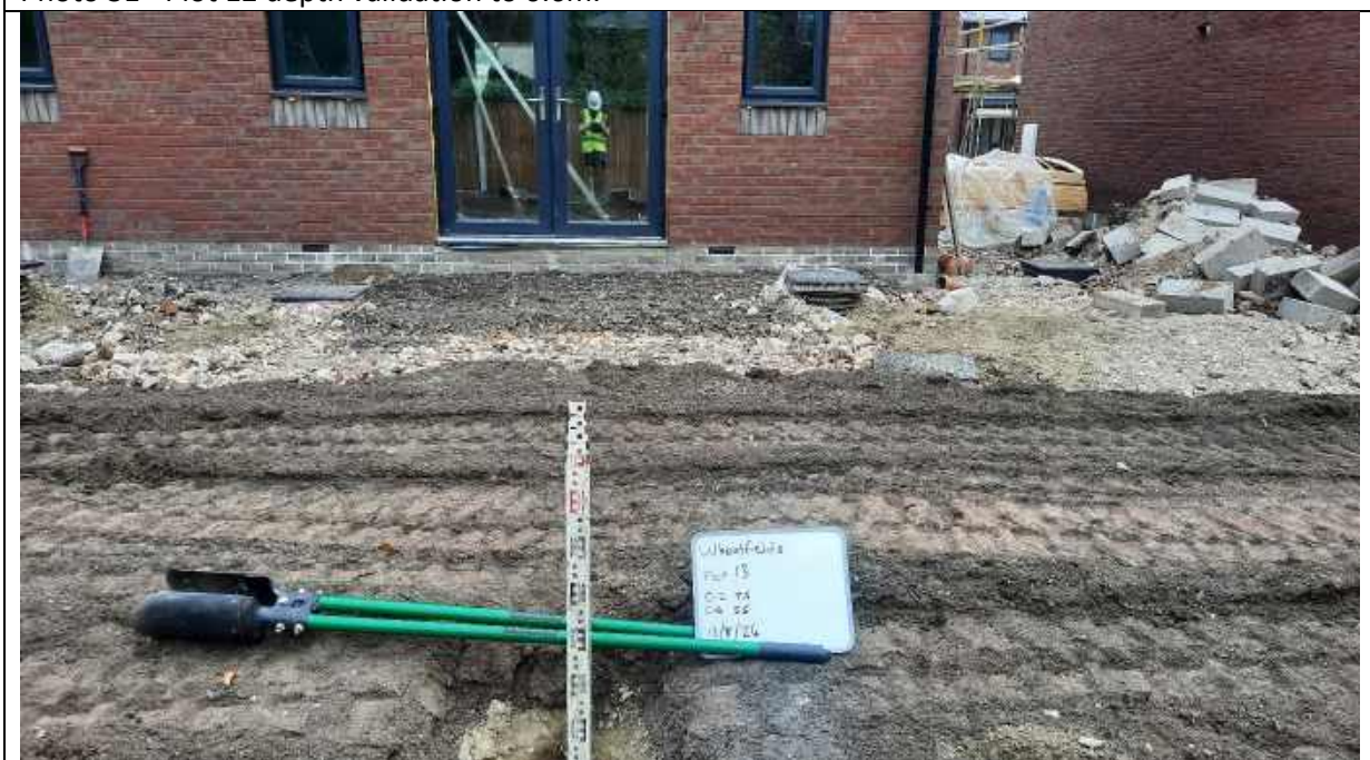
Photo 32 - Plot 13 depth validation to 0.6m.
