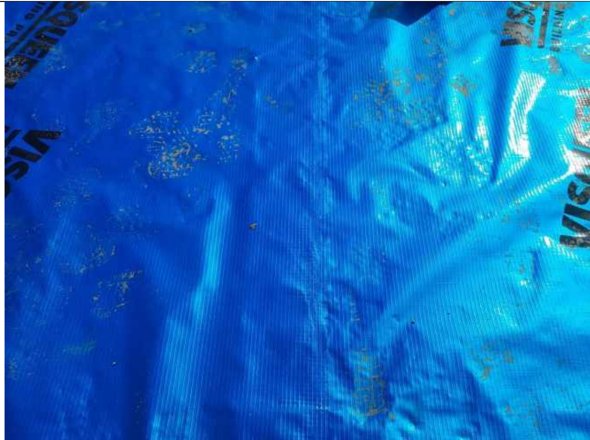
Plate 43: Showing heat sealed seams on the membrane on Plot 13
