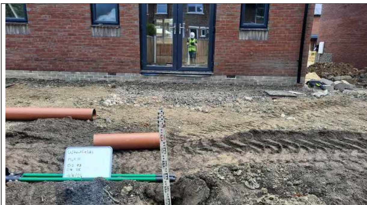
Photo 27 - Plot 11 depth validation to 0.6m.
