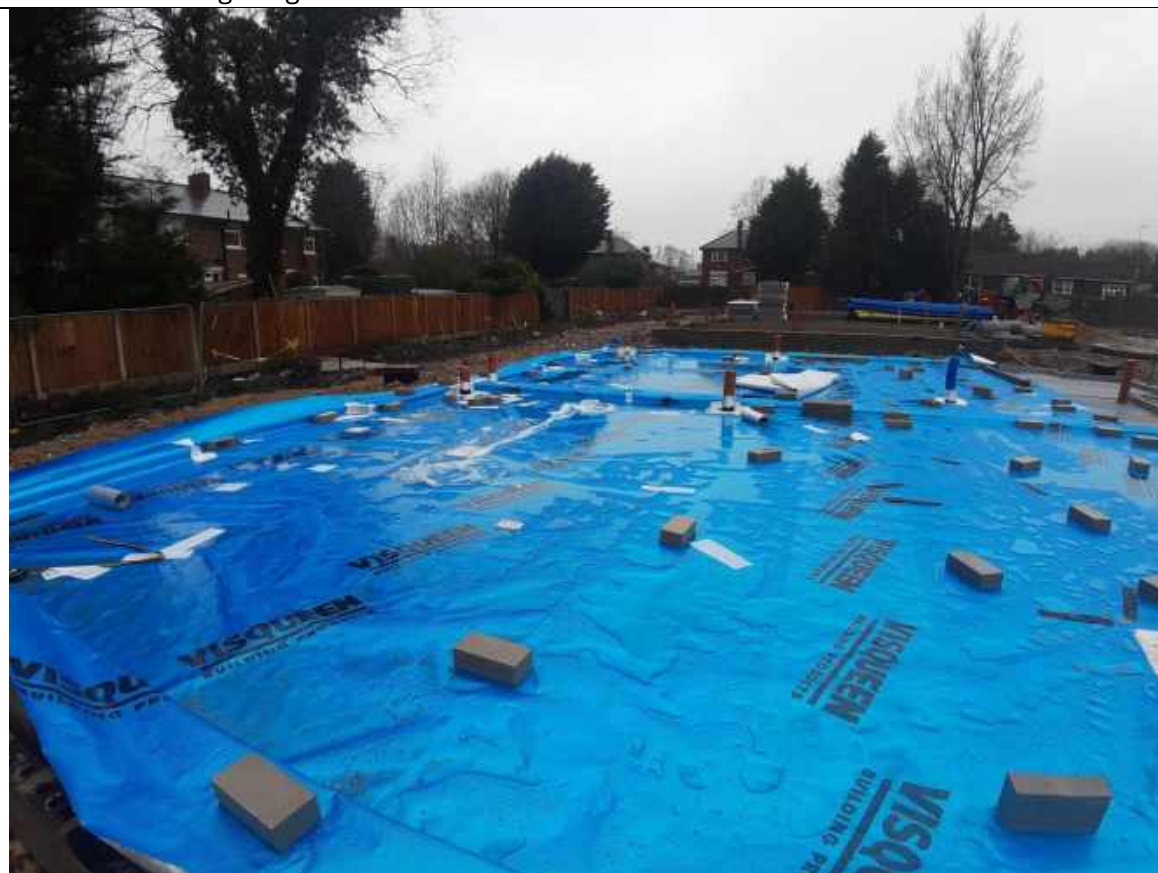
Plate 37: Showing the general condition of the membrane on Plots 11-12
