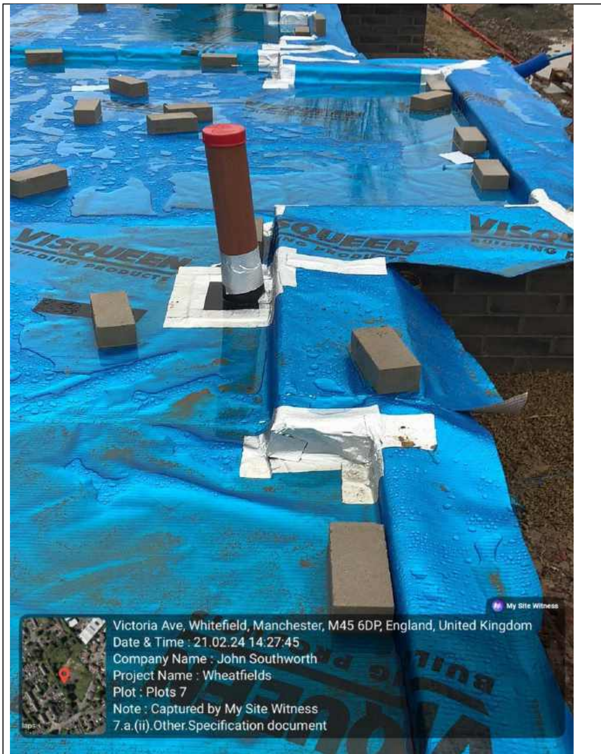
Plate 26: Showing a preformed top hat sealed with visqueen detailing tape Plot 7
