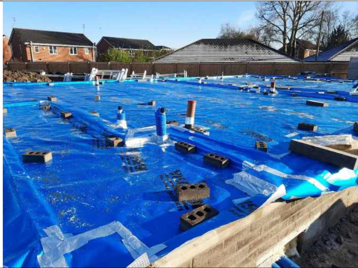
Plate 80: Showing the general condition of Plots 25-26
