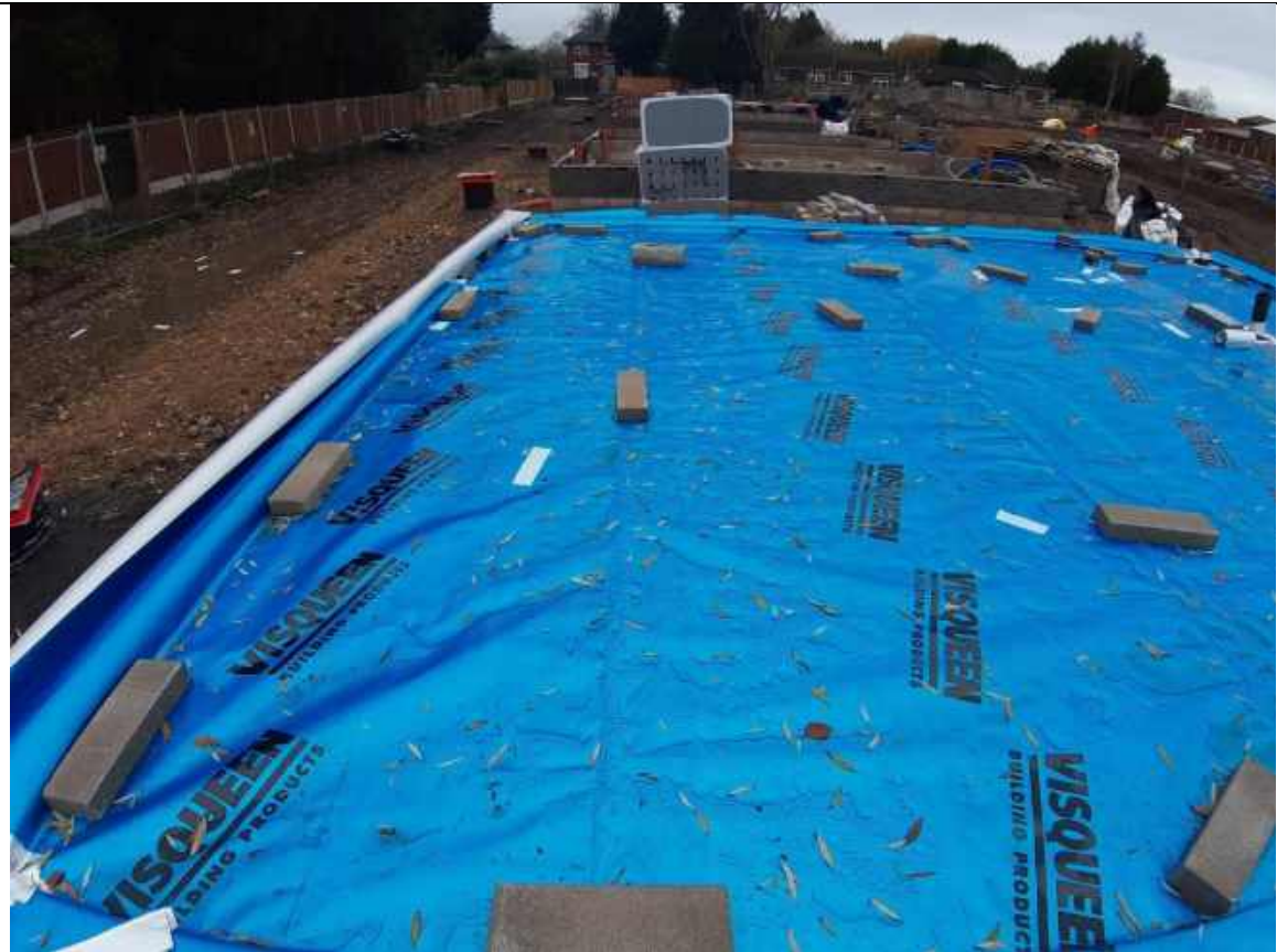
Plate 18: Showing the general condition of the membrane on plots 5-6
