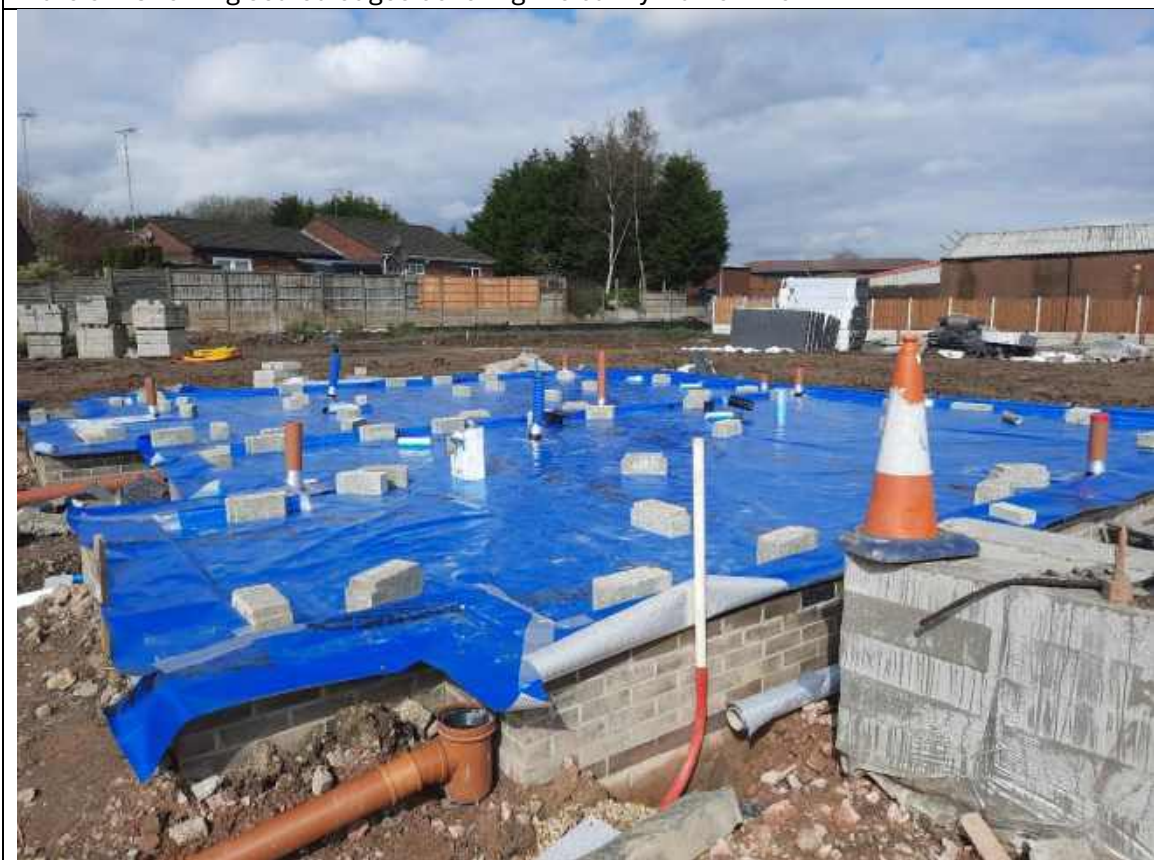
Plate 55: Showing the general condition of the membrane on Plot 18
