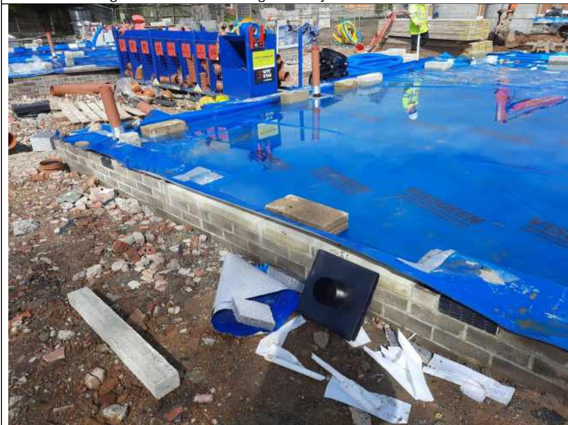
Plate 47: Showing the general condition of the membrane on Plot 15
