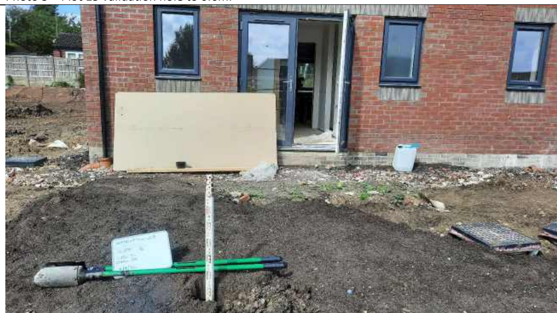
Photo 4 – Plot 16 validation hole to 0.6m.
