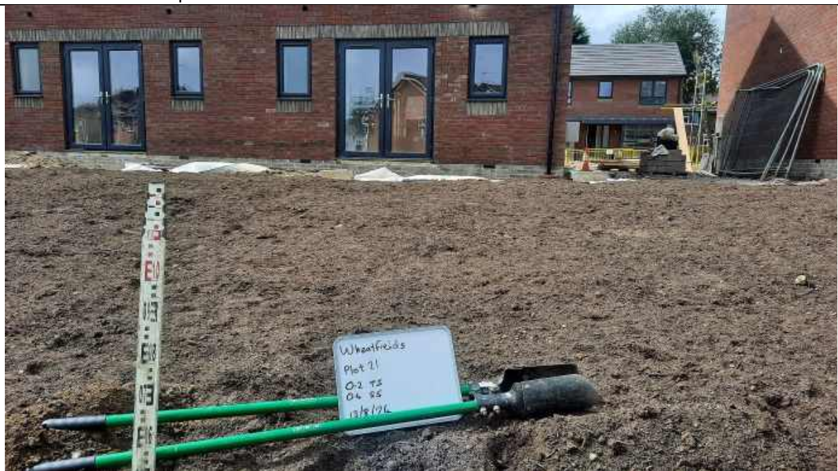
Photo 41 - Plot 21 depth validation to 0.6m.
