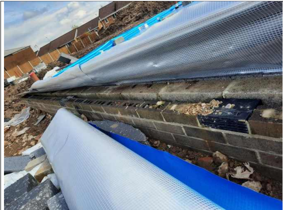
Plate 54: Showing sealed edges covering the cavity wall on Plot 17
