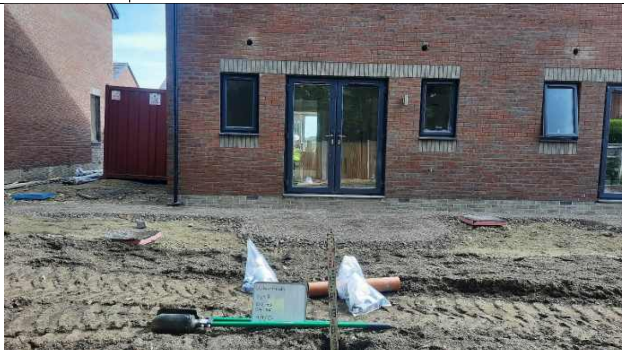
Photo 18 – Plot 8 depth validation to 0.6m.
