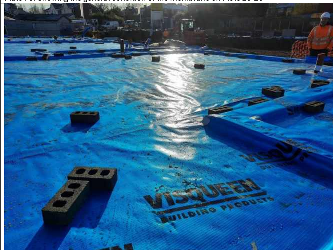
Plate 79: Showing the general condition of the membrane on Plots 25-26
