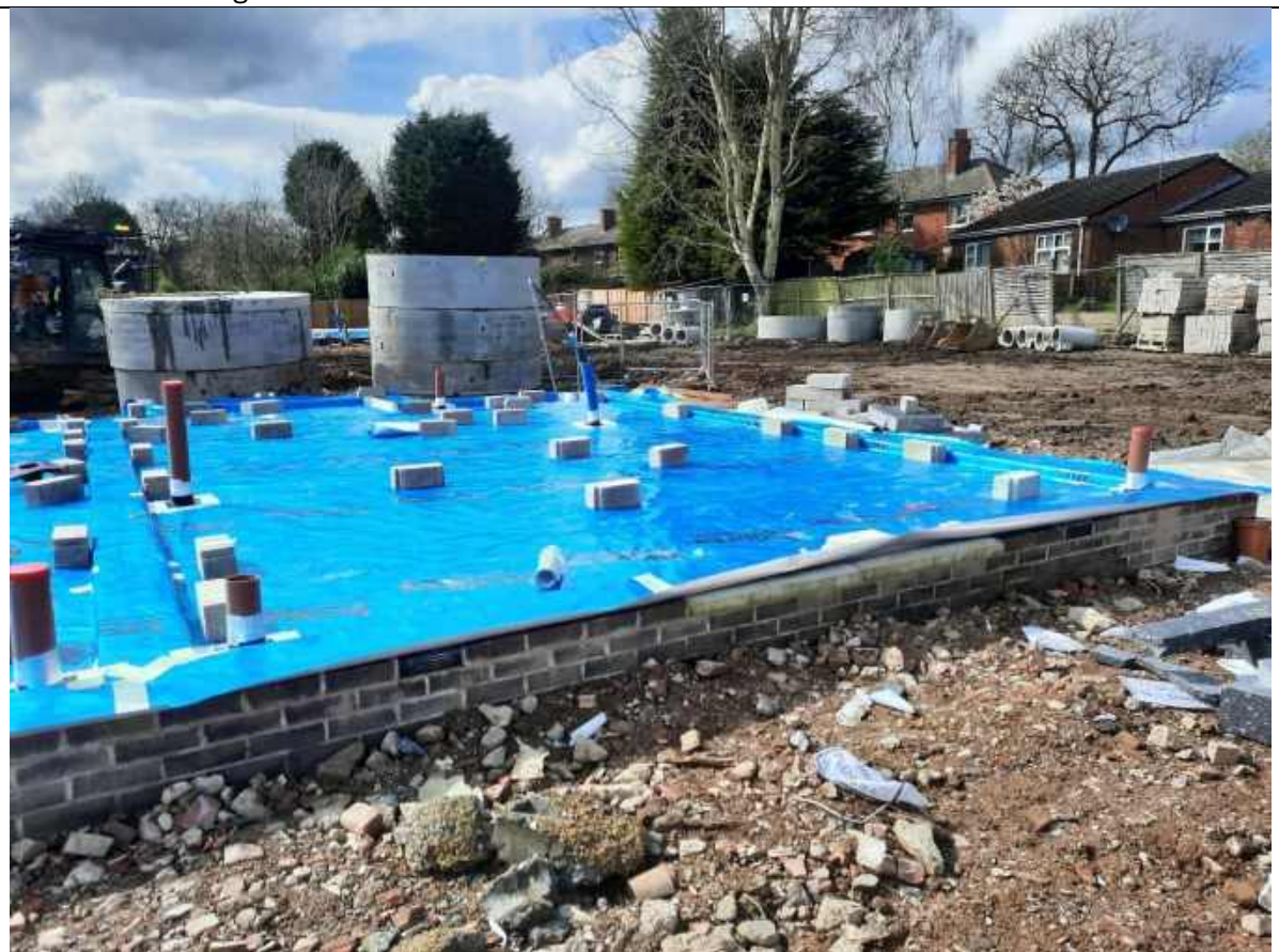
Plate 51: Showing the general condition of the membrane on Plot 17
