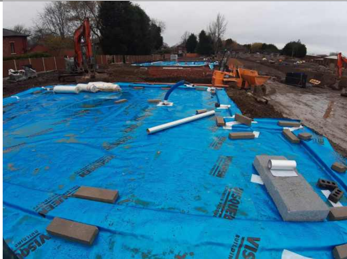
Plate 13: Showing the general condition of the membrane on plots 3-4
