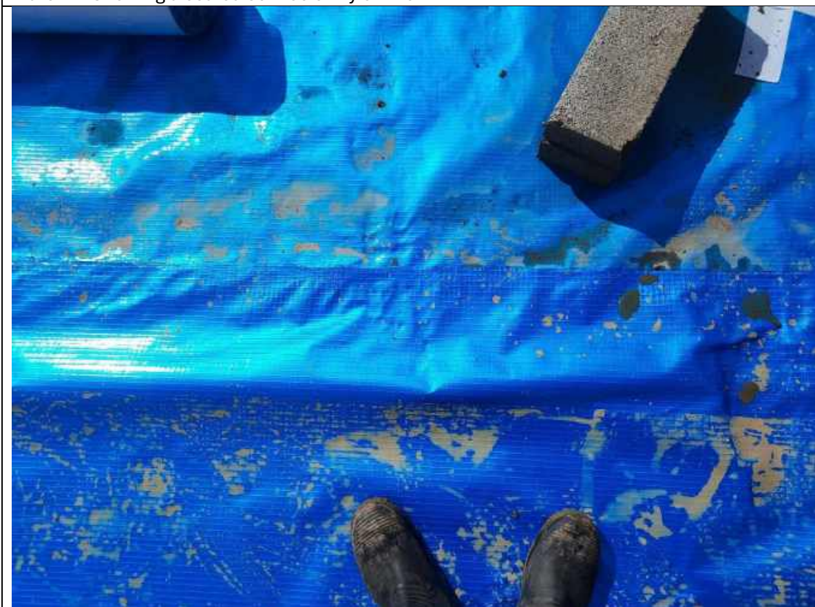
Plate 45: Showing heat sealed seams on Plot 14
