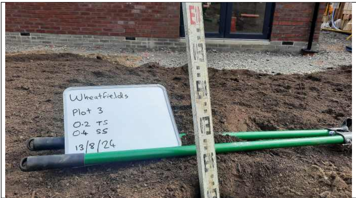
Photo 5 – Plot 3 depth validation to 0.6m.
