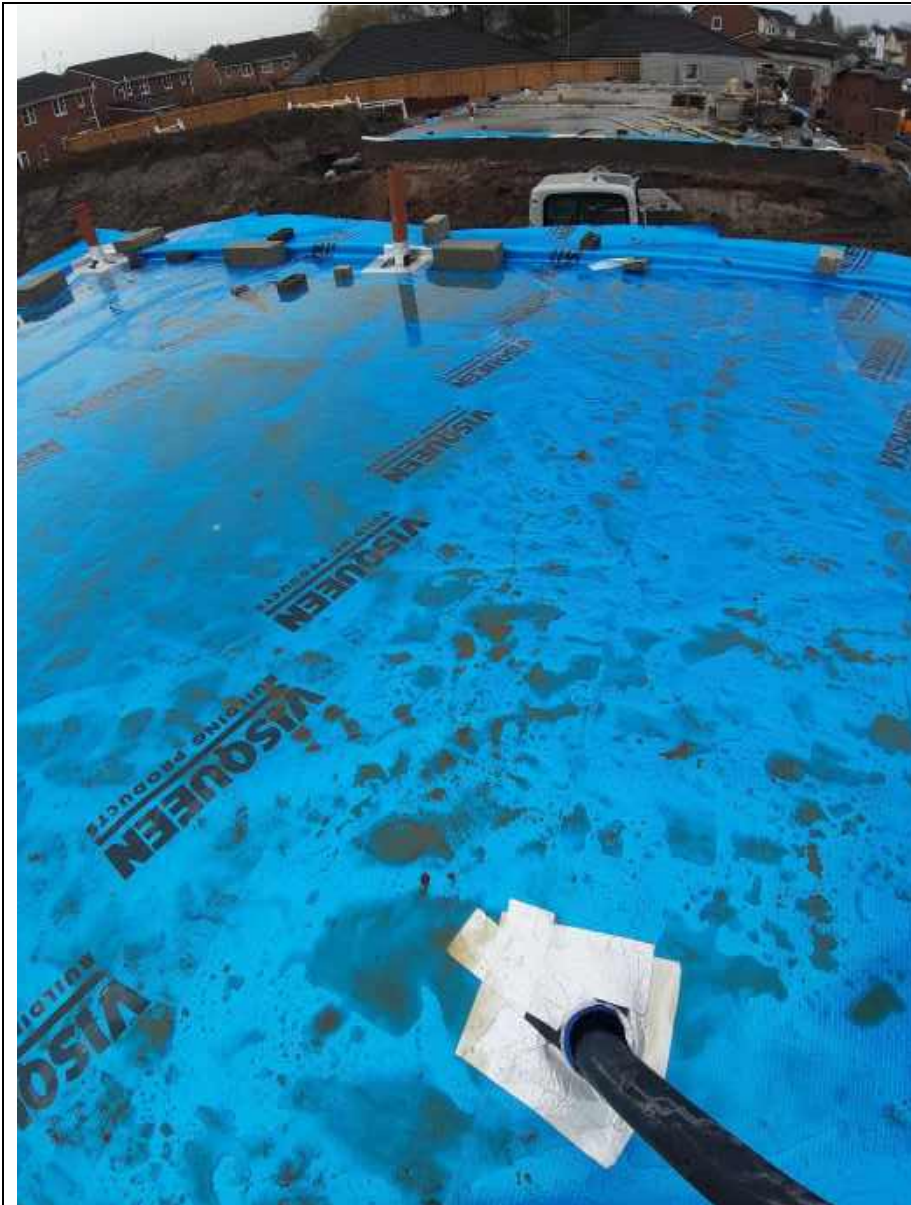
Plate 77: Showing the general condition of the membrane in Plots 23-24
