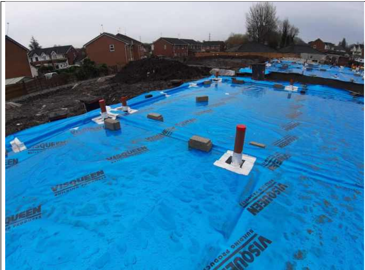
Plate 69: Showing the general condition of the membrane on Plots 21-22
