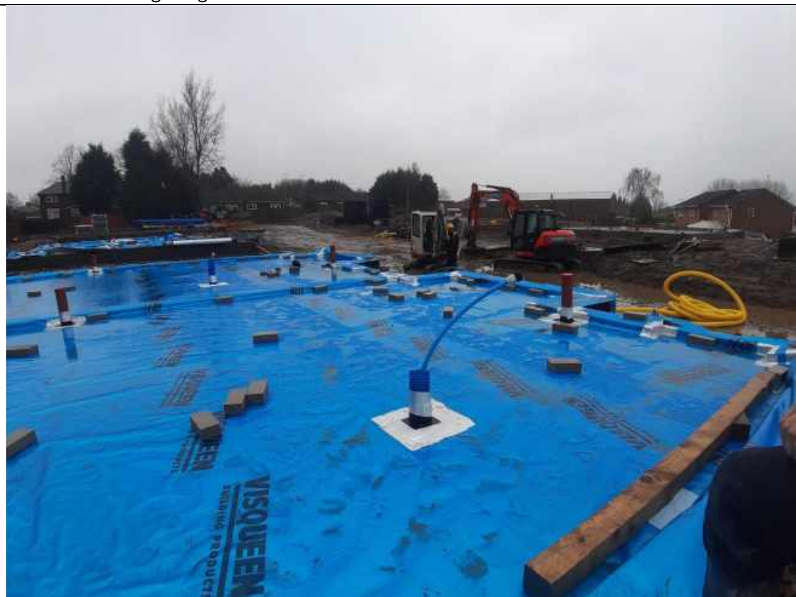
Plate 31: Showing the general condition of the membrane on Plots 9-10
