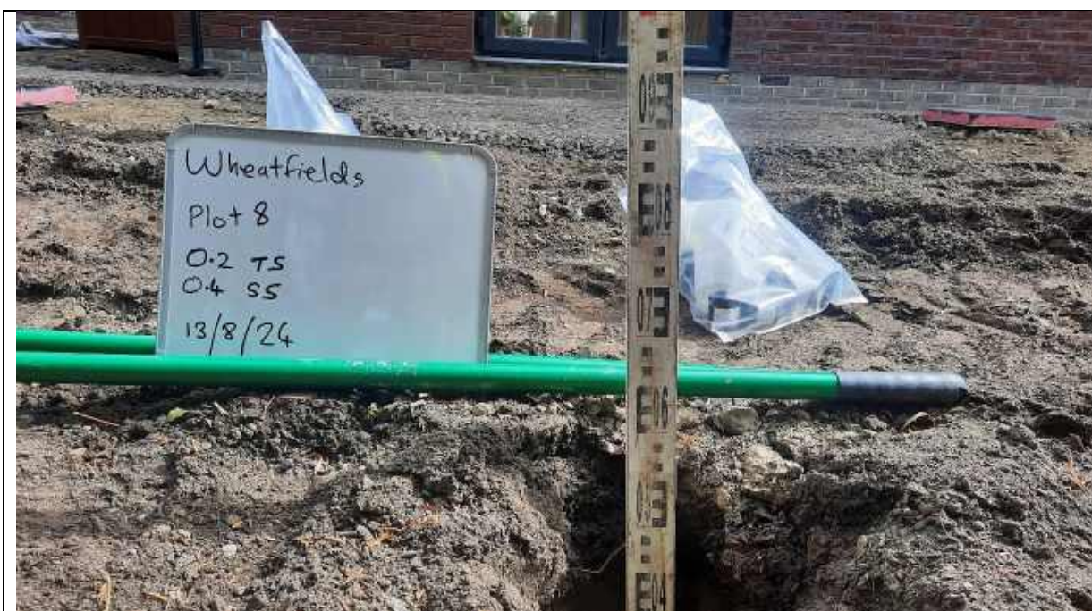
Photo 19 – Plot 8 depth validation to 0.6m.
