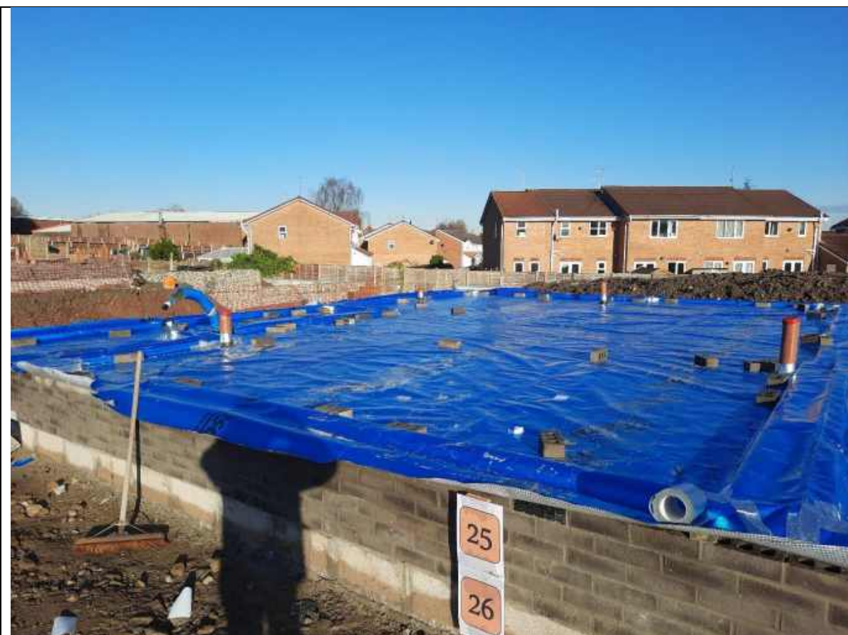
Plate 78: Showing the general condition of the membrane on Plots 25-26
