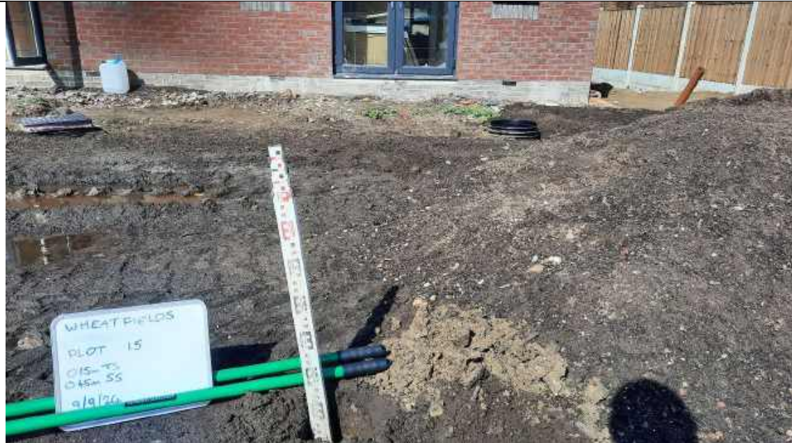
Photo 1 – Plot 15 validation hole to 0.6m.
