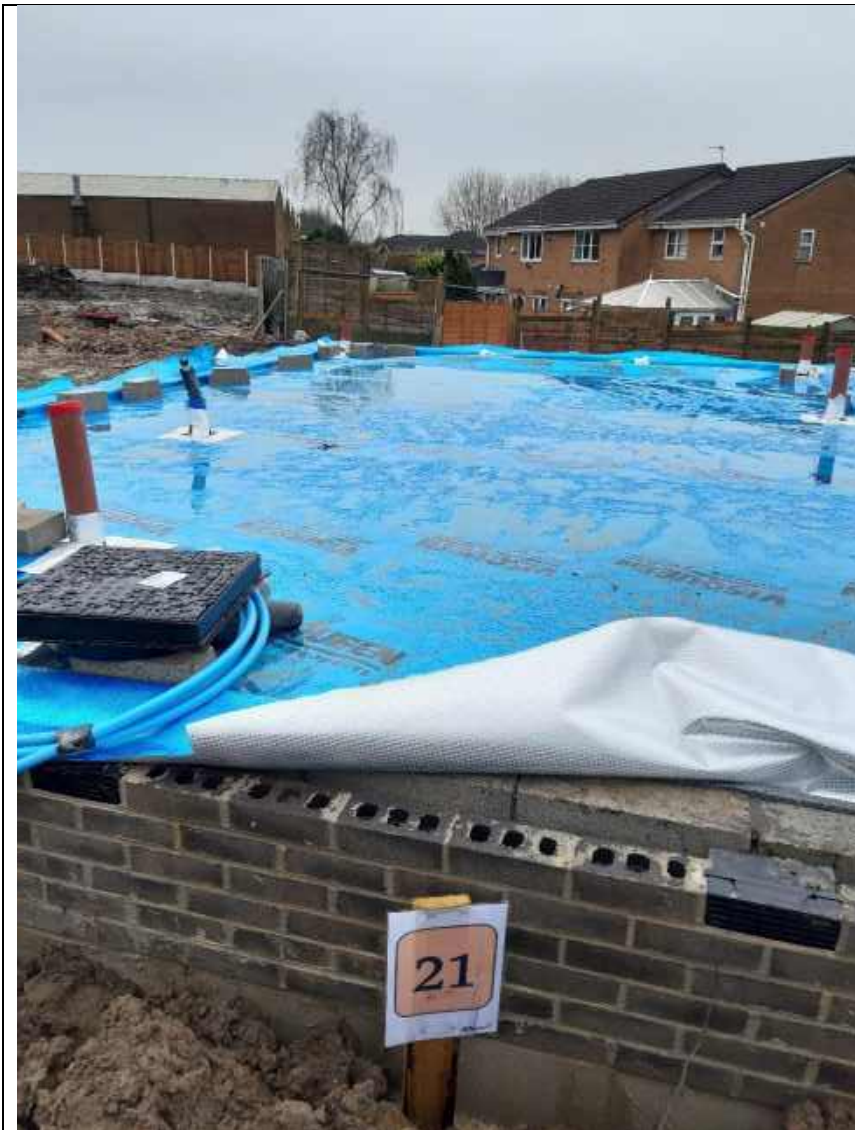
Plate 67: Showing the general condition of the membrane on Plots 21-22
