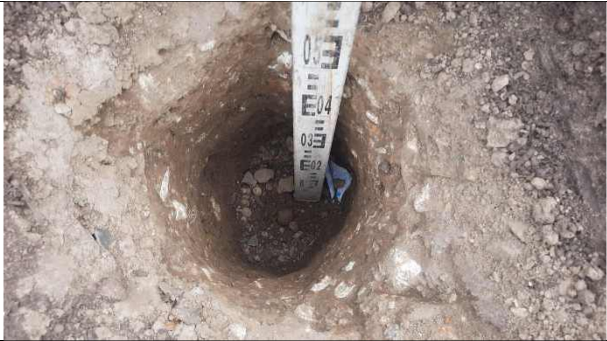
Photo 33 - Plot 13 depth validation to 0.6m.
