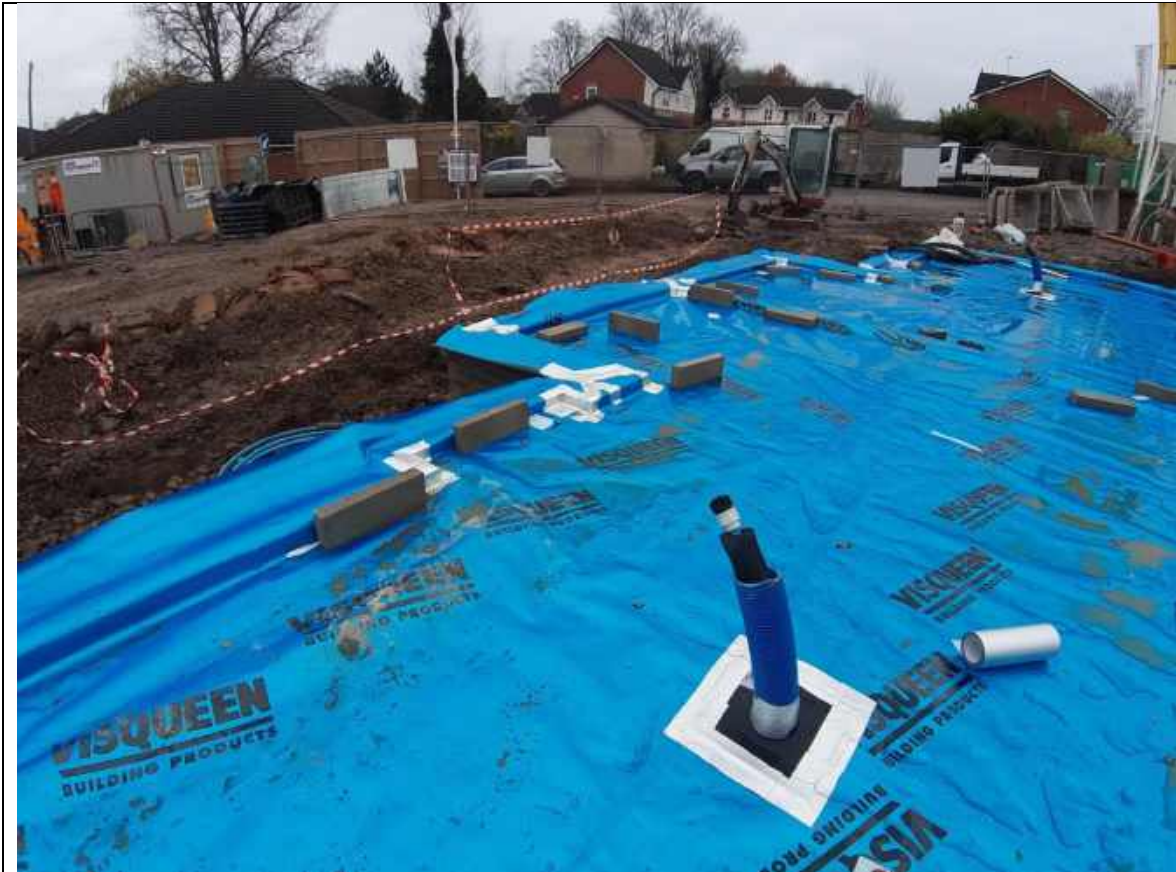
Plate 8: Showing the general condition of the membrane and sealed service entries in plots 3-4
