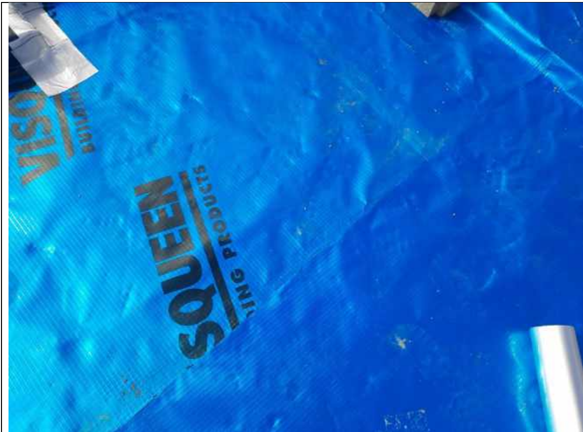
Plate 58: Showing heat sealed seams on Plot 18
