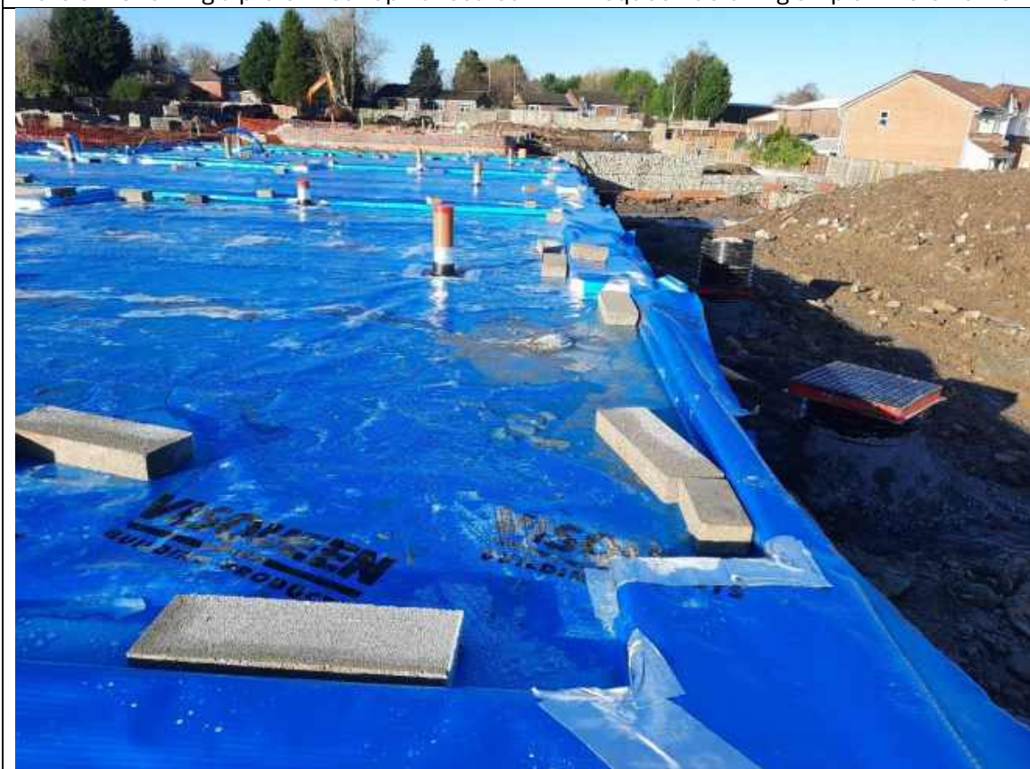
Plate 83: Showing the general condition of Plots 25-26
