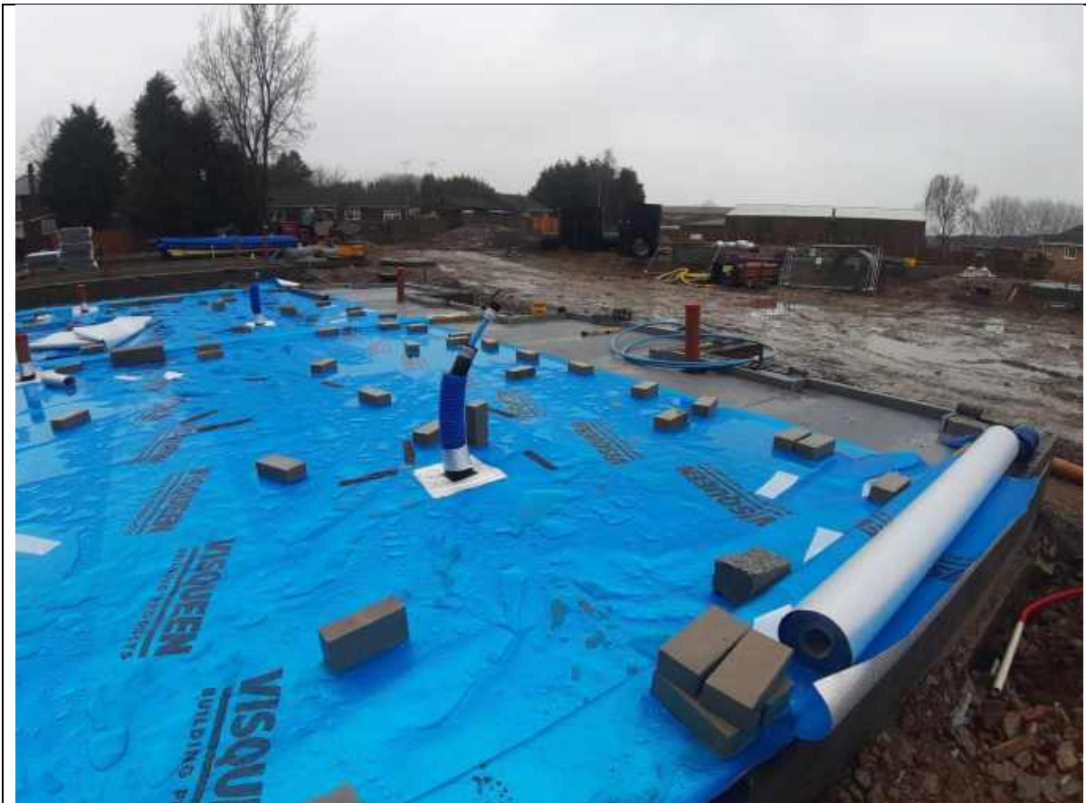
Plate 36: Showing the general condition of the membrane on Plots 11-12
