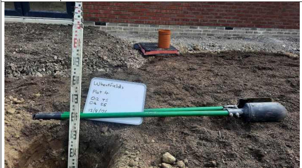
Photo 8 – Plot 4 depth validation to 0.6m.
