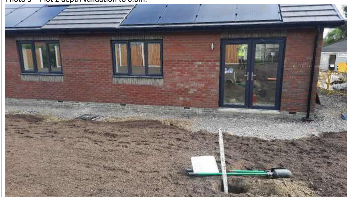
Photo 4 – Plot 3 depth validation to 0.6m.
