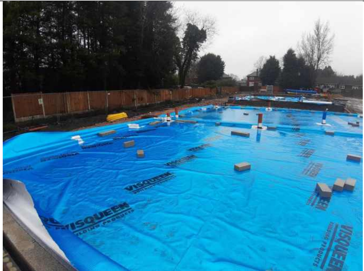
Plate 30: Showing the general condition of the membrane on Plots 9-10
