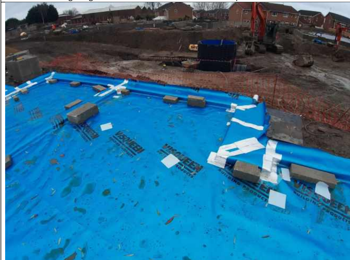
Plate 15: Showing the general condition of the membrane on plots 5-6
