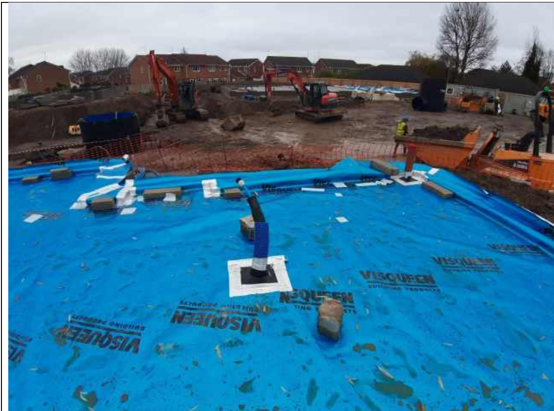
Plate 14: Showing the general condition of the membrane on plots 3-4
