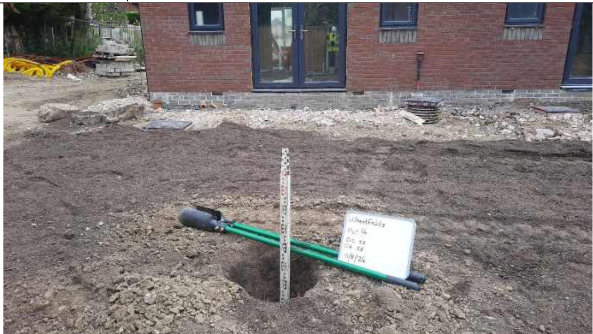
Photo 34 - Plot 14 depth validation to 0.6m.
