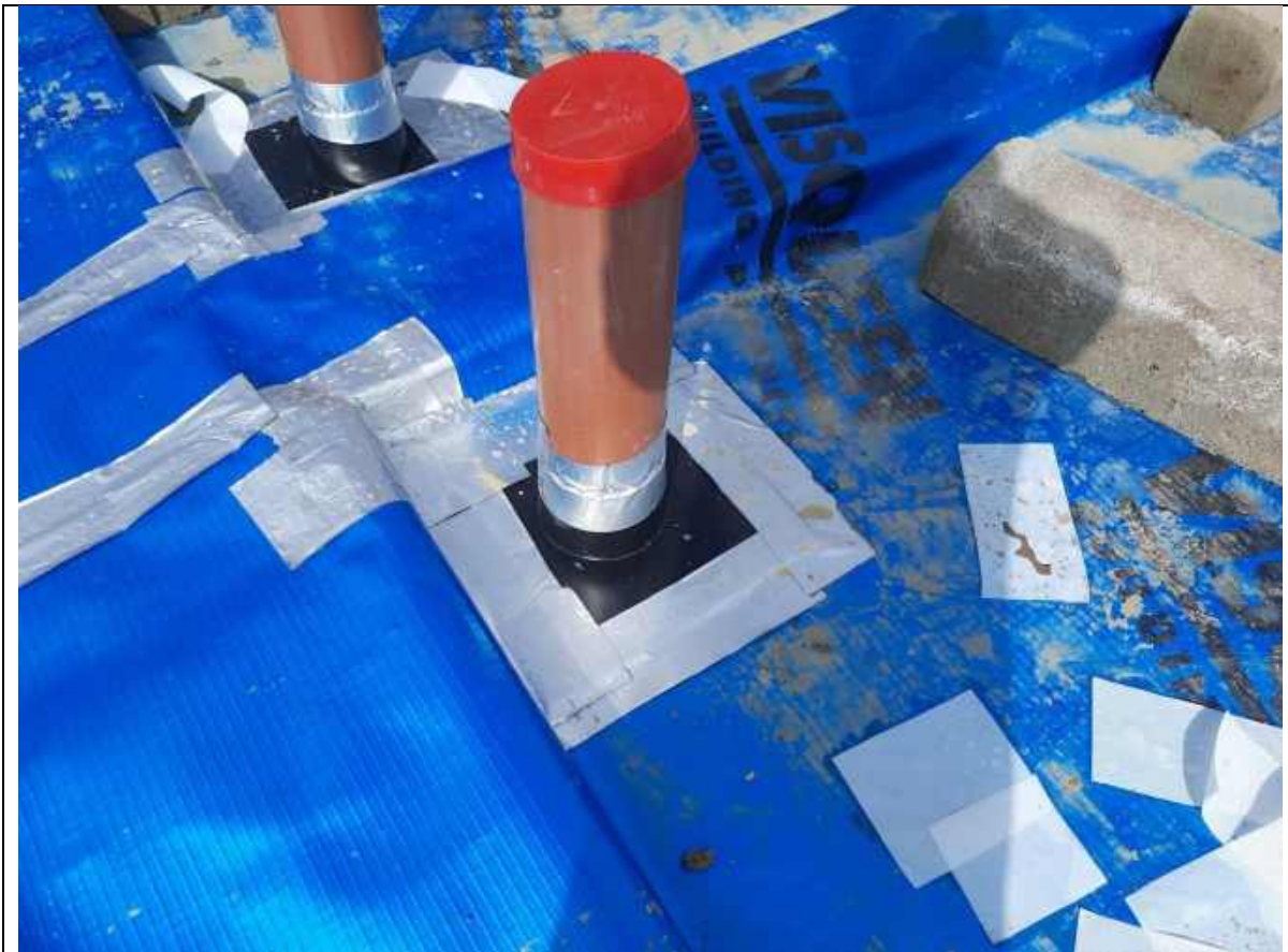
Plate 42: Showing a preformed tophate using Visqueen detailing tape on Plots 11-12
