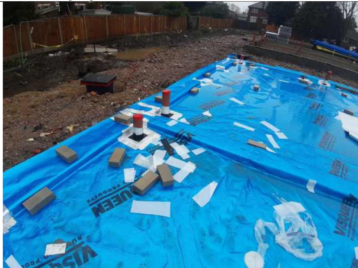
Plate 39: Showing the general condition of the membrane on Plots 11-12
