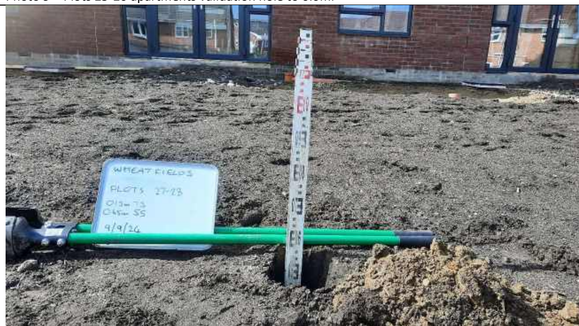
Photo 10 – Plots 27-28 apartments validation hole to 0.6m.
