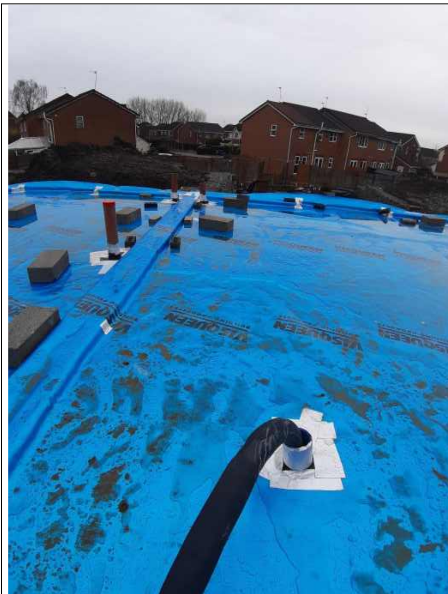
Plate 76: Showing the general condition of the membrane on Plots 23-24
