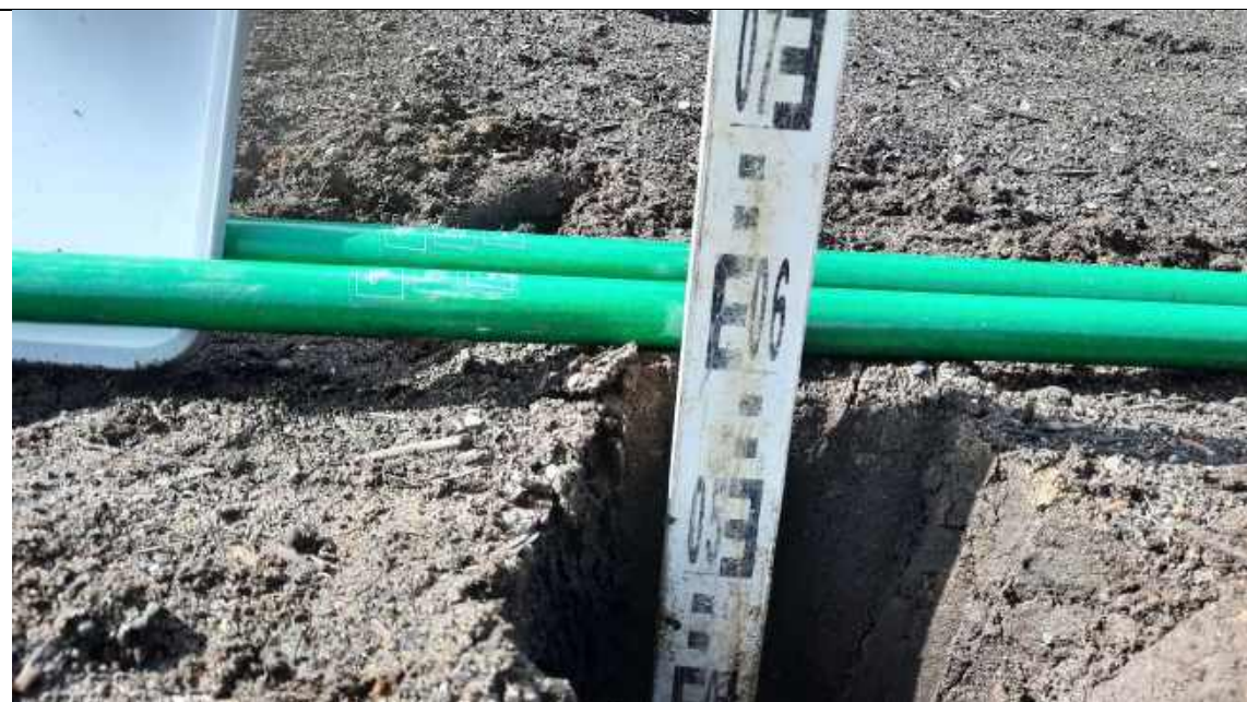
Photo 11 – Plots 27-28 apartments validation hole to 0.6m.
