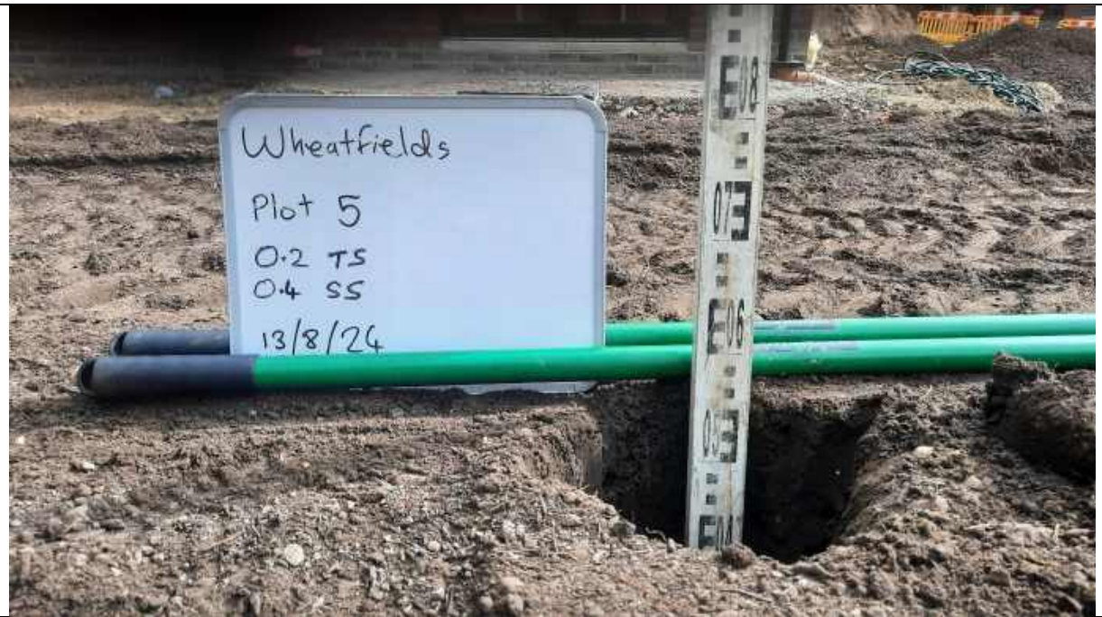
Photo 11 – Plot 5 depth validation to 0.6m.
