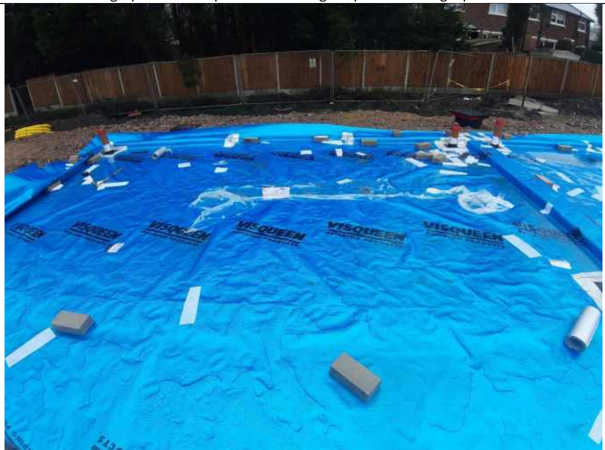
Plate 41: Showing the general condition of the membrane on Plots 11-12
