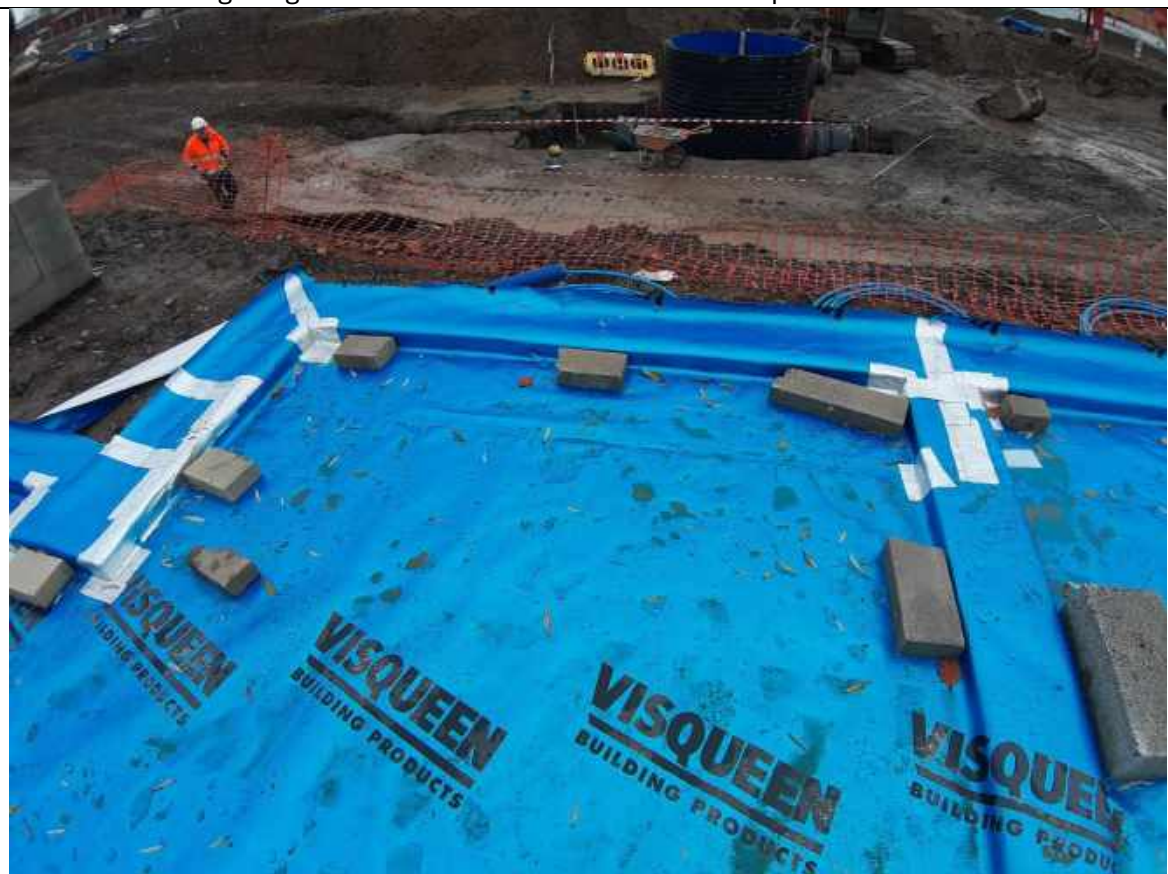
Plate 23: Showing the general condition of the membrane on plots 5&6
