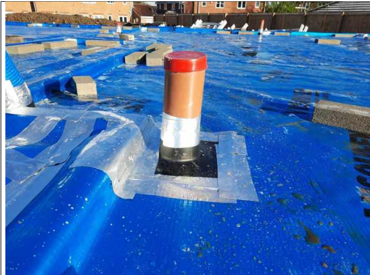
Plate 82: Showing a preformed top hat sealed with Visqueen detailing strip on Plots 25-26
