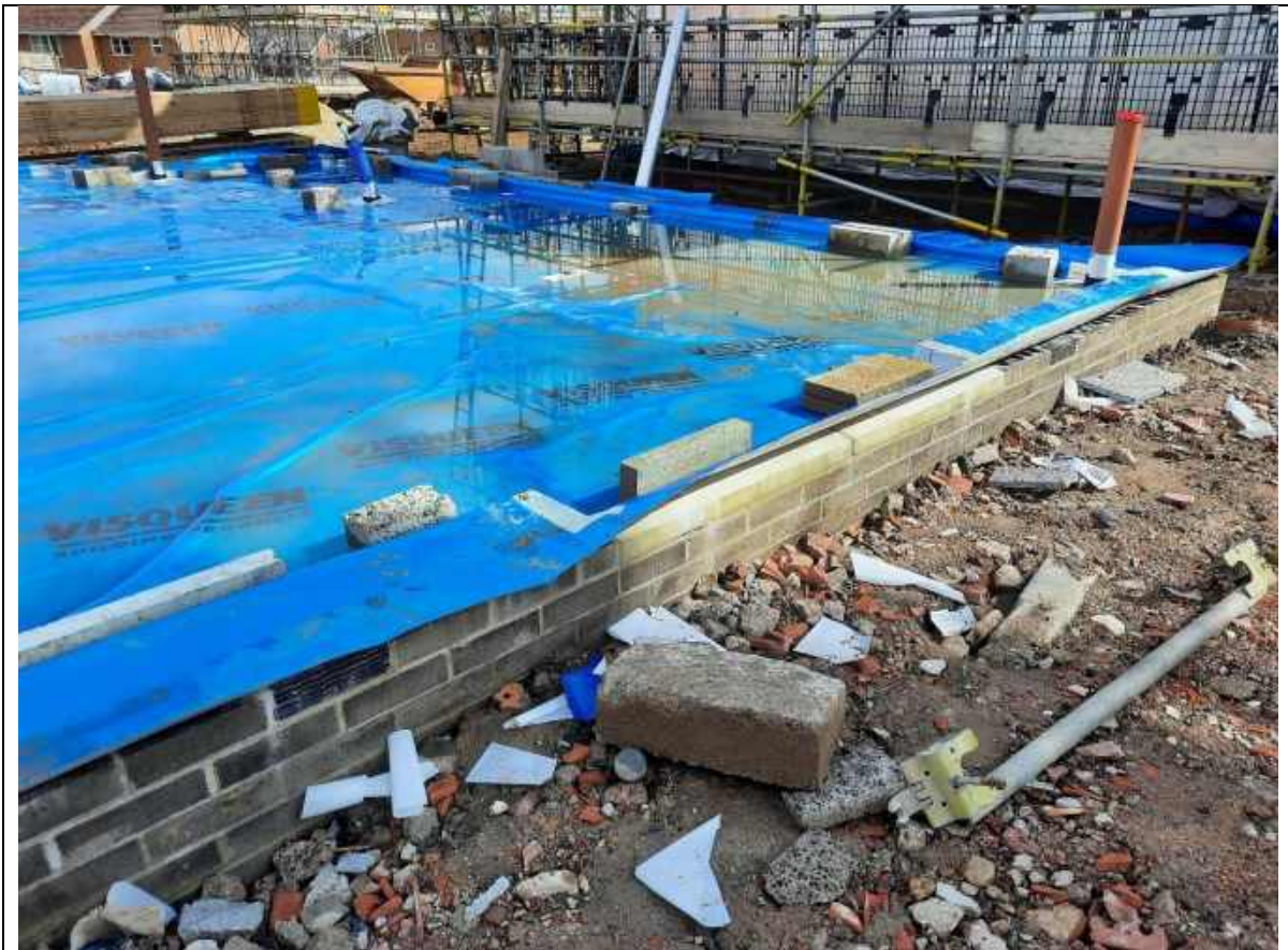
Plate 46: Showing the membrane covering the cavity wall on Plot 14
