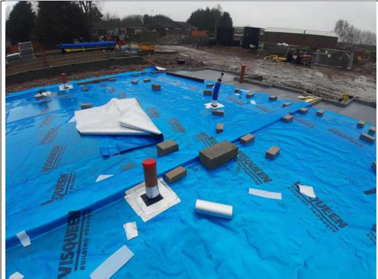
Plate 40: Showing a preformed tophat sealed using Visqueen detailing tape on Plots 11-12
