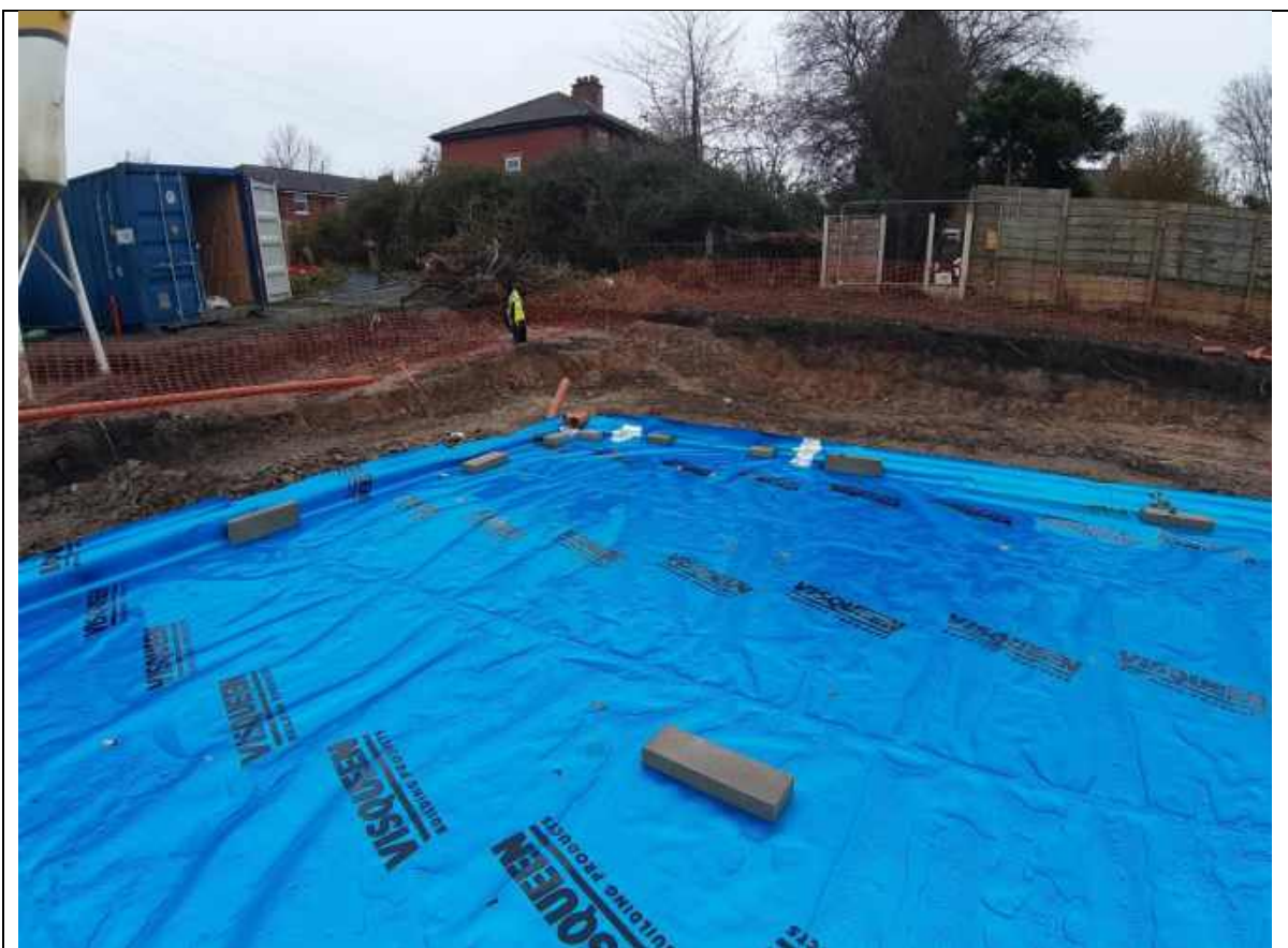
Plate 2: Showing the general condition of the gas membrane on plot 1
