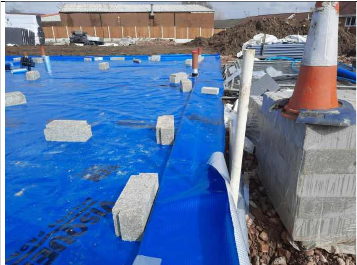
Plate 56: Showing the membrane covering the cavity wall on Plot 18
