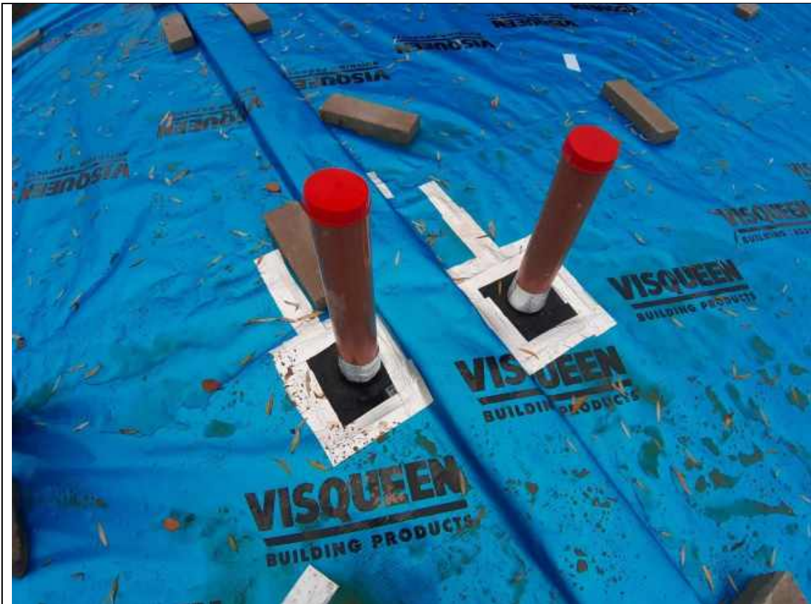
Plate 16: Showing sealed preformed top hats on plots 5-6
