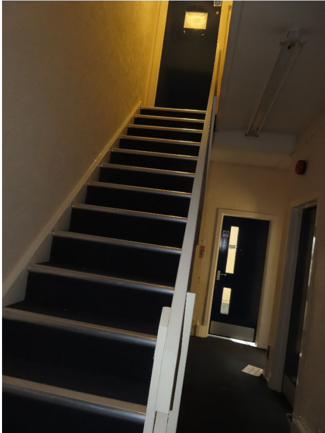
New staircase to first floor.
