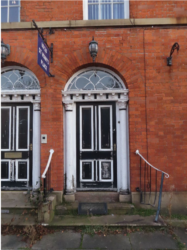
Repair to original balustrade to number 18.
