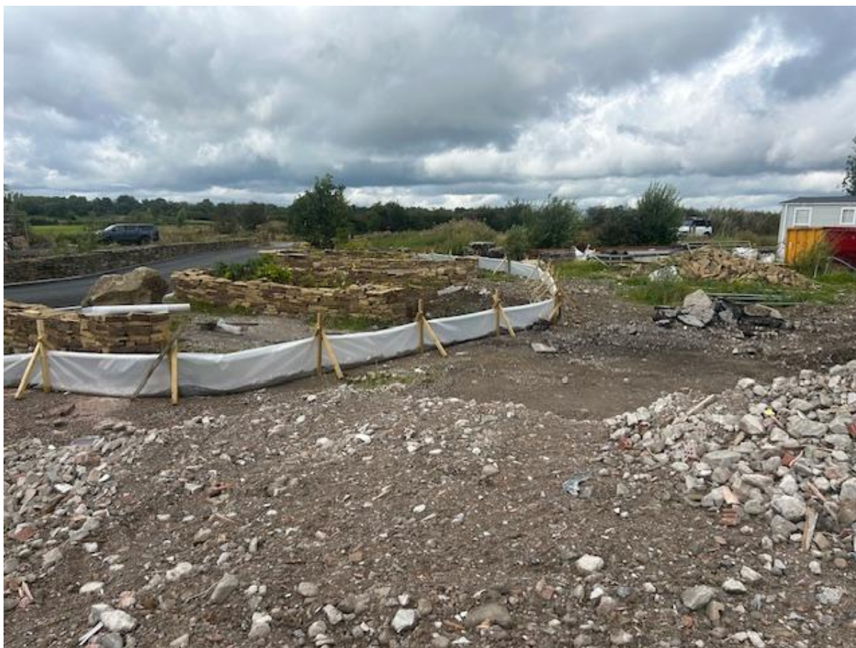
Photograph 3: Fencing located over hard standing road surface and crushed brick / concrete
