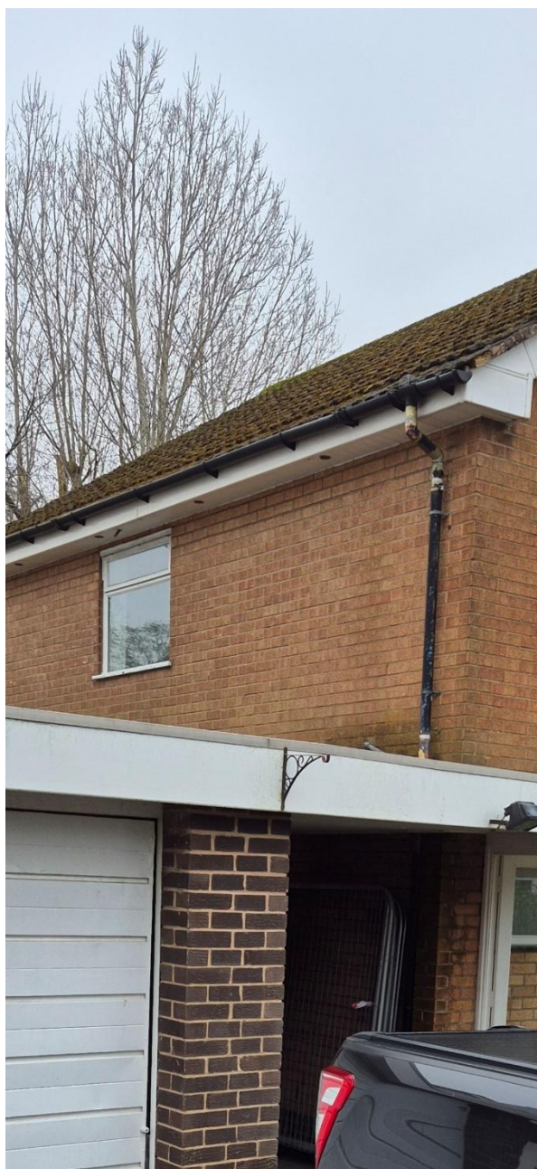
Photograph 2: Northern aspect of the dwelling showing roof, fascia boards and soffits in good repair.
