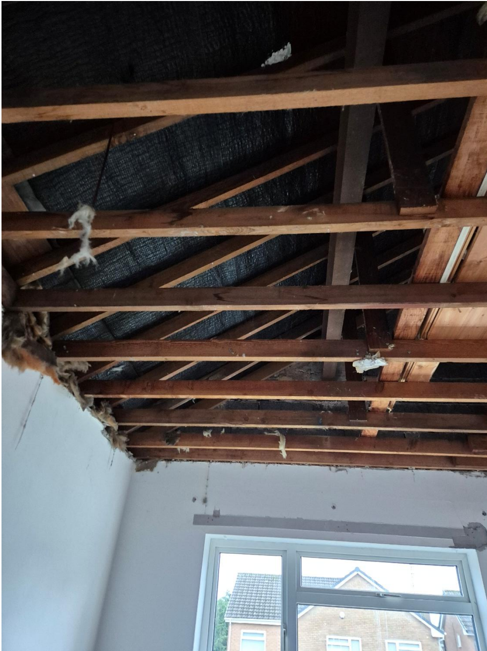
Photograph 4: Exposed loft insulation and wooden support beams.
