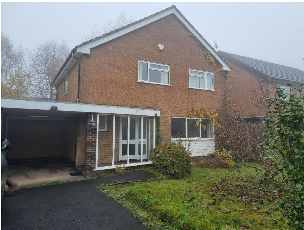
Photograph 1: Dwelling with fascia boards and PVC windows visible (western aspect)
