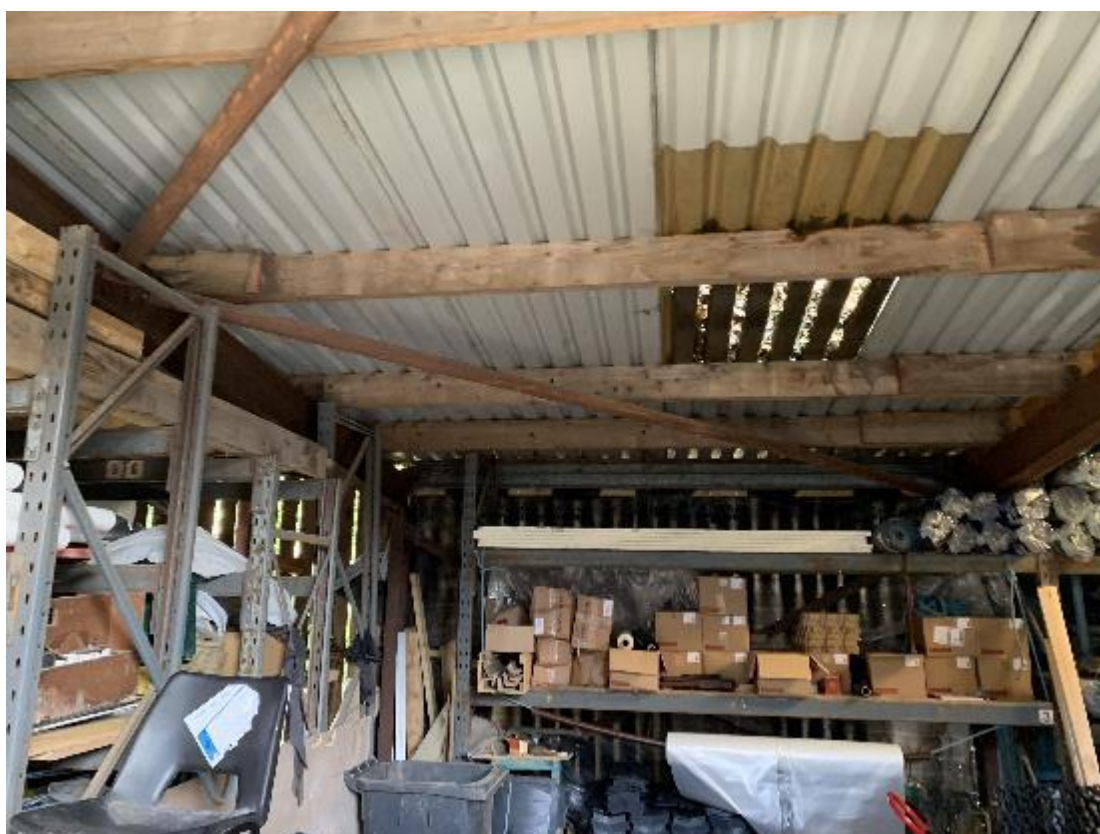
Plate 22 – Internal character of B2, showing use as storage
