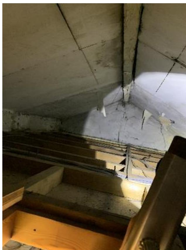
Plate 8 – Internal character of the loft space above the office section of B1
