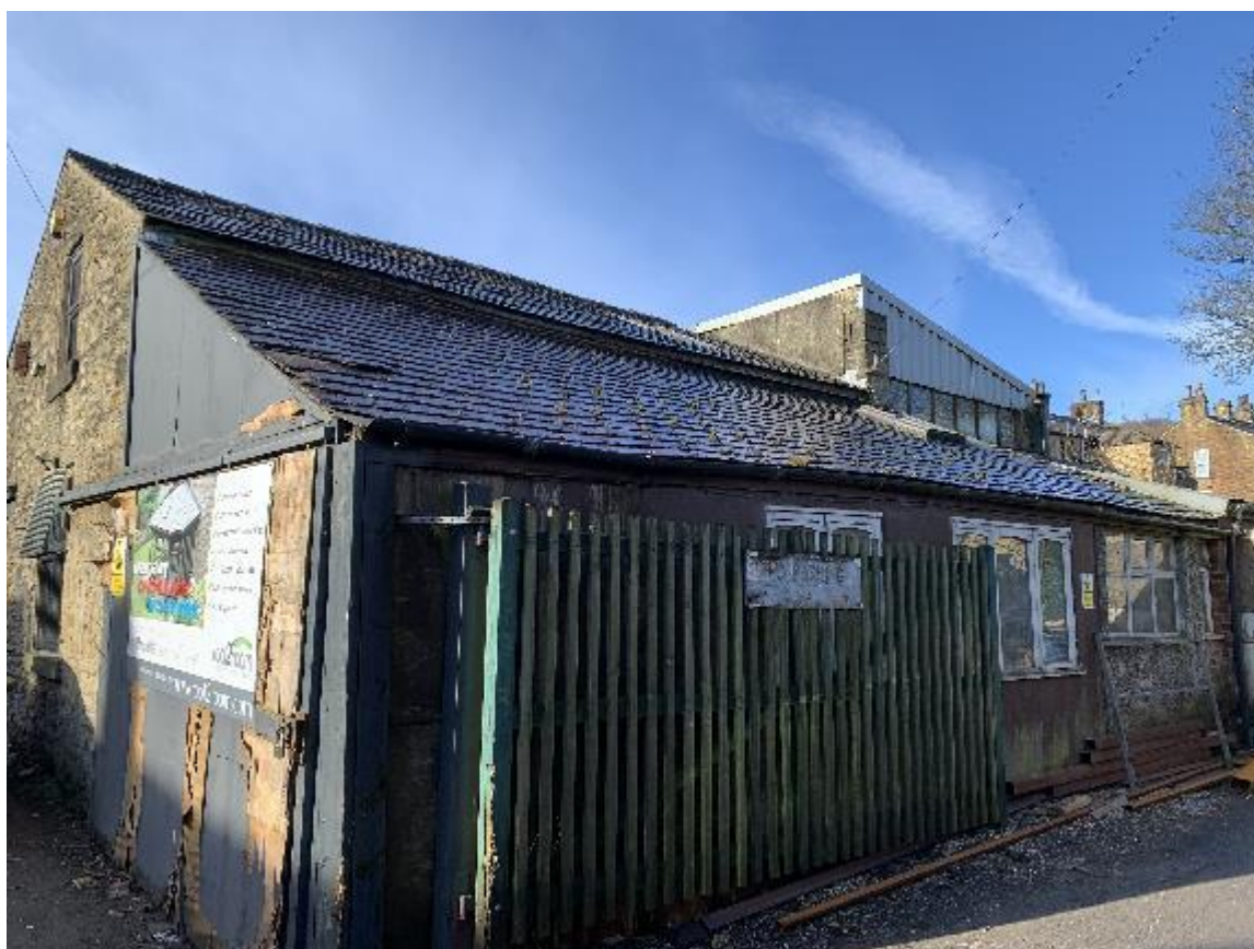
Plate 6 – North-eastern elevation of building B1
