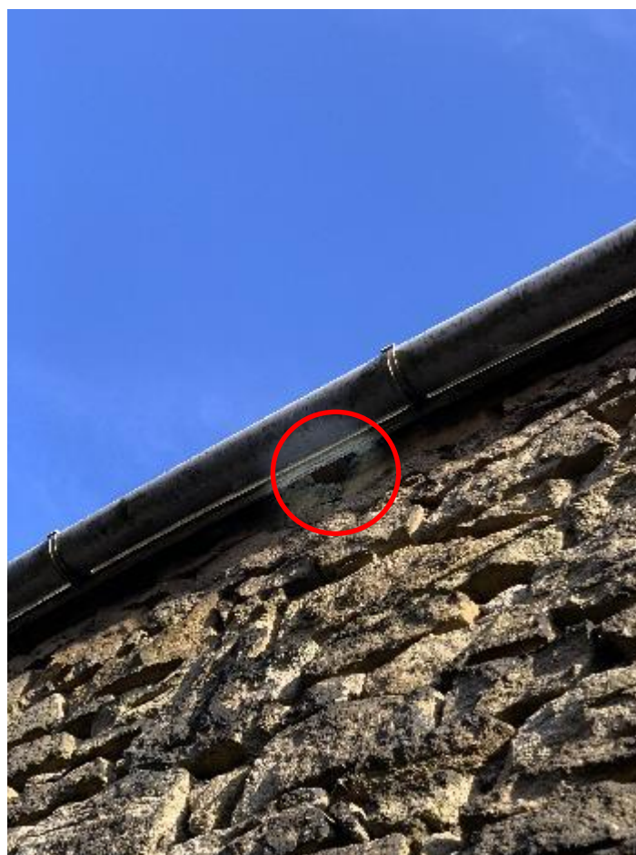
Plate 4 – One example of the many entry points at wall-plate level on south-western elevation
