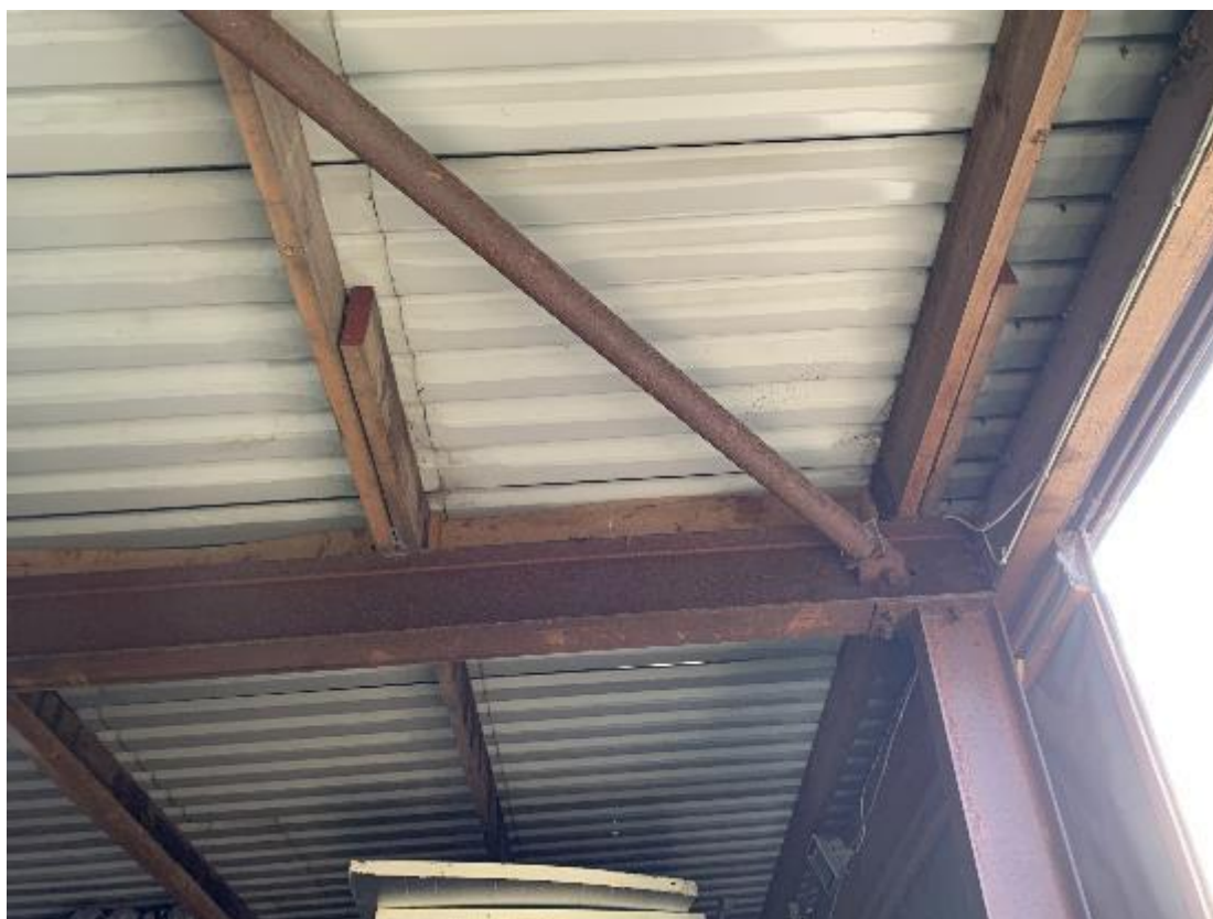
Plate 23 – Roof and building construction of B2
