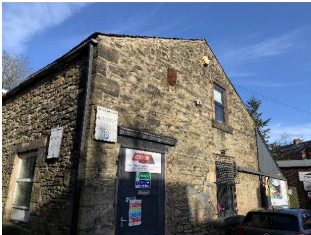
Plate 1 – South-eastern elevation of building B1
