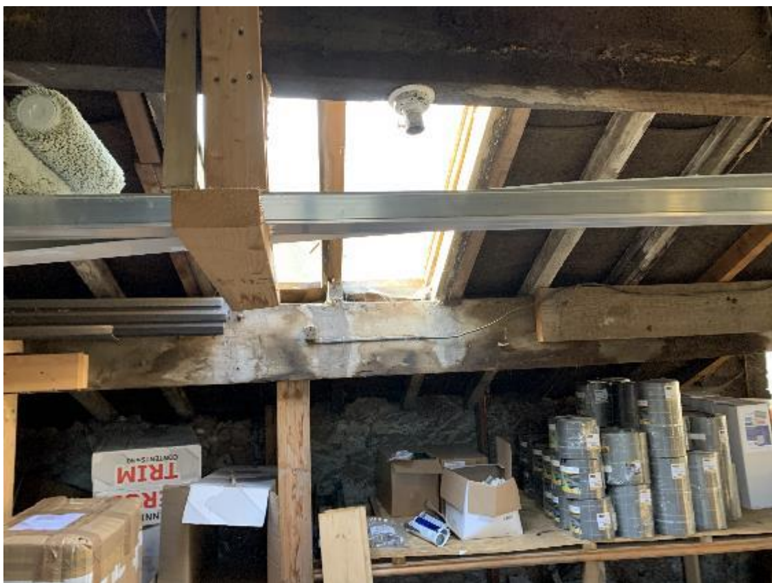
Plate 15 – Internal 'loft' space used as a wood storage
