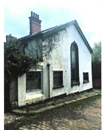
Pilsworth Cottages in the north east of Unsworth
