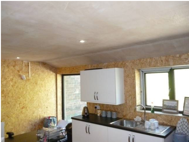
Internal second floor ceiling no loft space.
