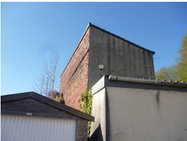
General view from the north east.
