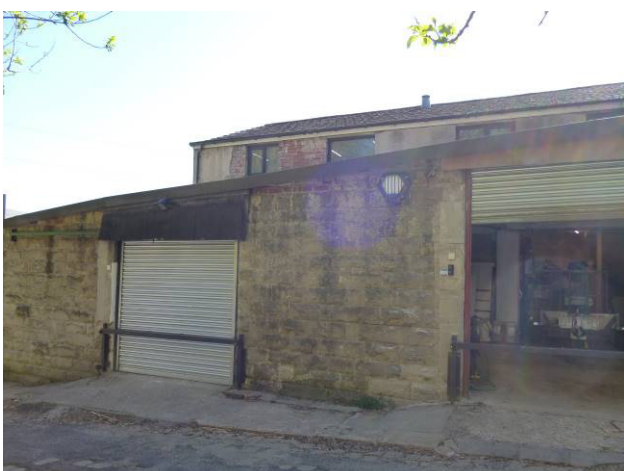
Western elevation viewed from Paradise Street.
