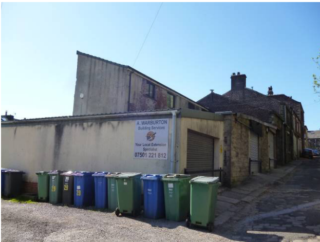
General view from the north.
