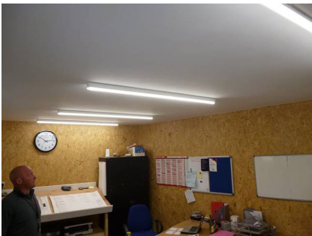
Internal second floor ceiling no loft space.
