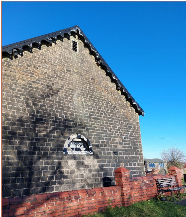
Figure 7: Southern end of the Chapel – the previous roof level and doorway can be clearly seen.
