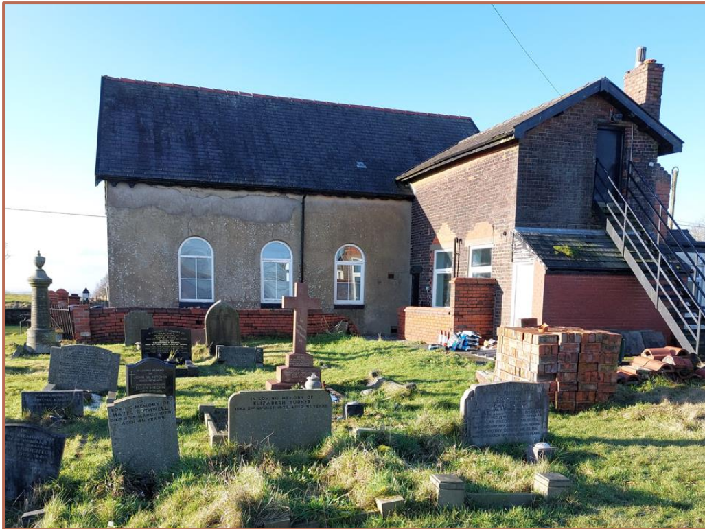
Figure 4: Photograph of Rear Elevation of Affetside Chapel
