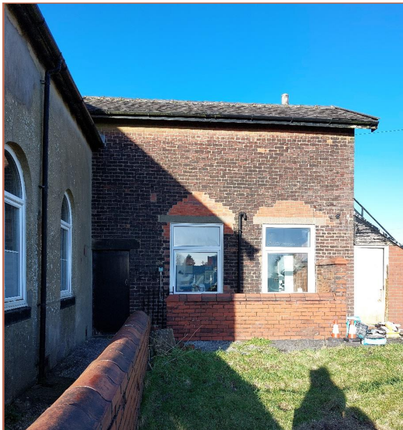
Figure 9: Rear Extension of the Chapel
