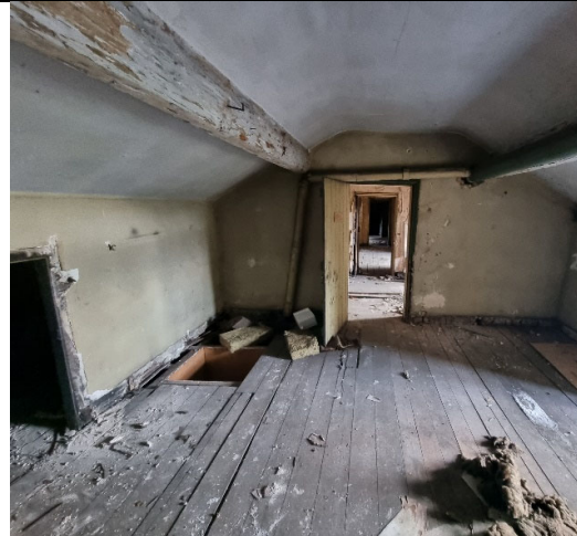
PHOTOGRAPH 6 (Above) – Timber roof purlins spanning between gable walls to intermediate masonry spine walls at second floor level
