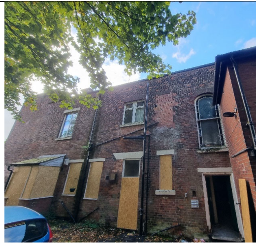
PHOTOGRAPH 4 (Above) – Partial rear elevation
