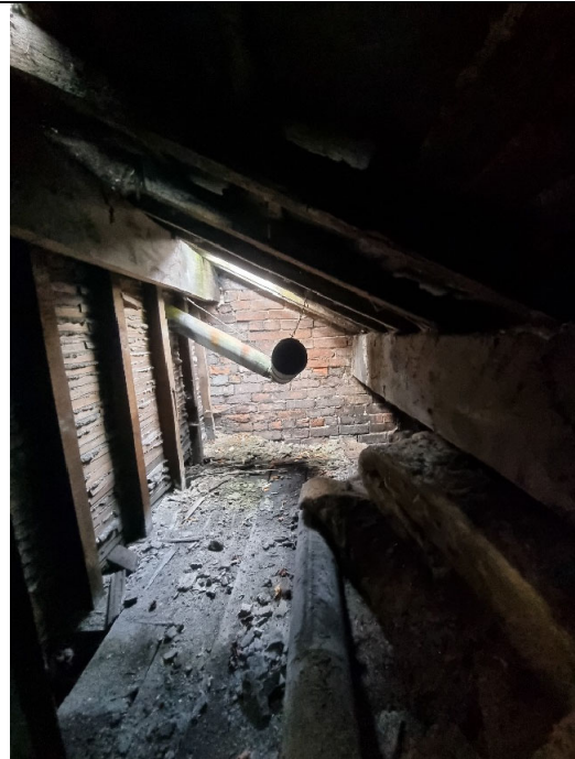
PHOTOGRAPH 8 (Above) - Typical roof construction with timber purlins and rafters. Note area of natural light leaving the 2 nd floor joists open to the element.
