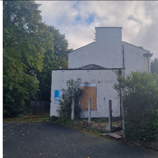
PHOTOGRAPH 2 (Above) – Left hand gable elevation and single storey extension finished in painted sand/cement render. Note chimney stack.
