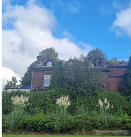
PHOTOGRAPH 1 (Above) – Front elevation with dense vegetation. Note single storey (white) extension to the left and two storey extension to the right with different bricks from that of the original building.
