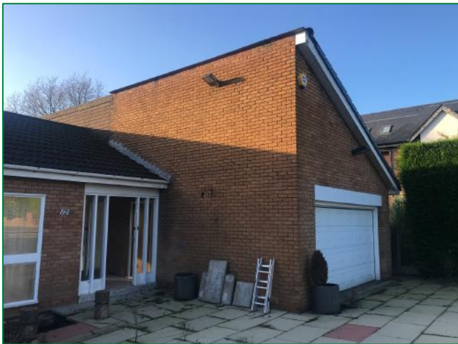
The west elevation of the property
