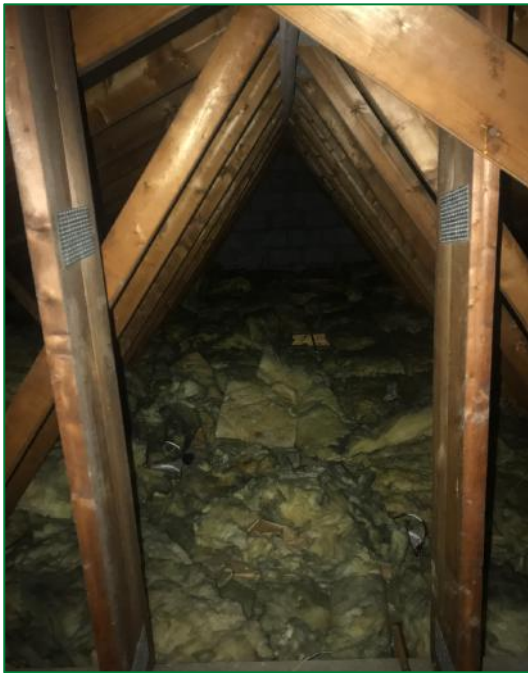
The loft void in the house
