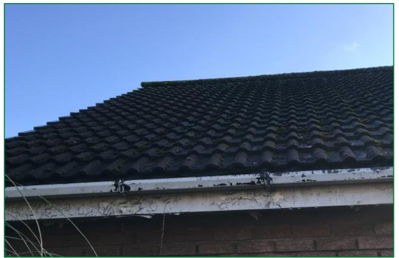
Tight-fitting tiles on the north elevation
