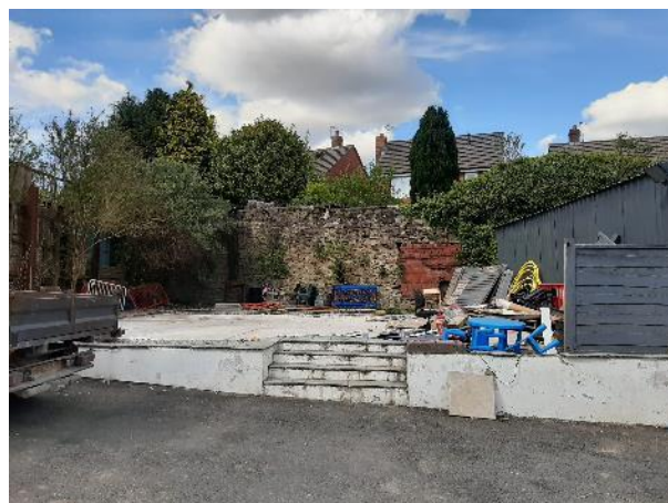
Figure 3 - Looking north showing the flat concrete plinth in the northern site section and the retaining wall on the northern boundary.
