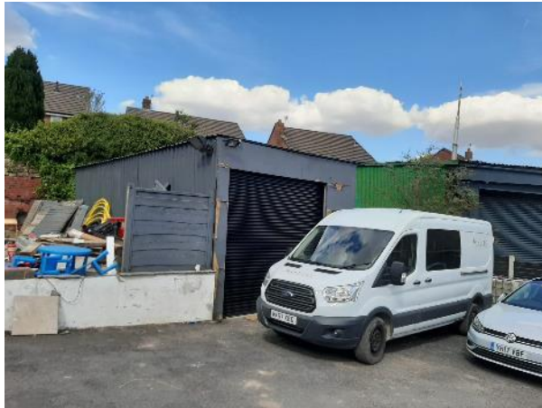
Figure 4 - Looking north east showing one of the two site buildings.
