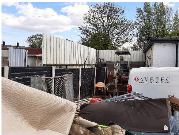
Figure 6 - Looking south towards the south eastern site corner. Plant is stored and materials are stored / tipped.
