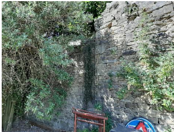
Figure 8 - Looking north west at the north western site corner. The retaining wall is of stone construction and many plants are growing on / out of it.
