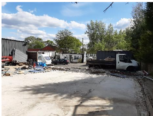
Figure 9 - Looking south east showing a general view of the site from the north west site corner.
