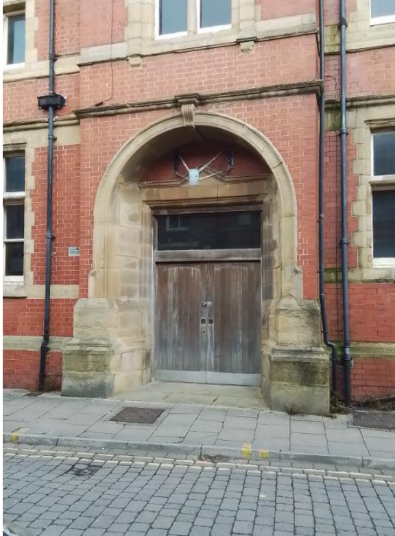
Figure 12 – Existing Front Door
