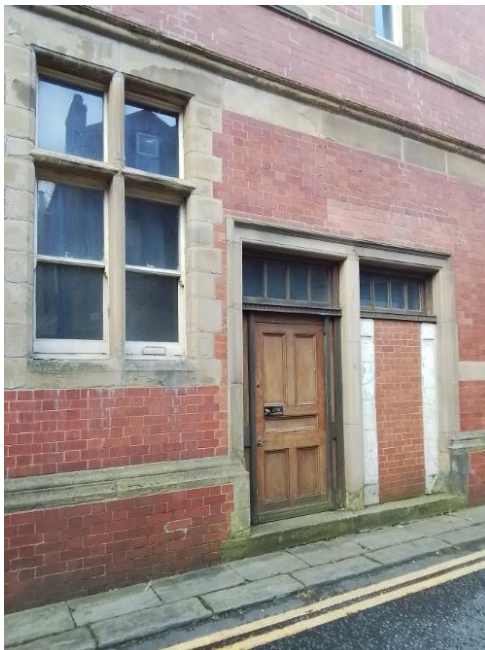
Figure 15 – Bricked up door to be replaced with a window on Back Rock
