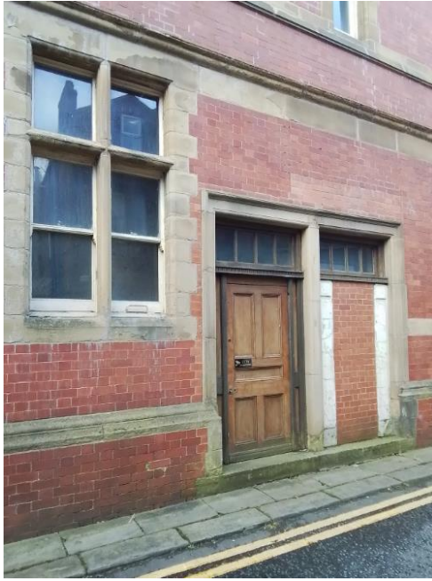
Figure 10 – Bricked up door to be replaced with a window on Back Rock
