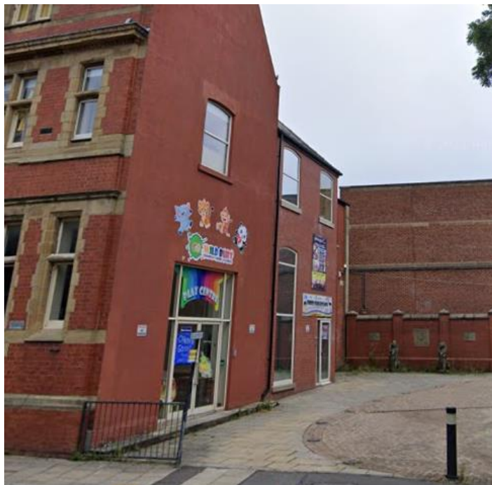
Photo 1 – Grey window frames opposite the Site
