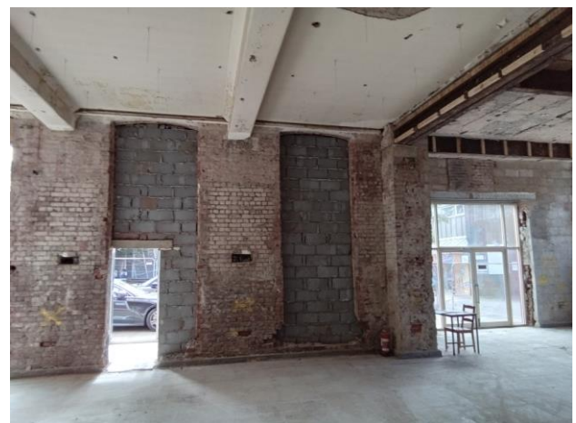
Photo 1 – Original windows shown internally and bricked up.
