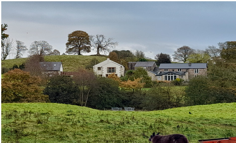
Shaunings Cottage (to the right) from the west, with the site to the right hand gable.
