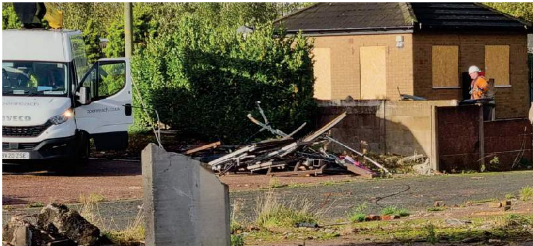
Figure 6: 26/10/22 – Openreach engineers on site disconnecting remaining services
