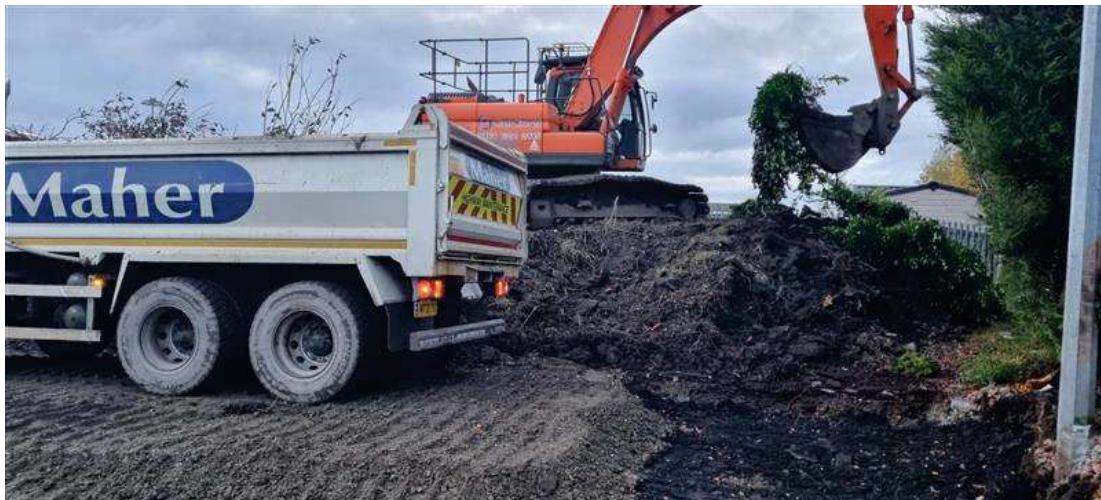
Figure 27 5/12/22 – Loading green waste/vegetation strip materials for disposal
