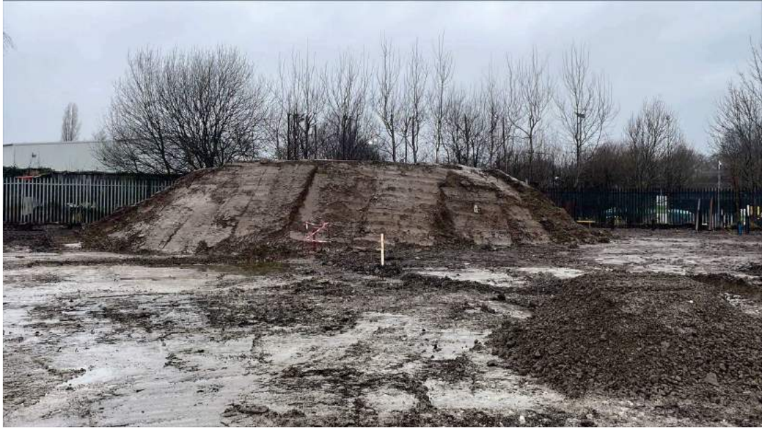
Figure 47: 3/02/23 – Western stockpile of clean certified subsoil (Stockpile 5)
