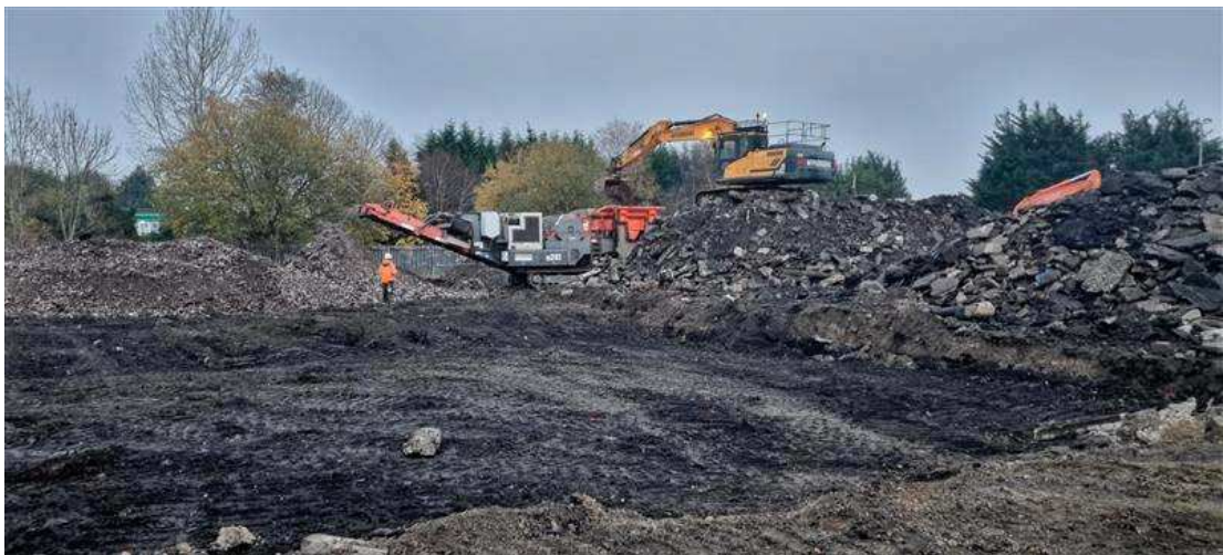
Figure 26 1/12/22 – Crushing stockpiled oversized materials
