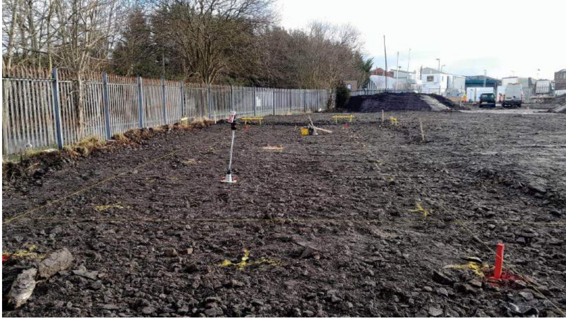
Figure 45 : 27/01/23 – Lightweight Deflectometer testing on completed pile mat
