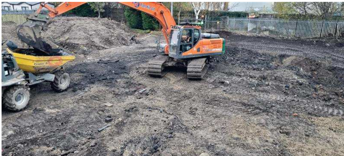
Figure 24 30/11/22 – Lifting and stripping hardstanding
