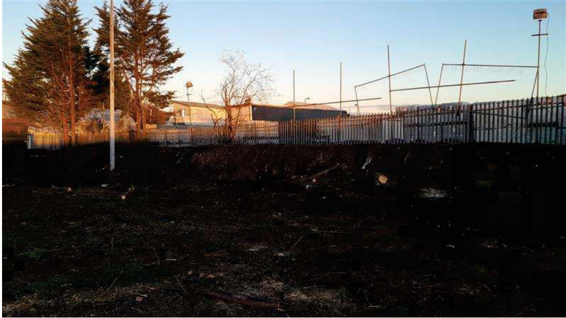
Figure 29 : 7/12/22 – Treefelling works almost complete
