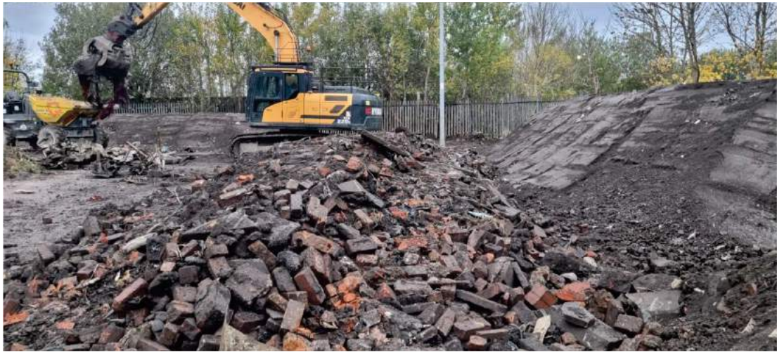
Figure 15 : 10/11/22 – Separating waste from oversize
