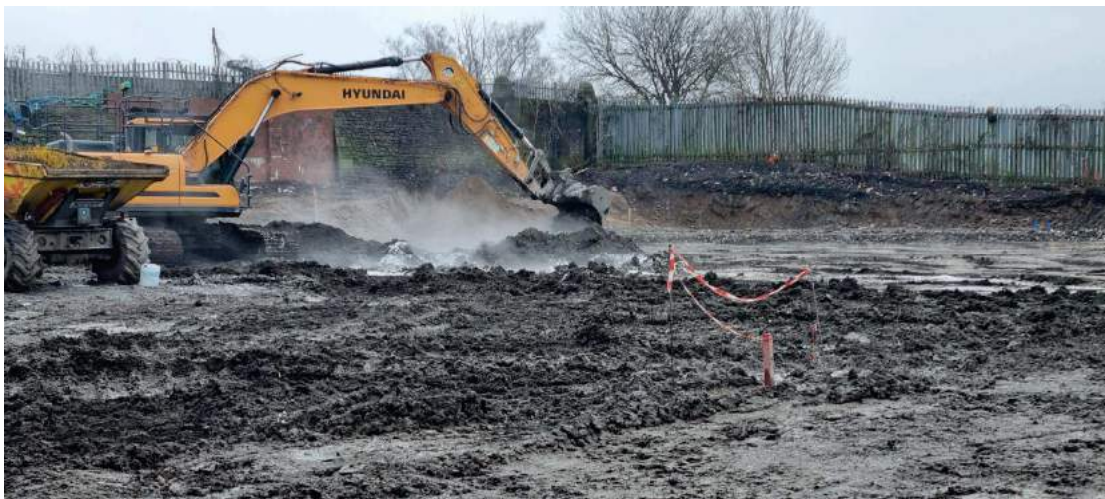
Figure 38: 17/01/23 – Using the granulated lime to reduce the free moisture content of fill material
