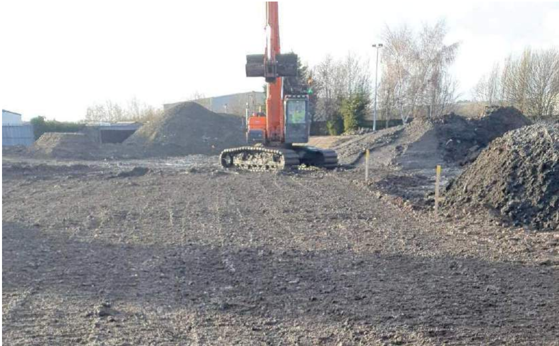
Figure 35 : 29/12/22 – PLacement of crush to access road
