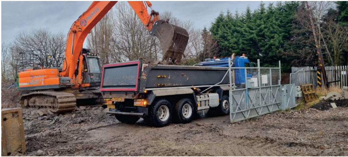
Figure 37: 12/01/23 – Disposal of last remaining oversize material
