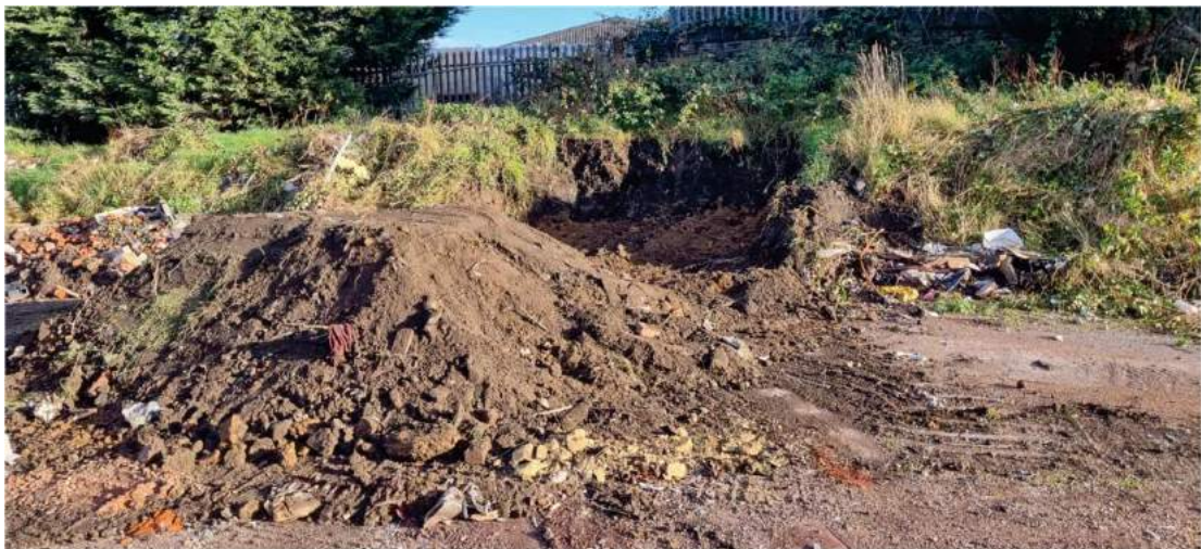
Figure 10: 4/11/22 – TP512 stockpiled on hardstanding ahead of removal from site to a licensed landfill
