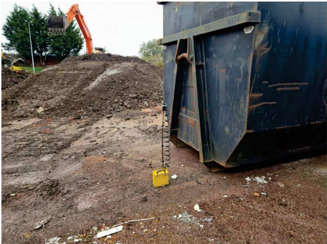
Figure 16 : 10/11/22 & 11/11/22 – Background (reassurance) air monitoring in progress around site boundary during riddling activities
