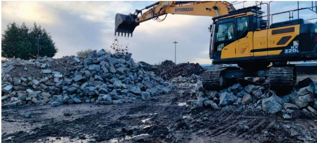
Figure 19: 16/11/22 – Oversize stockpile management
