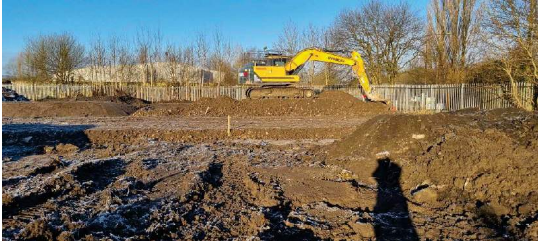
Figure 41 : 23/01/23 – Placement of granular fill to plots
