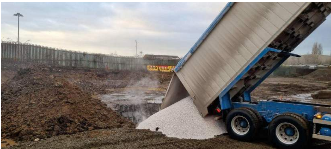
Figure 36 : 11/01/23 – Delivery of granulated lime for treatment of saturated soils
