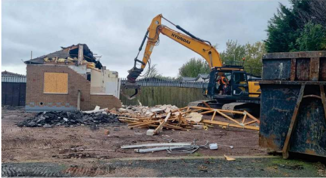
Figure 5: 31/10/22 – Ongoing demolition and disposal of segregated waste streams
