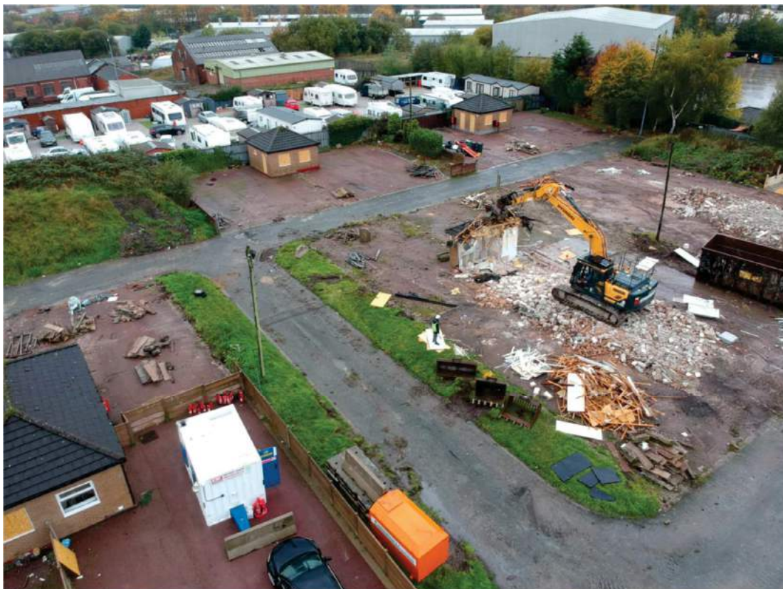
Figure 4 : 27/10/22 - Excavator demolishing/segregating materials from central building
