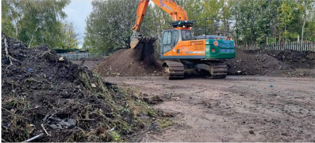
Figure 11 : 8/11/22 – Riddling material from perimeter bund to remove oversize for subsequent processing
