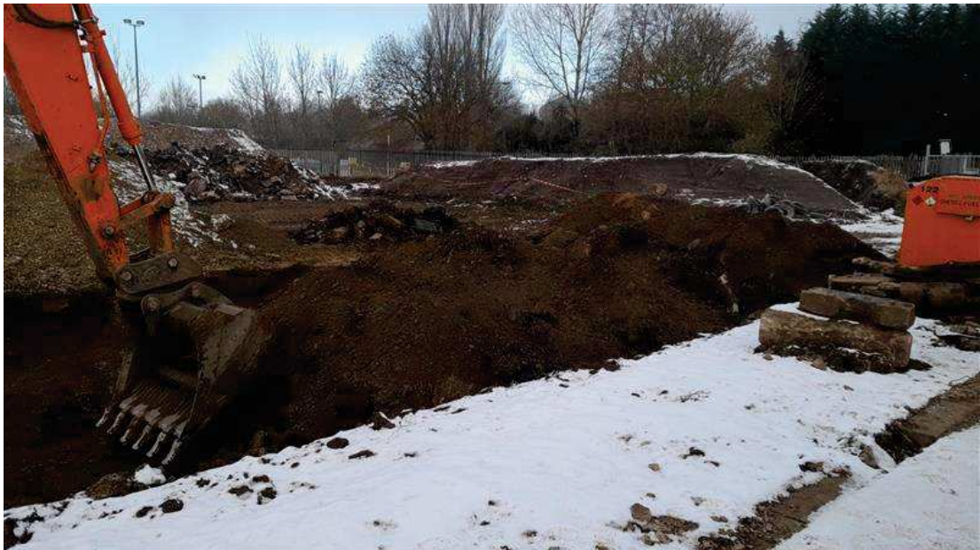
Figure 30 : 12/12/22 – Turnover under main access road
