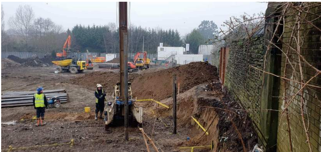
Figure 42 : 24/01/23 – Piling rig at work in SE corner of the site
