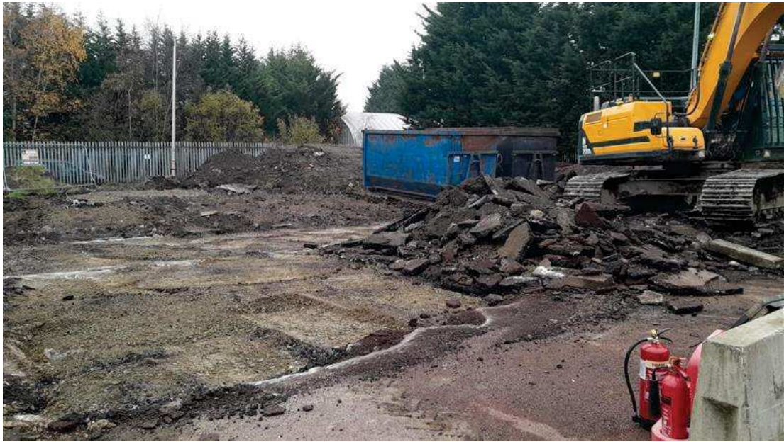
Figure 25 : 1/12/22 – Lifting and stripping areas of tarmac surfacing
