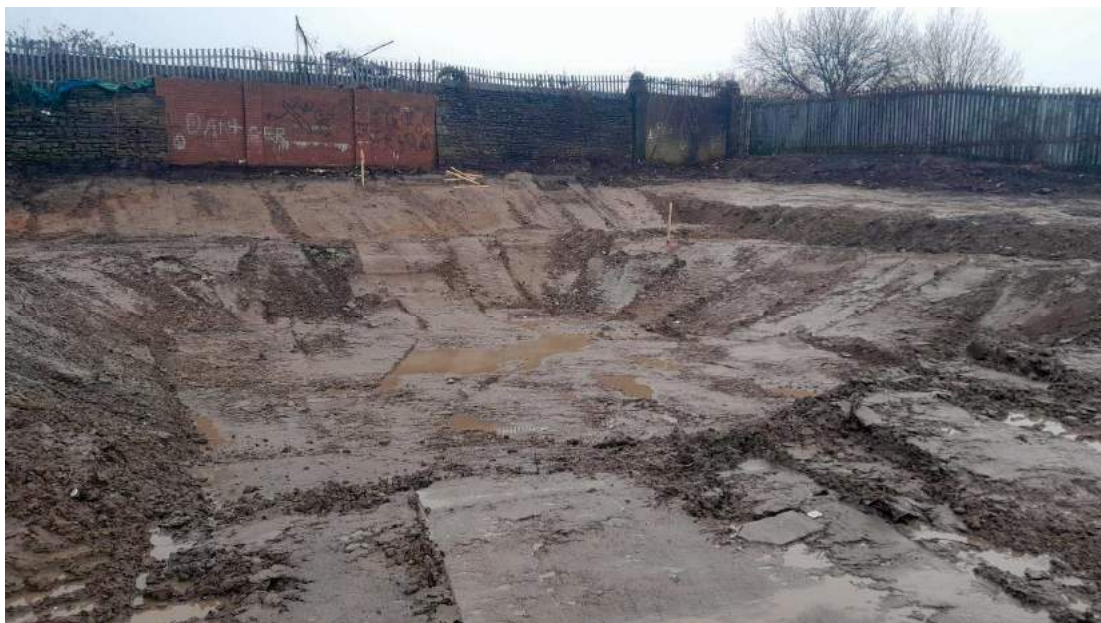
Figure 34 : 23/12/22 – Completed excavation for subsoils
