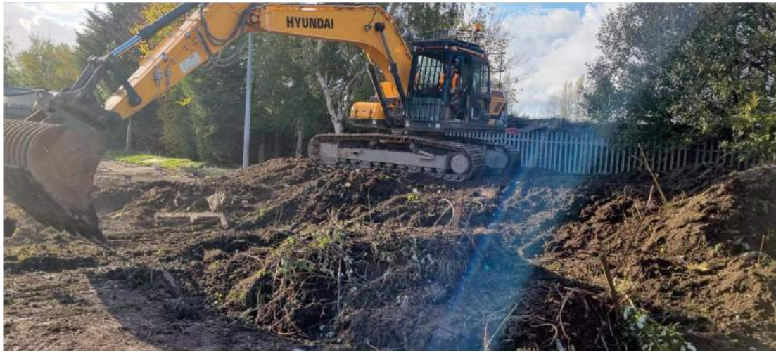
Figure 7: 3/11/22 – Vegetation scrape and segregation of green waste
