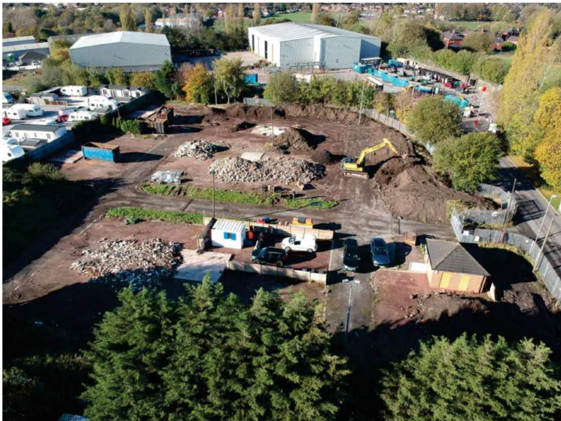
Figure 8: 4/11/22 – Stockpile management/removal of contamination hotspot (TP503) ahead of delineation
