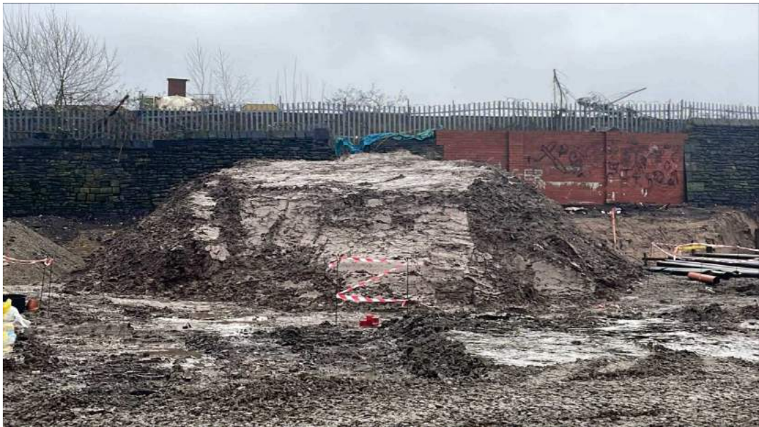
Figure 48 : 3/02/23 – Eastern stockpile of clean certified subsoil (Stockpile 6)
