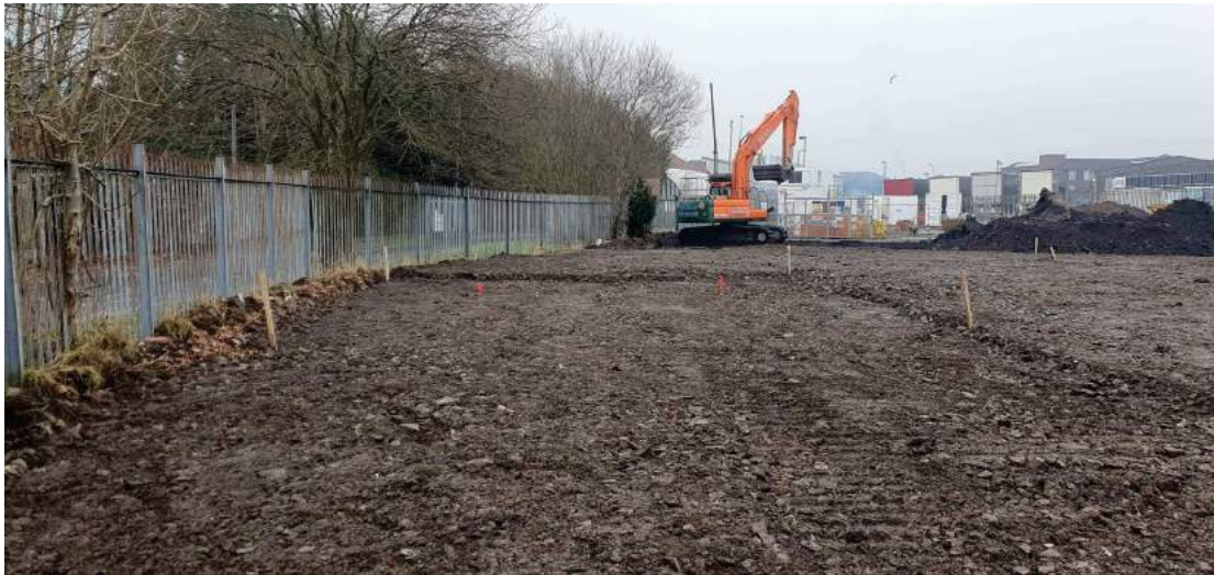
Figure 44 : 24/01/23 – Completed plot in NW of site
