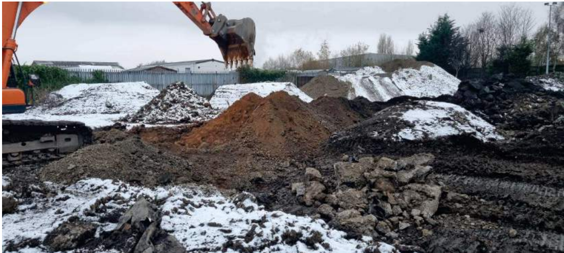
Figure 32 : 13/12/22 – Segregation of materials into stockpiles
