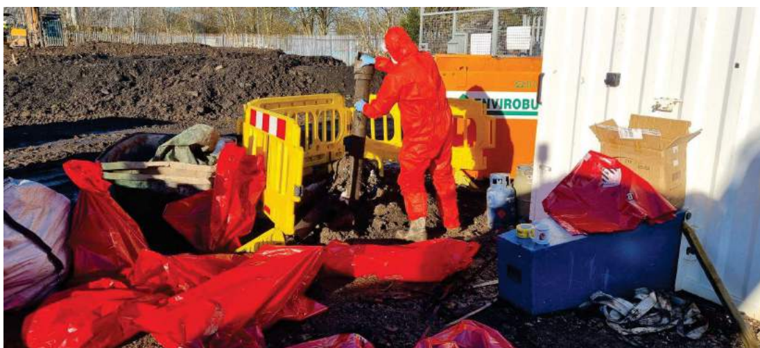
Figure 40 : 23/01/23 – Double-bagging of asbestos-cement pipes prior to removal from site
