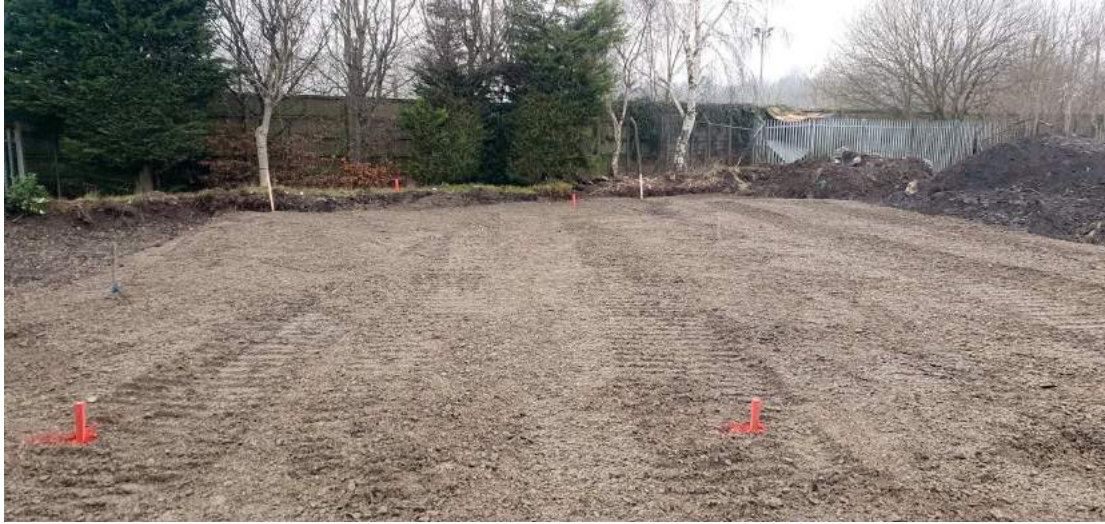
Figure 43 : 24/01/23 – Completed plot in SW of site
