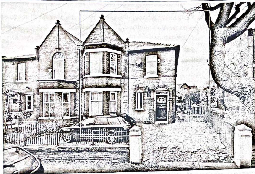
A view of the front of the site
