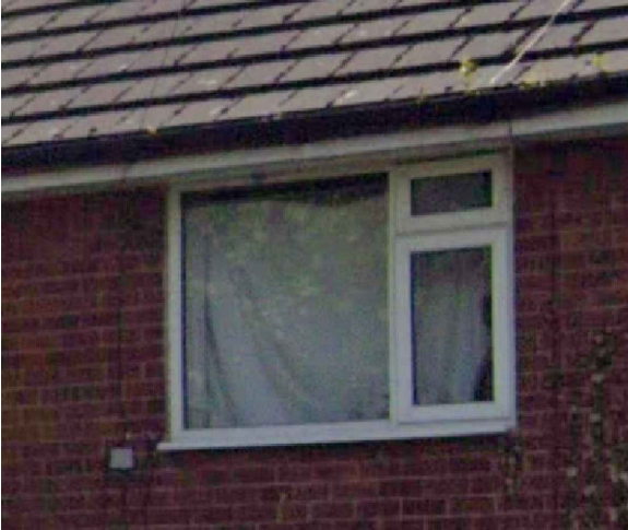
uPVC Windows to match adjacent properties
