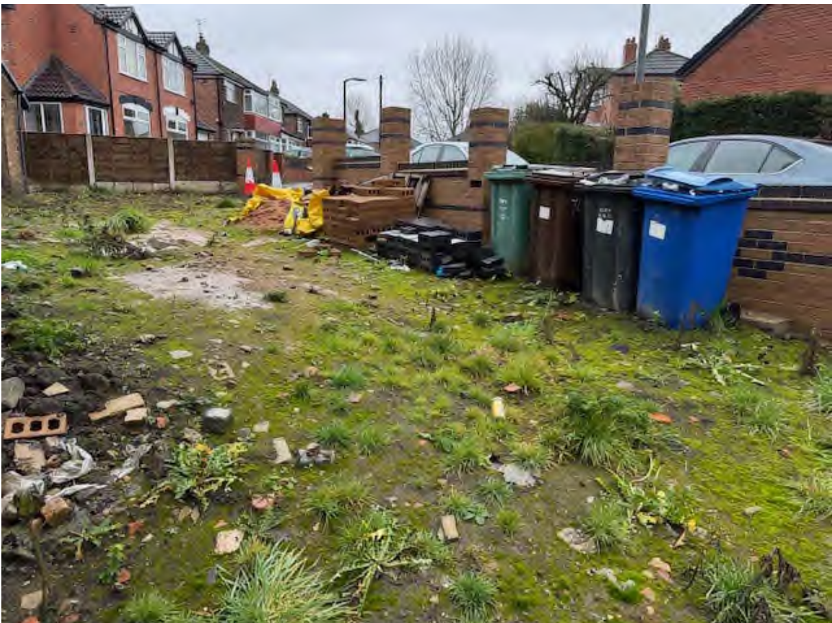
Photograph 4 - Bins & Construction Materials Adjacent to Edgeware Avenue Boundary
