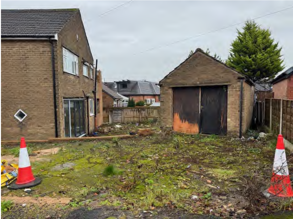
Photograph 5 - Existing Garage, Accessed from Edgware Avenue
