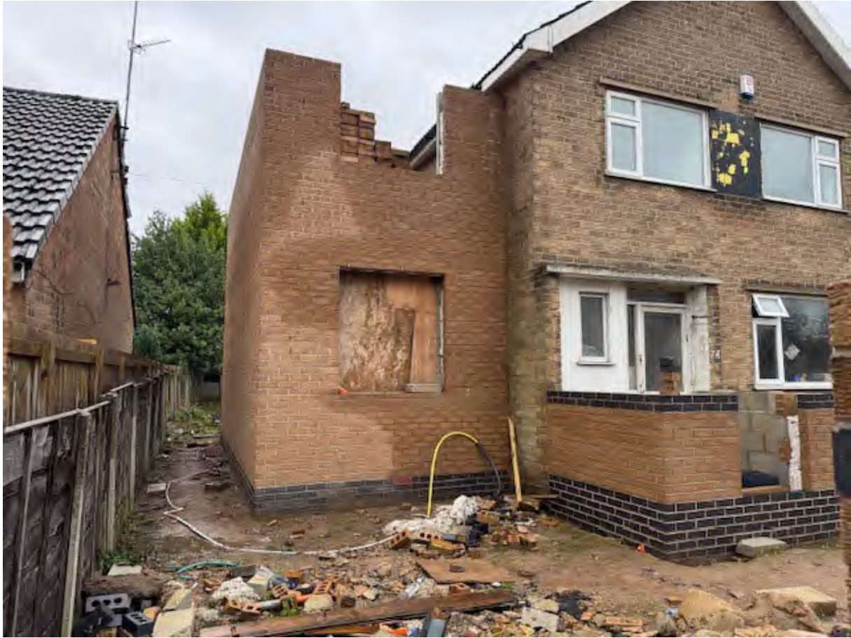
Photograph 7 - Partially Constructed 2-Story Side Extension
