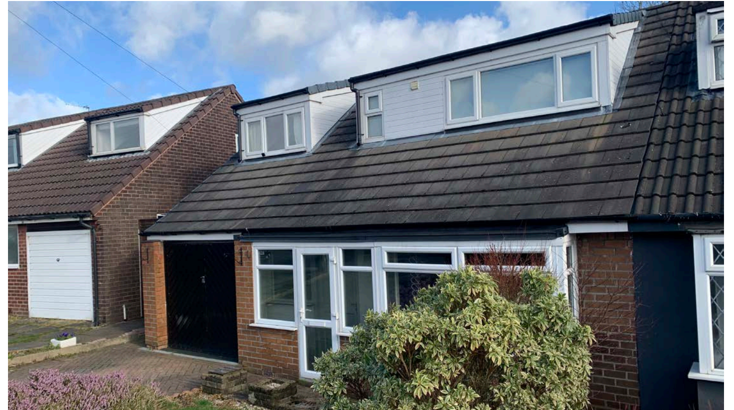
Above: Existing House - Front
