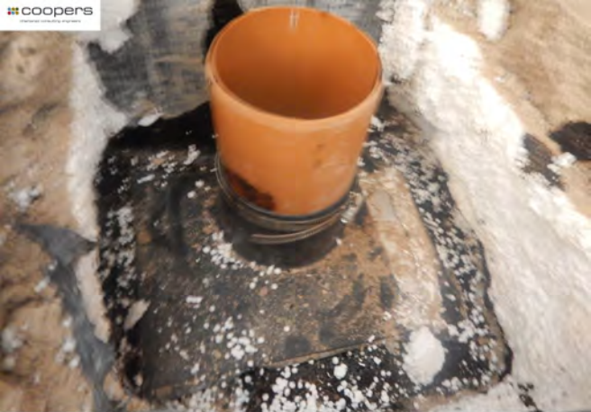
Tophat repair inspected by Coopers, in addition to inspection carried out on site by Kier Living. Photograph dated 1st August 2017.
