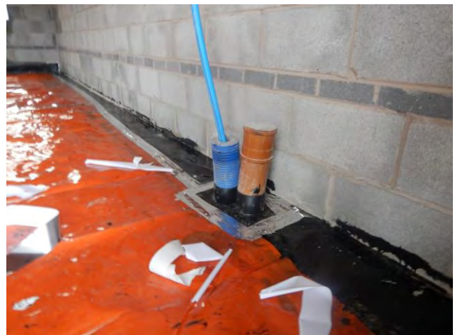
Photograph 18: Showing the typical installation of a preformed tophat using butyl and silver joining tape on Plot 15-17 during inspection on 29 th June 2017.
