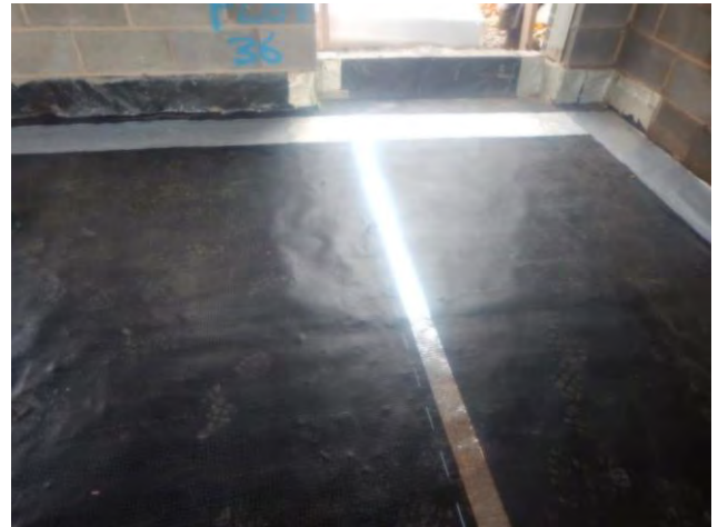
Photograph 16: Showing the general condition of the membrane installation on Plot 36 with detailing strip used to seal and join onto the perimeter during inspection on 17 th October 2017.
