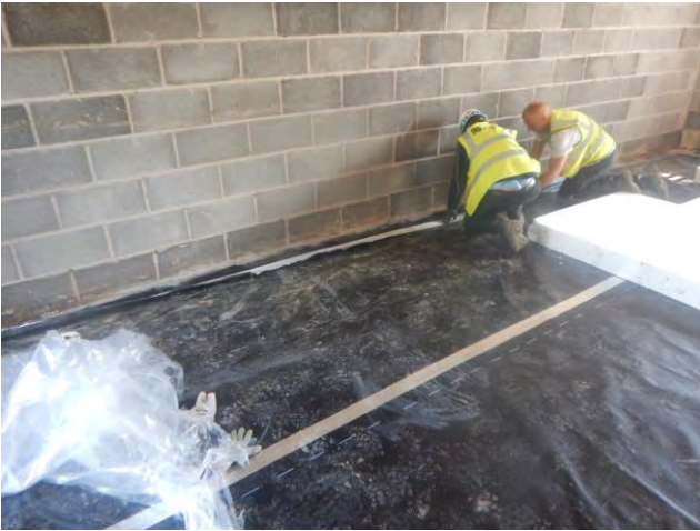
Photograph 13: Showing the general condition of the membrane installation on Plot 4 during inspection on 14 th August 2017.
