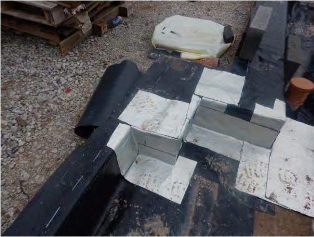
Photograph 9: Showing the first stage of membrane construction on top of the cavity wall, with corners showing sufficient seal and overlap using detailing strip and the general condition of the membrane installation on Plots 36-37 during inspection on 8 th August 2017.
