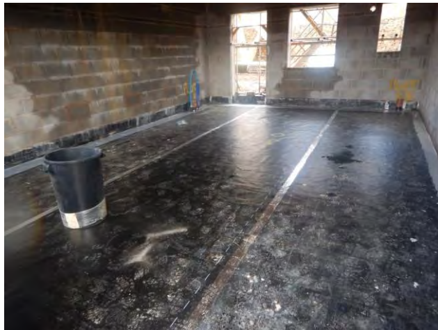
Photograph 15: Showing the general condition of the membrane installation on Plot 28 with detailing strip used to seal and join onto the perimeter during inspection on 18 th August 2017.
