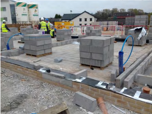
Photograph 5: Showing the first stage of membrane construction on top of the cavity wall, with corners showing sufficient seal and overlap using detailing strip and the general condition of the membrane installation on Plots 28-31 during inspection on 7 th April 2017.
