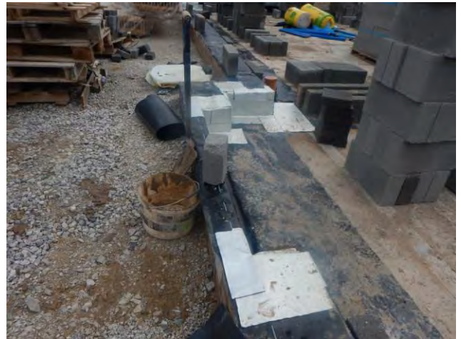
Photograph 12: Showing the first stage of membrane construction on top of the cavity wall, with corners showing sufficient seal and overlap using detailing strip and the general condition of the membrane installation on Plots 36-37 during inspection on 8 th August 2017.
