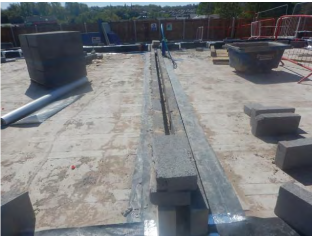
Photograph 3: Showing the first stage of membrane construction across the party walls and the general condition of the membrane installation on Plots 7-10 during inspection on 4 th May 2017.
