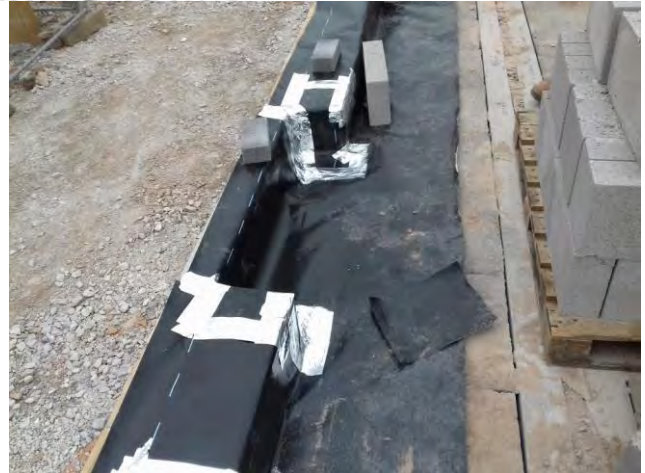
Photograph 6: Showing the first stage of membrane construction on top of the cavity wall, with corners showing sufficient seal and overlap and the general condition of the membrane installation on Plots 28-31 during inspection on 7 th April 2017.
