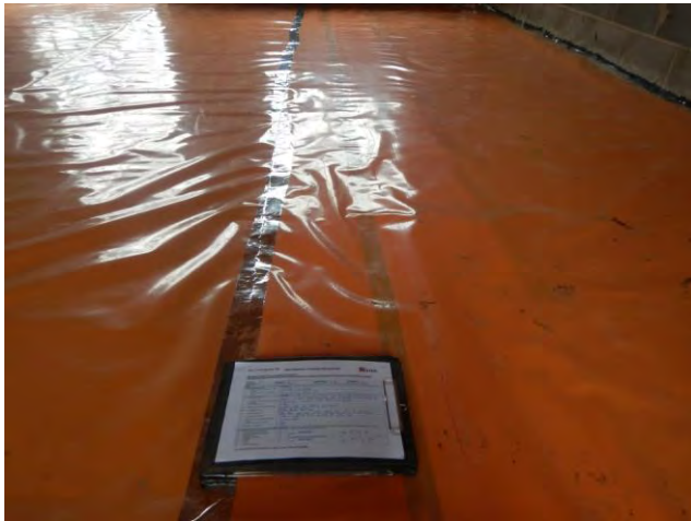
Photograph 21: Showing the jointing of two sections of membrane with greater than 150mm of overlap, sealed with butyl and silver joining tape on Plot 13 during inspection on 11 th July 2017.
