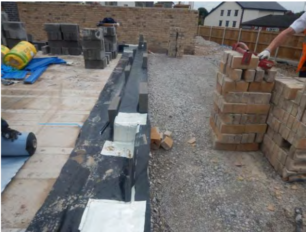
Photograph 11: Showing the first stage of membrane construction on top of the cavity wall, with corners showing sufficient seal and overlap using detailing strip and the general condition of the membrane installation on Plots 36-37 during inspection on 8 th August 2017.
