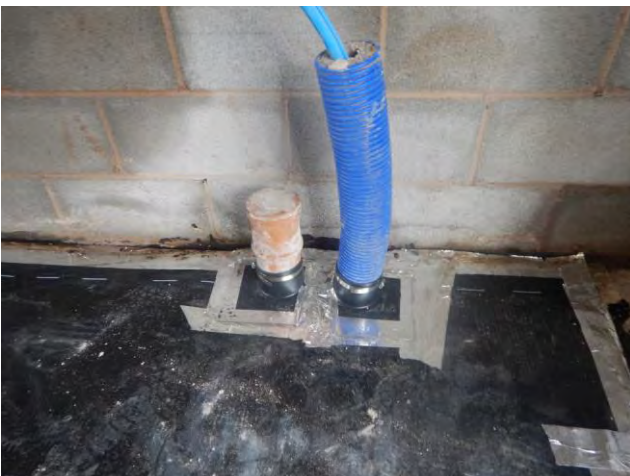
Photograph 17: Showing the typical installation of a preformed tophat using a jubilee clip, butyl and silver joining tape on Plot 33 during inspection on 31 st July 2017.
