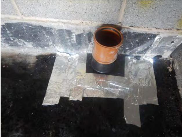
Photograph 19: Showing the typical installation of a preformed tophat using butyl and silver joining tape on Plot 9 during inspection on 27 th July 2017.
