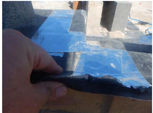
Photograph 4: Showing the first stage of membrane construction on top of the cavity wall, with corners showing sufficient seal and overlap and the general condition of the membrane installation on Plots 7-10 during inspection on 4 th May 2017.
