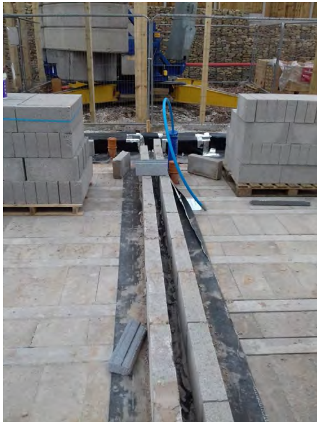
Photograph 7: Showing the first stage of membrane construction across the party walls and the general condition of the membrane installation on Plots 28-31 during inspection on 7 th April 2017.
