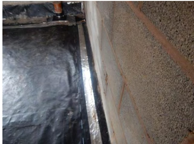
Photograph 22: Showing the membrane jointed to the perimeter stage one membrane underneath the blockwork with >150mm overlap on Plot 33 during inspection on 31 st July 2017.
