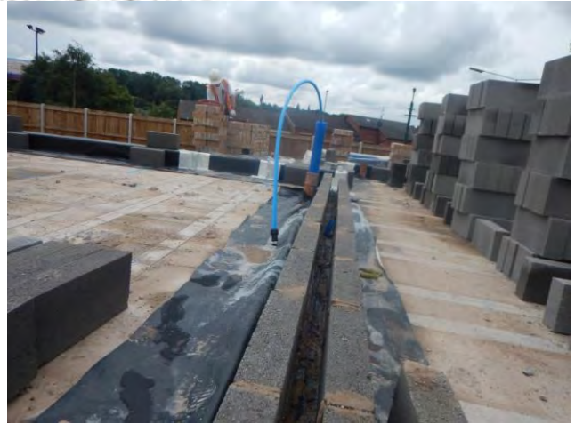
Photograph 10: Showing the first stage of membrane construction across the party walls and the general condition of the membrane installation on Plots 36-37 during inspection on 7 th April 2017.
