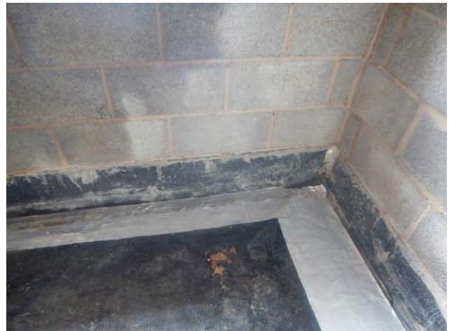
Photograph 24: Showing the membrane jointed to the perimeter stage one membrane underneath the blockwork using detailing strip with >150mm overlap on Plot 28 during inspection on 18 th August 2017.
