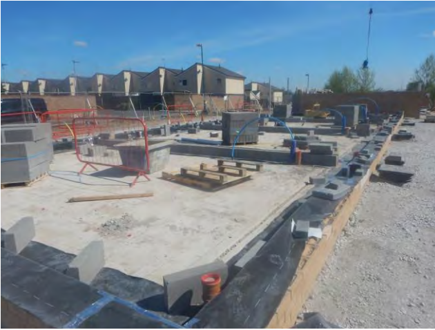
Photograph 1: Showing the first stage of membrane construction on top of the cavity wall, with corners showing sufficient seal and overlap using detailing strip and the general condition of the membrane installation on Plots 7-10 during inspection on 4 th May 2017.
