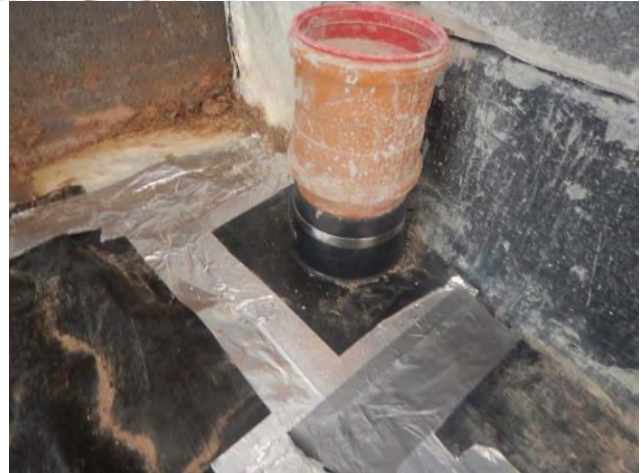
Photograph 20: Showing the typical installation of a preformed tophat using a jubilee clip, butyl and silver joining tape on Plot 4 during inspection on 14 th August 2017.
