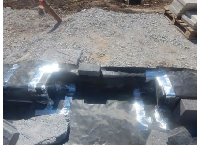
Photograph 2: Showing the first stage of membrane construction on top of the cavity wall, with corners showing sufficient seal and overlap and the general condition of the membrane installation on Plots 7-10 during inspection on 4 th May 2017.
