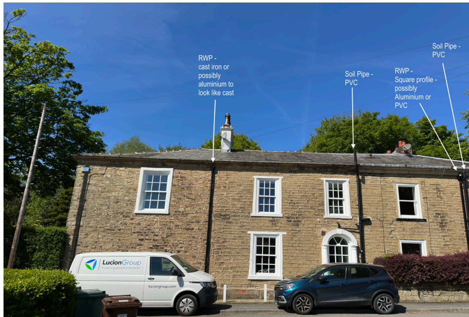
Figure 3: Photograph of the existing condition labelled to show pipework use and material.
