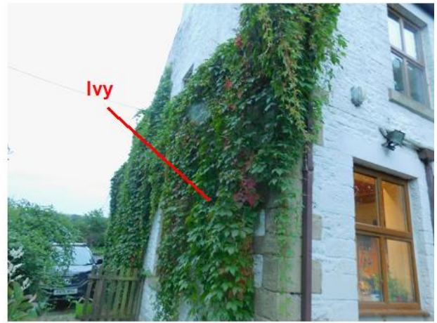
PHOTO 10 North-eastern Corner of House
