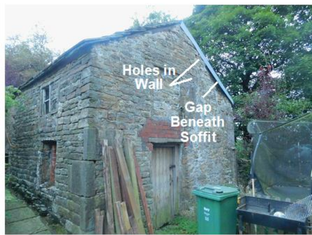
PHOTO 16 South-eastern Corner of Barn
