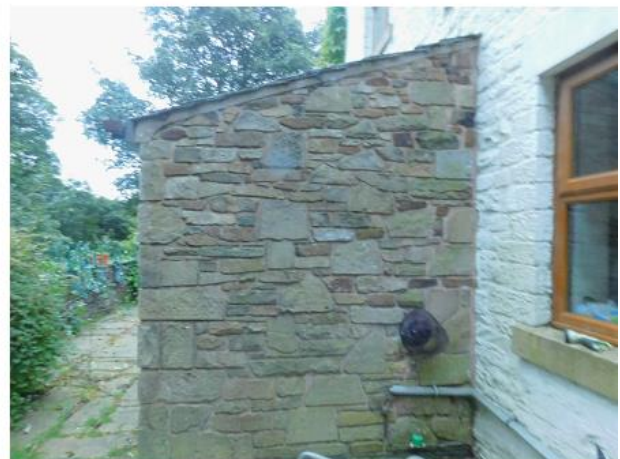
PHOTO 6 North-western Corner of Kitchen Extension
