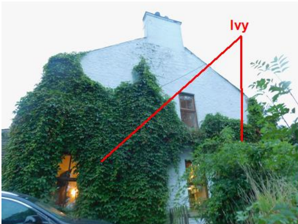
PHOTO 11 Eastern Elevation of House
