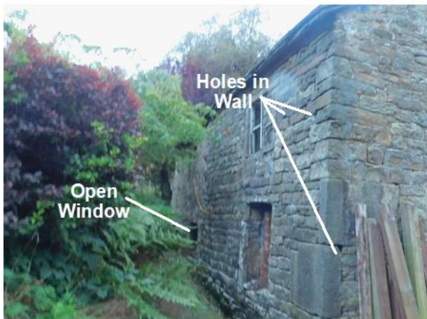
PHOTO 17 Southern Elevation of Barn
