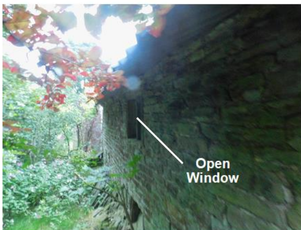
PHOTO 21 View along Northern Elevation of Barn
