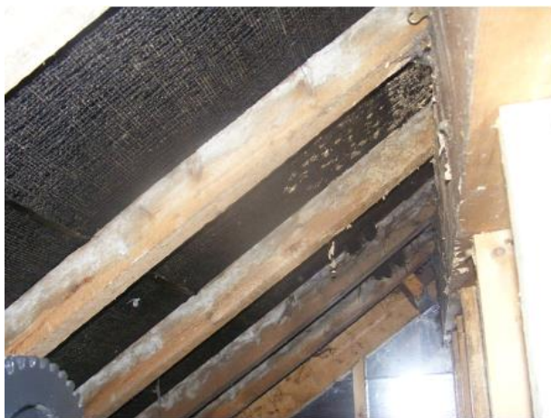
PHOTO 13 Underside of Southern Roof
