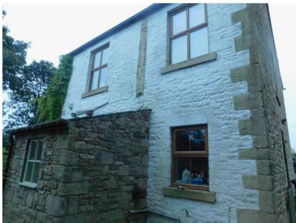
PHOTO 5 Western Elevation of House
