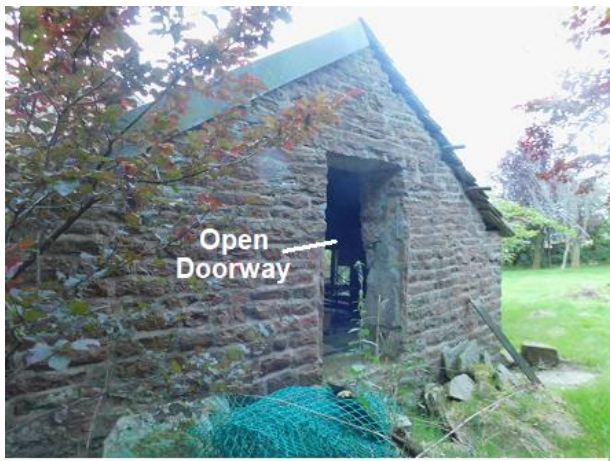
PHOTO 19 Western Elevation of Barn
