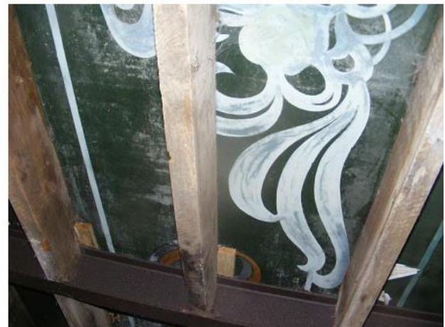
PHOTO 24 Underside of Cellar Roof
