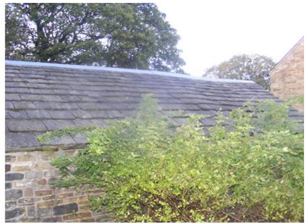
PHOTO 20 Northern Elevation of Barn
