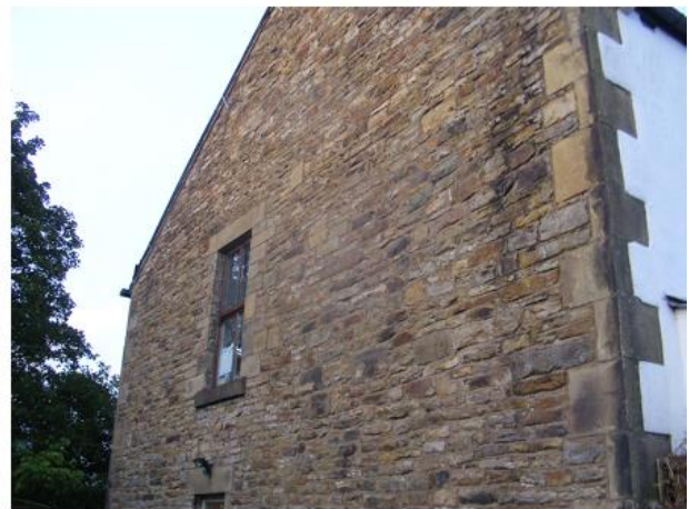
PHOTO 4 Western Elevation of House
