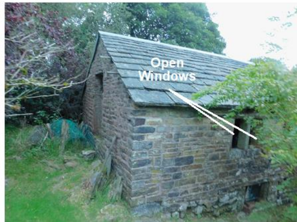
PHOTO 18 South-western Corner of Barn
