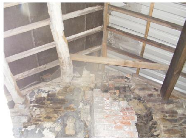
PHOTO 22 Underside of Eastern Roof of Barn
