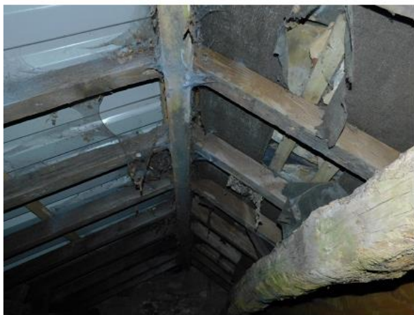
PHOTO 23 Underside of Western Roof of Barn
