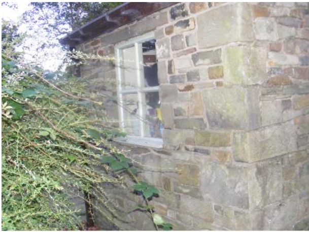
PHOTO 7 Northern Elevation of Kitchen Extension
