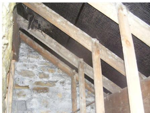
PHOTO 14 Underside of Northern Roof
