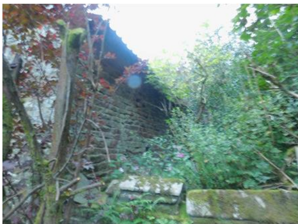
PHOTO 15 North-eastern Corner of Barn
