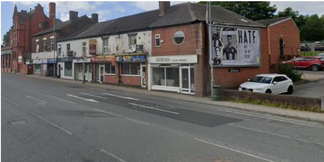
Advertisement hoarding on the gable of 251 Bury New Road
