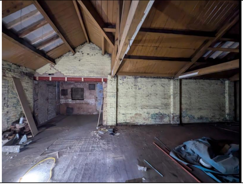
Photo 7. View of timber clad section of roof from upper floor.
