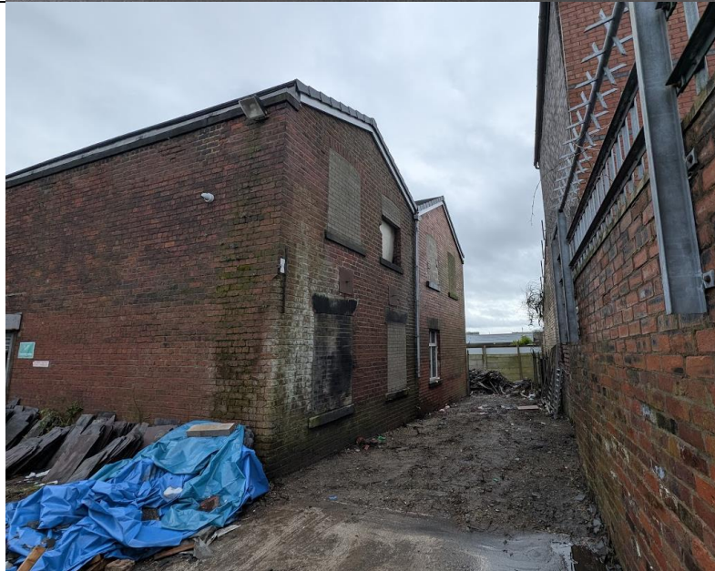
Photo 2. Section of rear (north) elevation.
