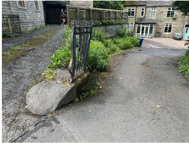
Condition of fence and concrete to LHS at entrance
