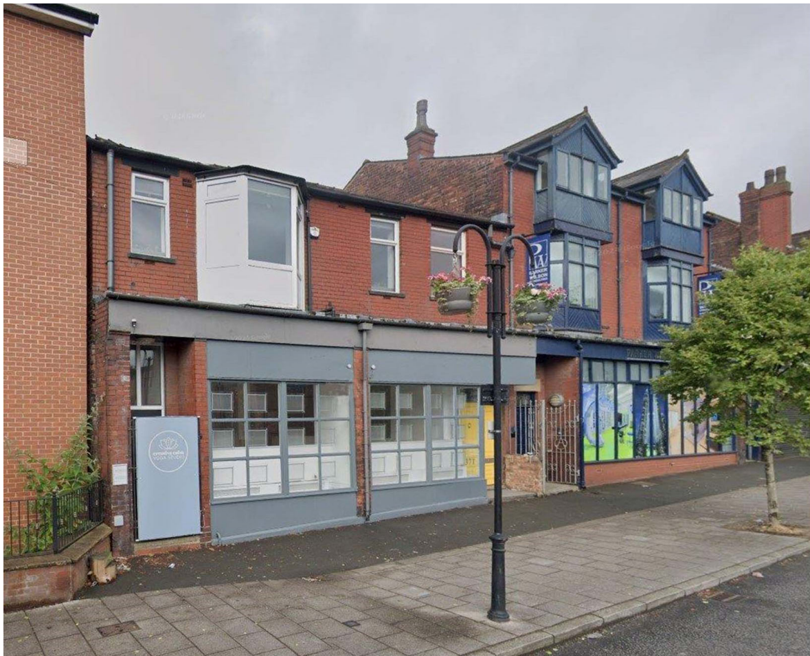
Frontage of Number 371 on to Bury New Road with Number 373 to the right – Number 373's frontage was restored nearly twenty years ago through funding made available from the Council/ English Heritage jointly funded Heritage Economic Regeneration Scheme
