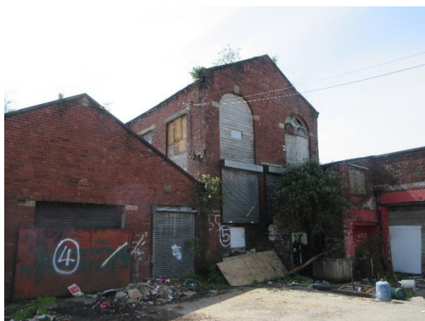
Photo 7: Northern elevations of B2 (right) and B3 (left)
