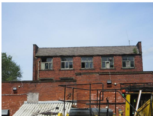
Photo 13: Southern elevation and roof of B6
