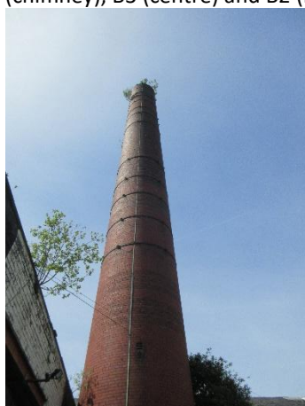
Photo 11: Building B4 (chimney)
