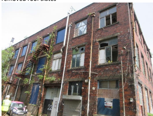
Photo 17: Western and southern elevations of B6
