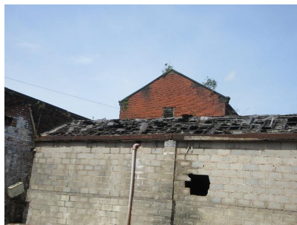
Photo 8: Southern elevation of B2 and sections of B7 with removed roof slates
