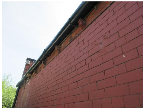
Photo 2: Sealed timber fascia at northern elevation of B1
