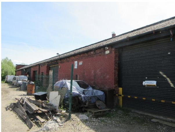
Photo 1: Northern elevation of B1
