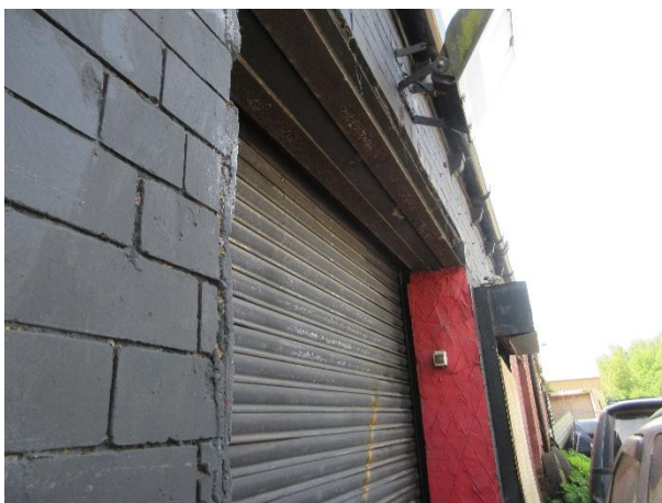
Photo 3: No gaps / potential roost features (PRFs) at doorway apertures at B1
