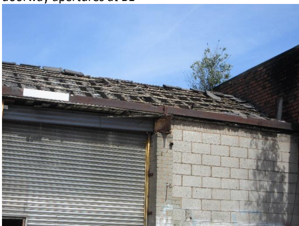
Photo 5: Sealed concrete blockwork and removed slates on roof at B1
