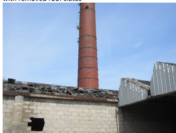
Photo 10: B4 (chimney) and sections of B7 with removed roof slates
