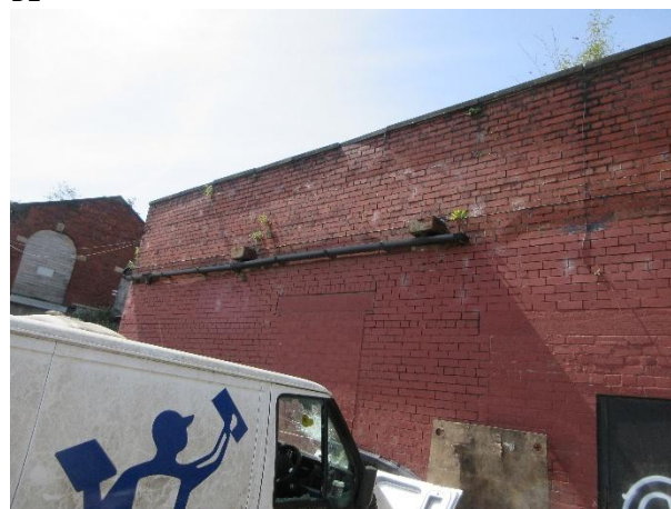
Photo 4: Sealed brickwork at B1
