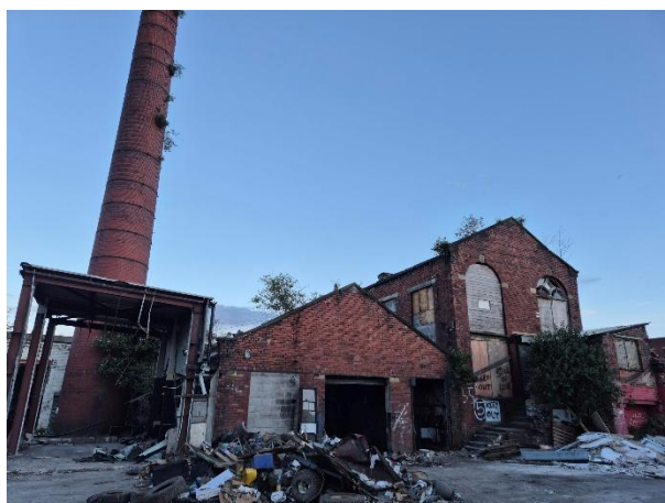
Photo 9: Northern elevations of B5 (left), B4 (chimney), B3 (centre) and B2 (right)
