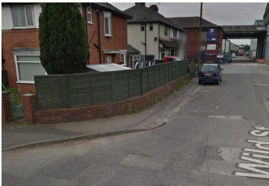
Fig 4: Southern edge of Wild Street with demarked pedestrian route but now kerb upstand to differentiate for vehicles
