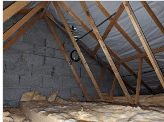
Figure 14: Internal roof void
