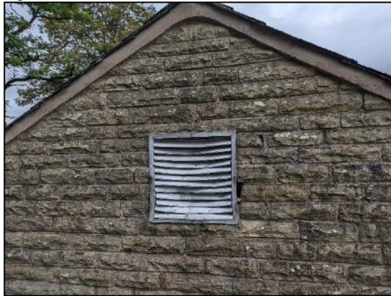
Figure 13: vent on western gable
