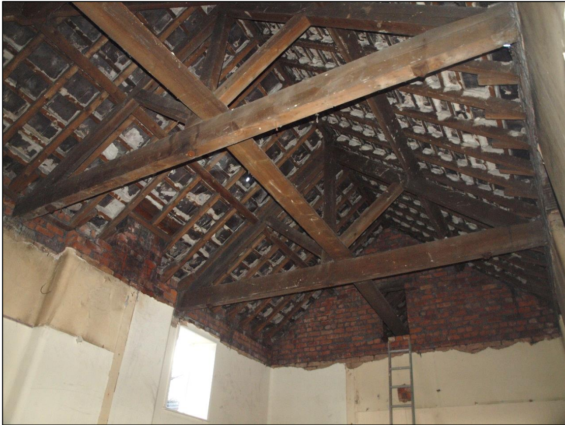
Plate 19: Shot showing roof structure
