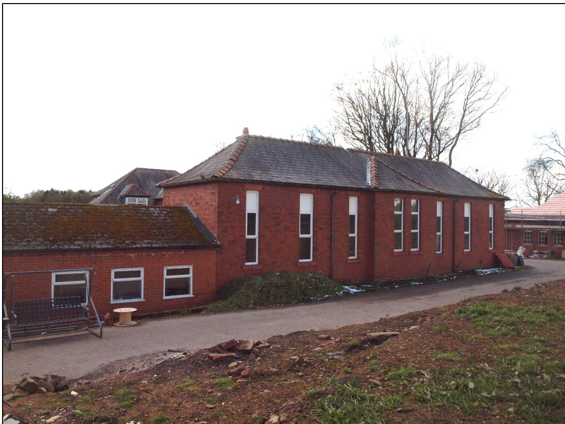
Plate 6: General shot of north elevation
