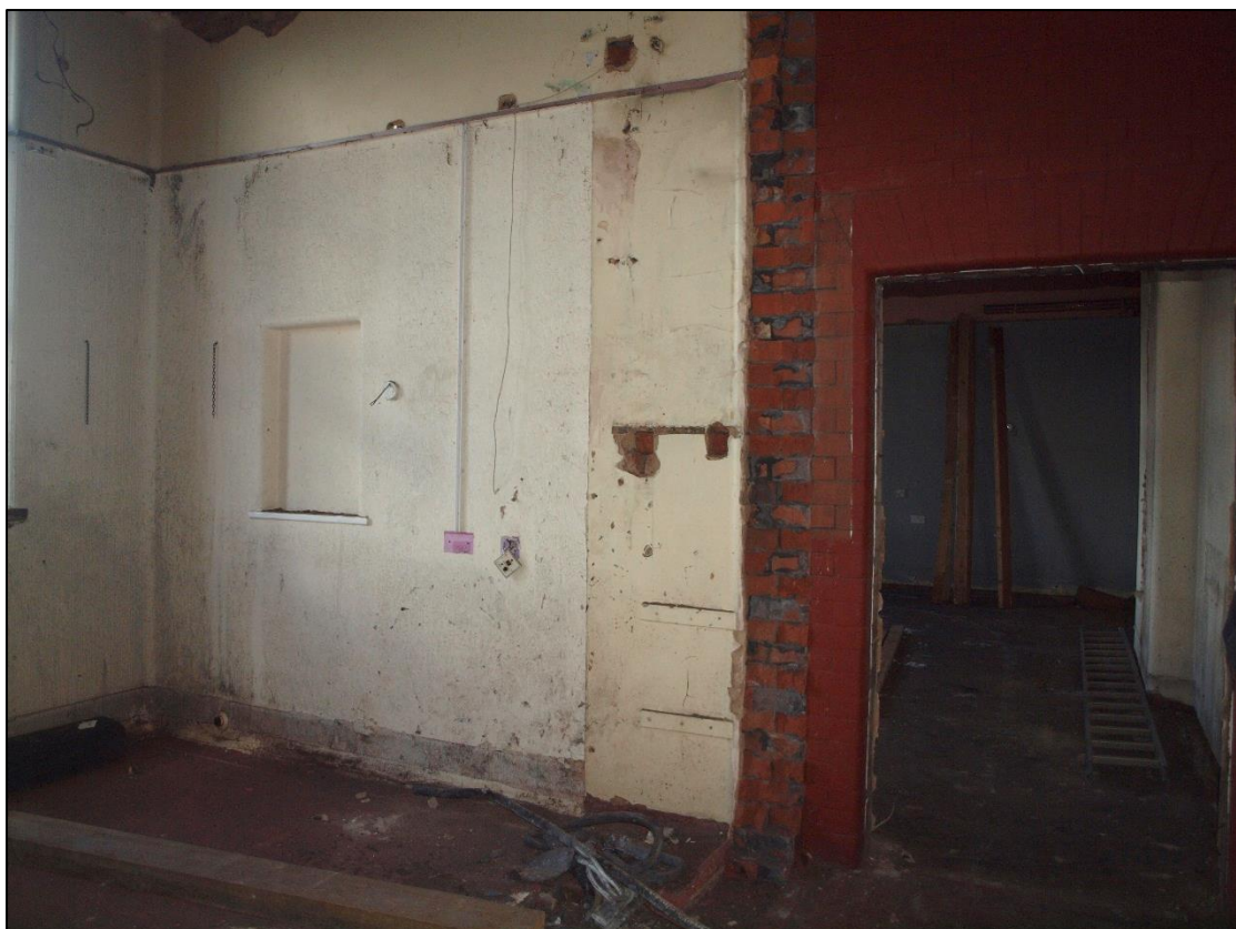
Plate 14: Nurses station opposite entrance showing hatch and doorway to east ward
