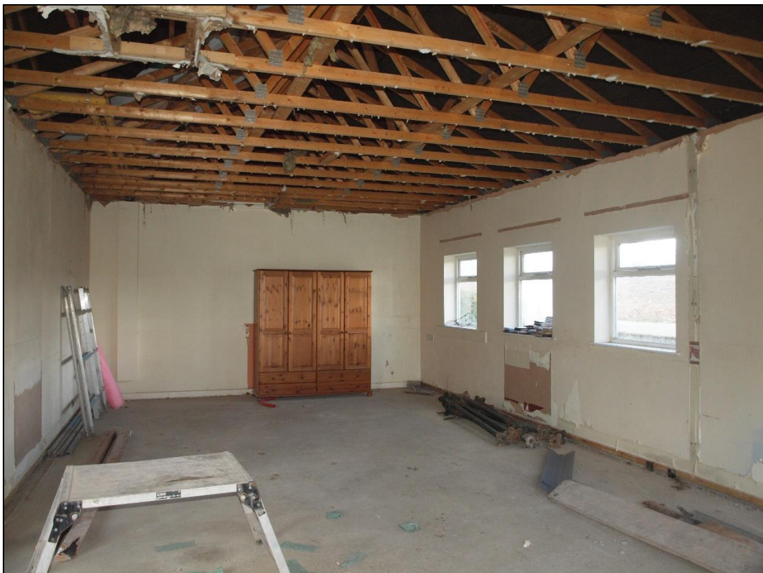
Plate 22: Room at north end of modern extension, looking west
