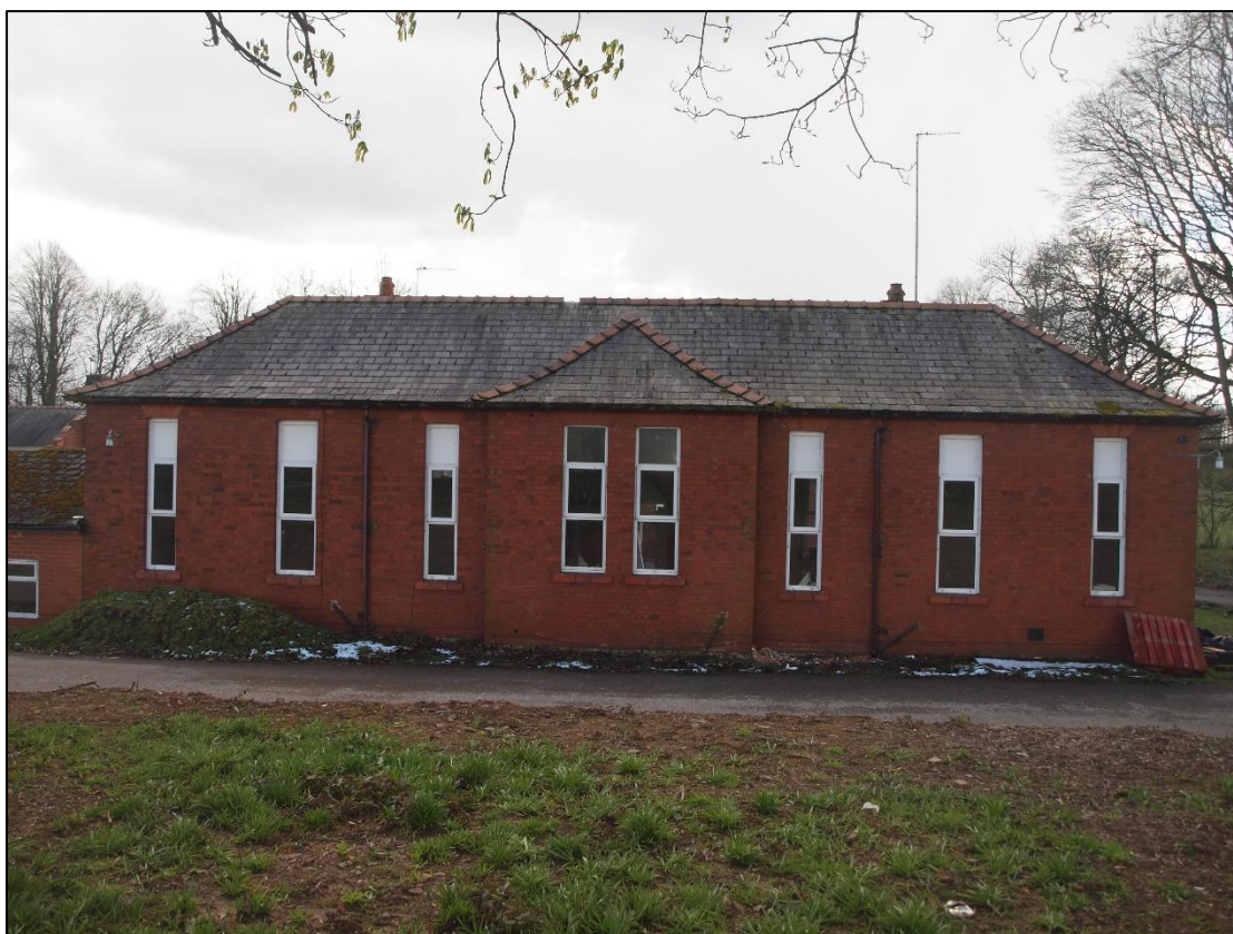
Plate 7: North elevation of main building showing inserted windows
