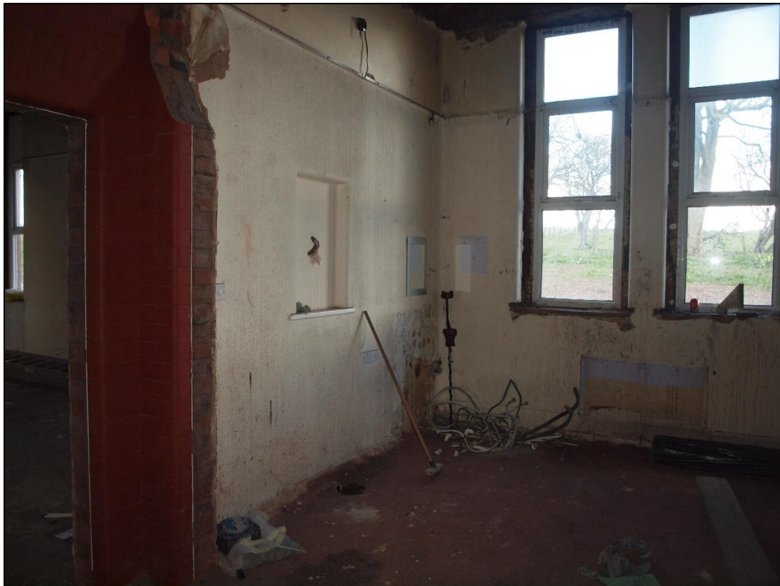
Plate 13: Nurses station opposite entrance showing hatch to west ward
