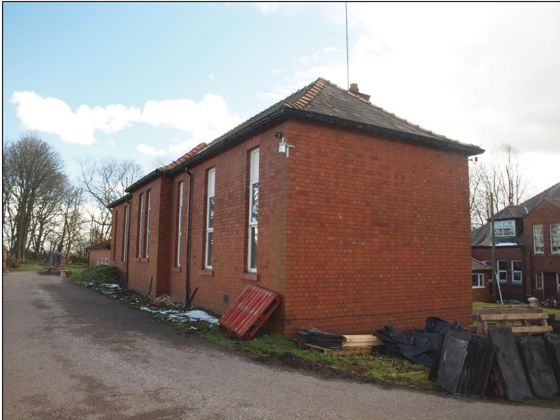
Plate 5: West elevation of main building
