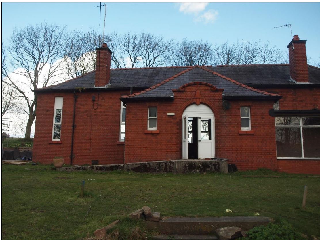
Plate 2: South elevation showing west side and central entrance
