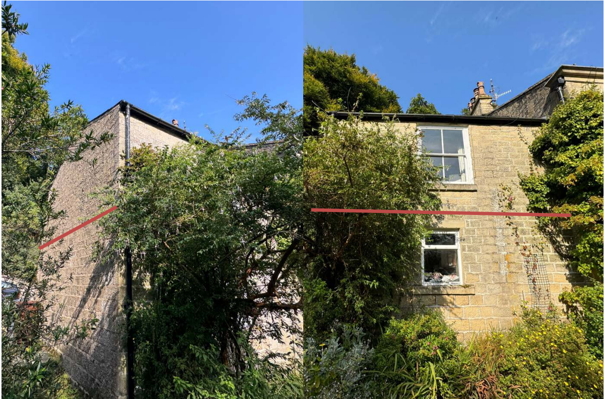
Figures 15 and 16 – Red line shows the top edge of the wall to be removed.
