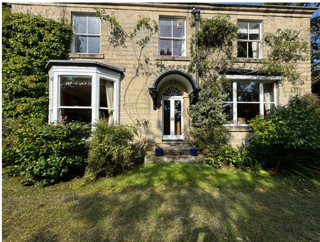
Figure 9 – End of C19th alterations to include bay and lead roof canopy.
