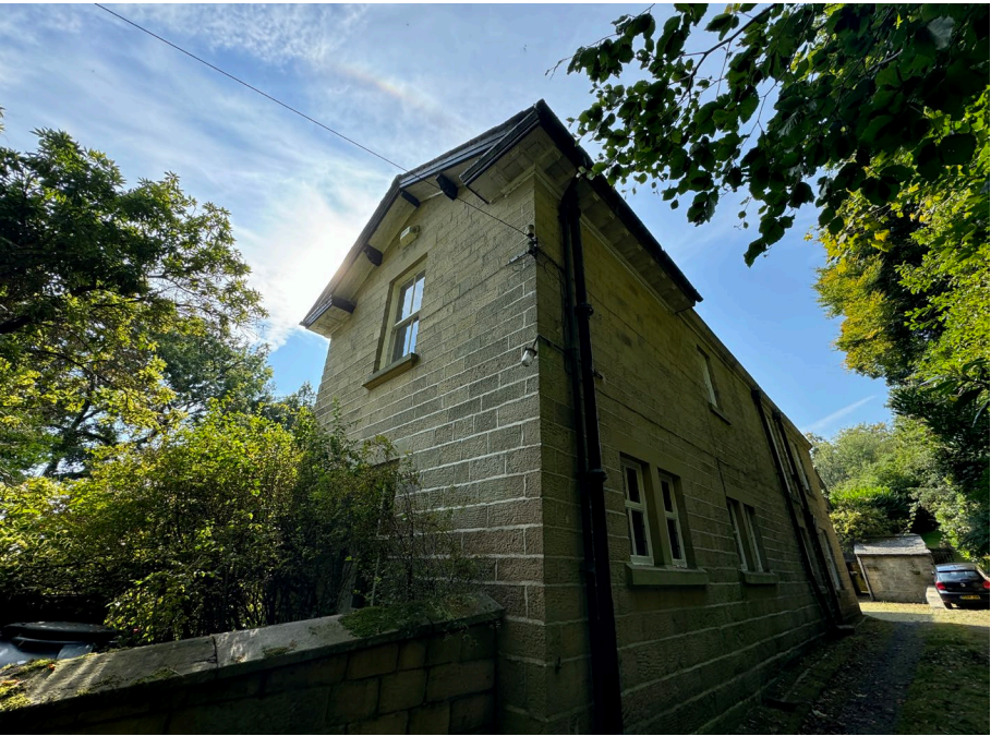
Existing North East corner of Woodside on approach from access drive
