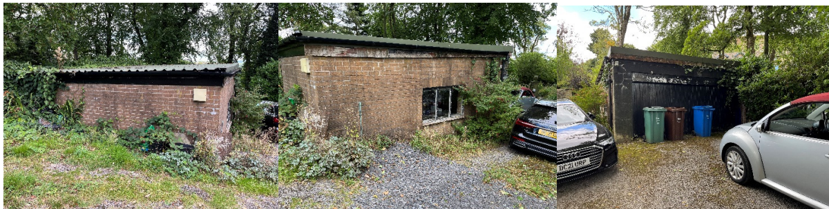
Existing Garage Rear Elevation
