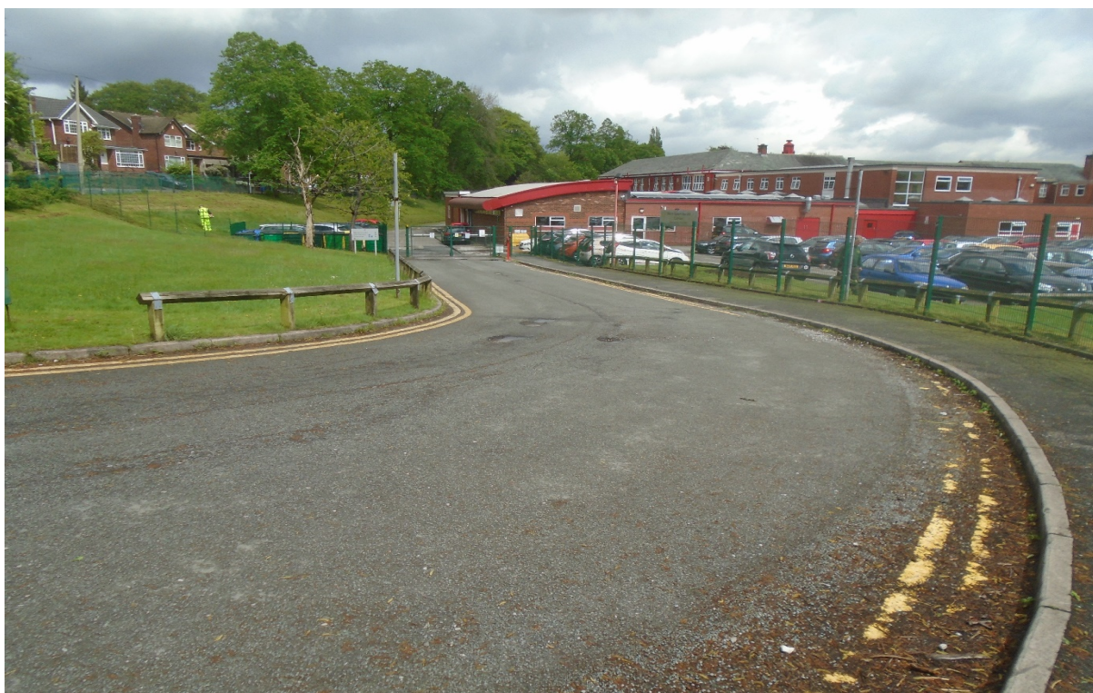
PHOTO 6 : Showing the entrance road onto site currently two way for traffic but will become one way ( inwards ) on the new proposal with the new car park exit to the lower top right of the photo.
