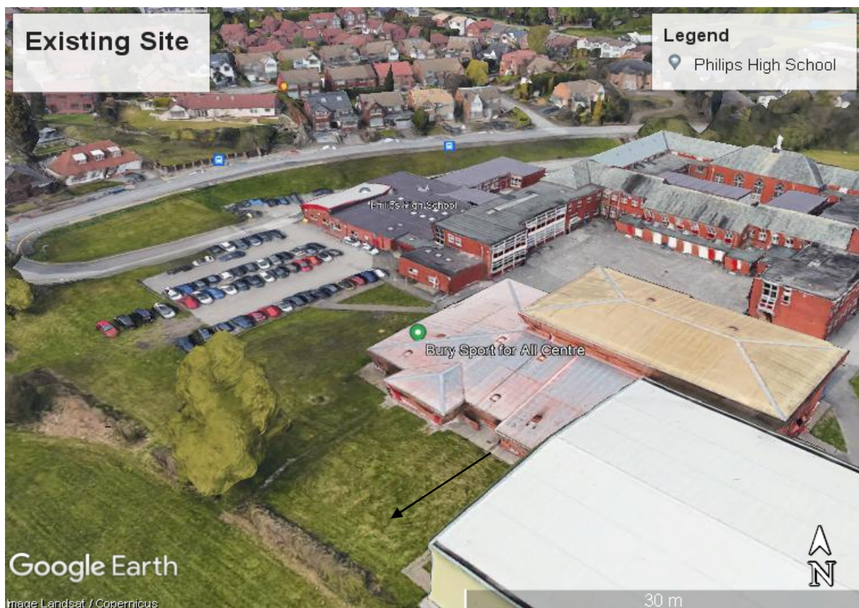
PHOTO 9 : Showing existing car park and how staff because of capacity issues have started to park on the grassed area beyond the hardstanding designated parking area. How far the previous Ball Hall has extended into the green belt strip between the school sports hall and school sports field can be seen by the arrow.
