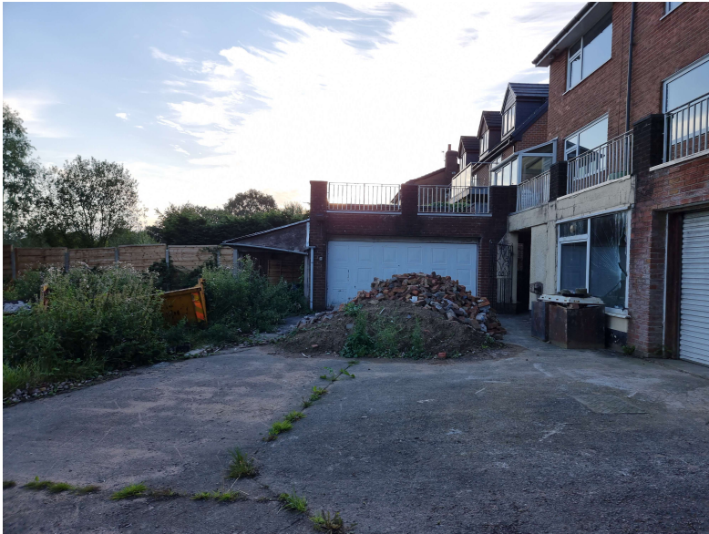
Existing concrete paved area to rear
