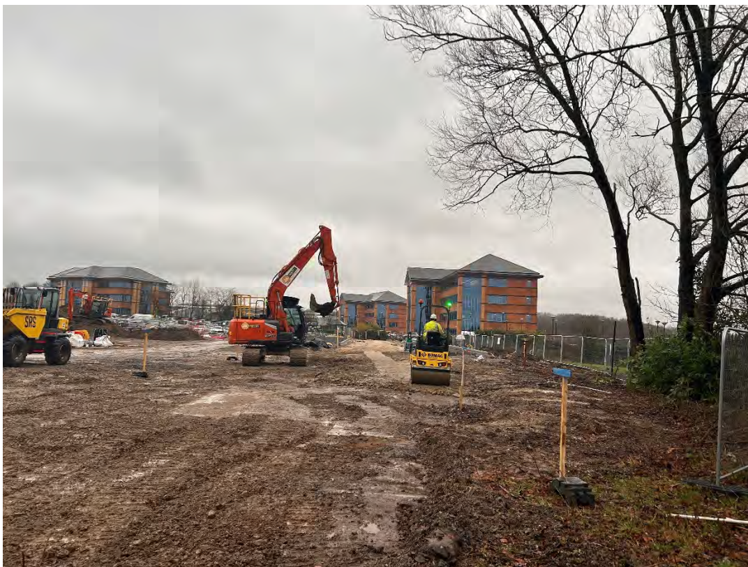
Photograph 3 – Compaction of Formation Level
