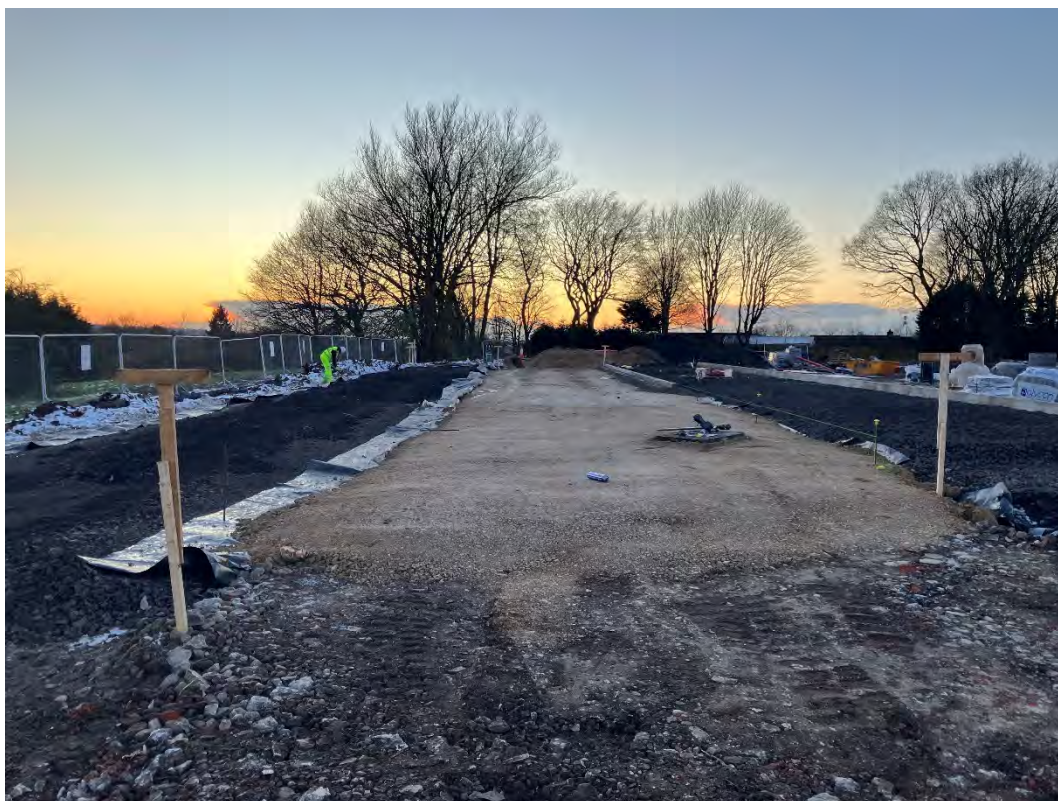
Photograph 4 – Forming of Roads
