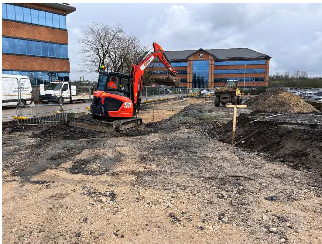
Photograph 2 – Cut to Formation
