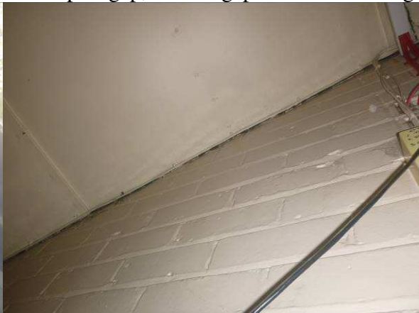
P6 Well-sealed ceiling
