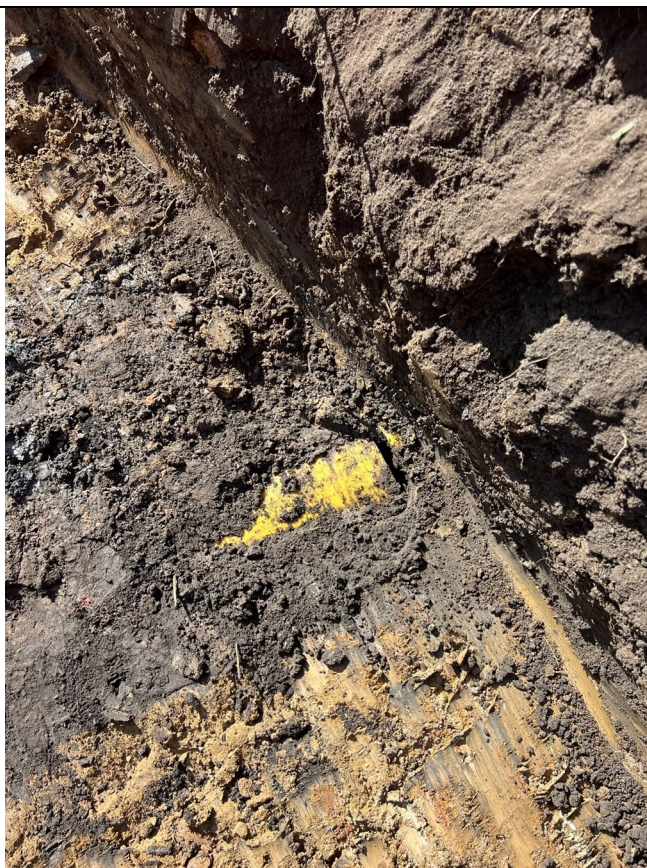
TT07 5-Plastic drain (end visible in slope above stream)
