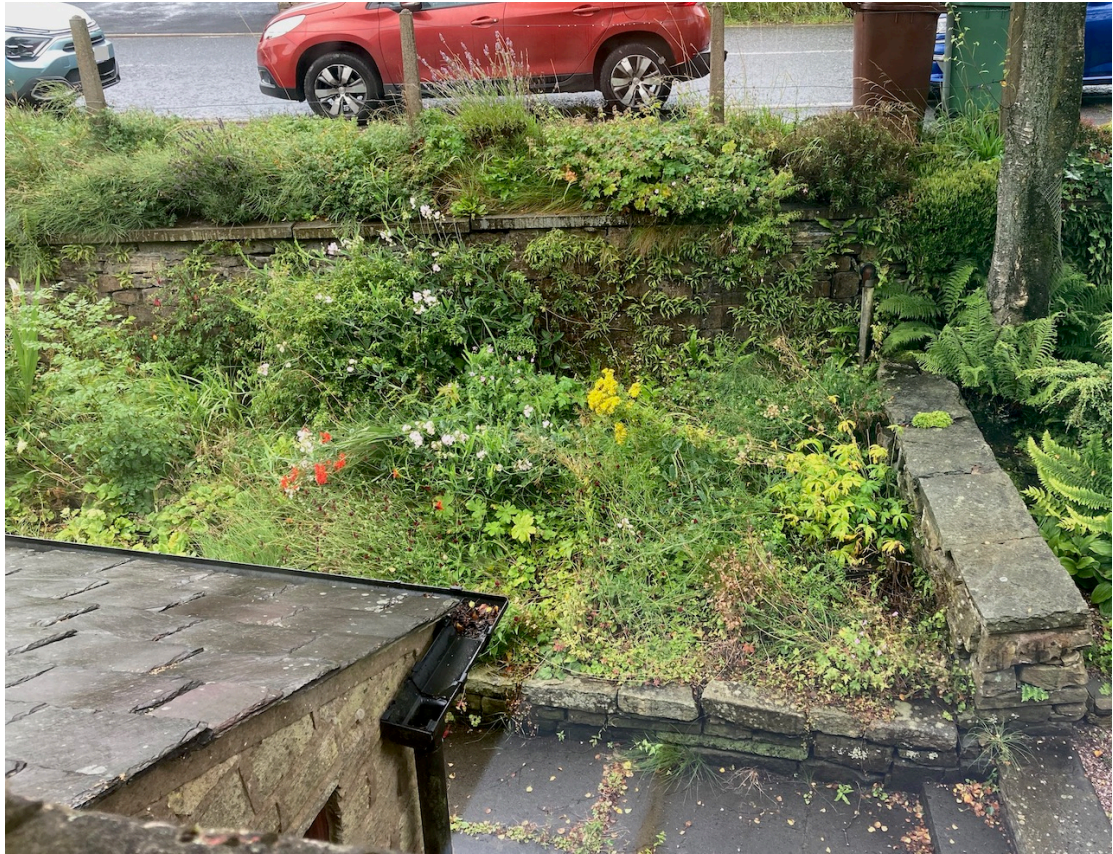
Figure 2: View of the front garden area and retaining wall to the footpath along Turton Road.
